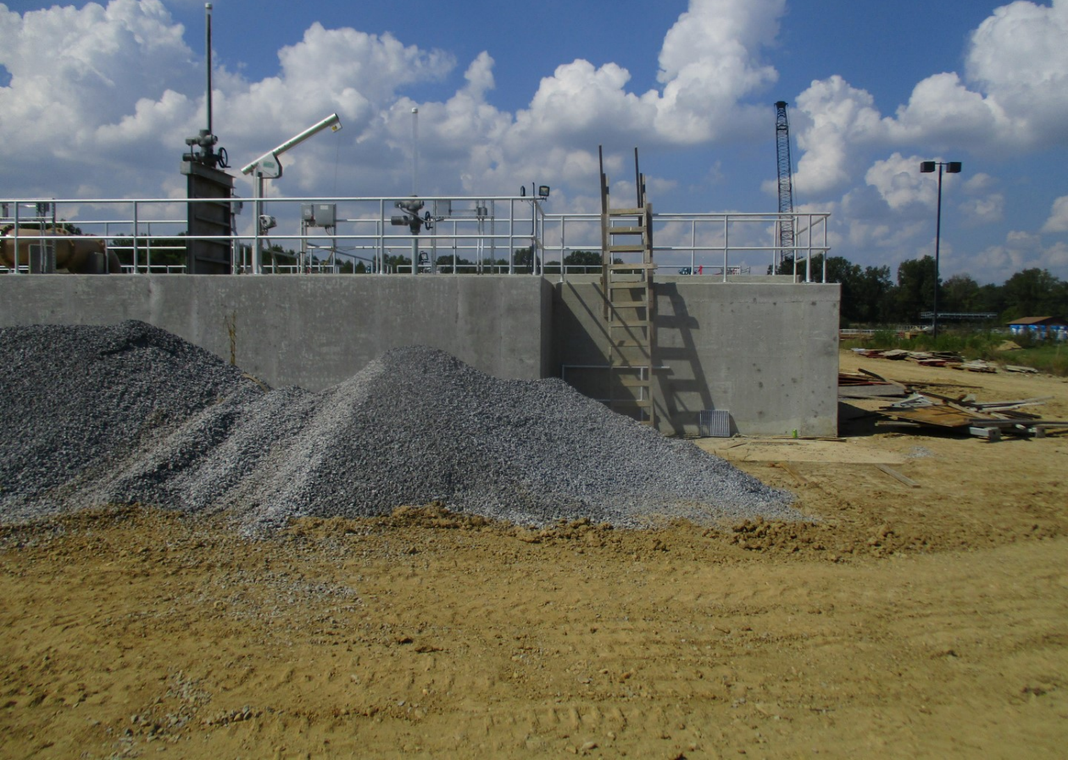
Vertical Loop Reactor - Photo 7
