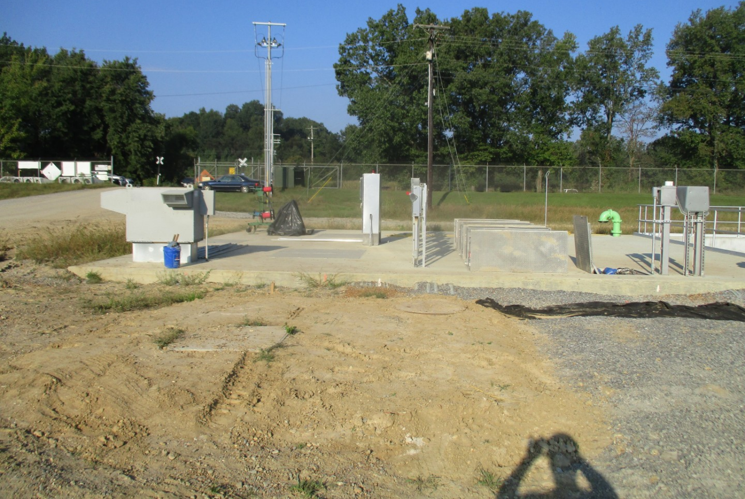
Pretreatment Facilities - Photo 4
