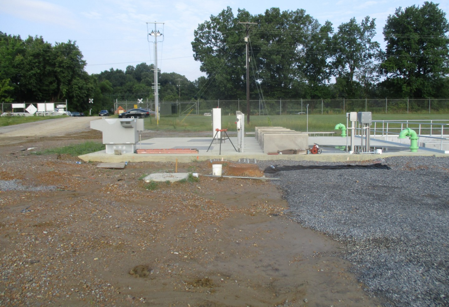
Pretreatment Facilities - Photo 4
