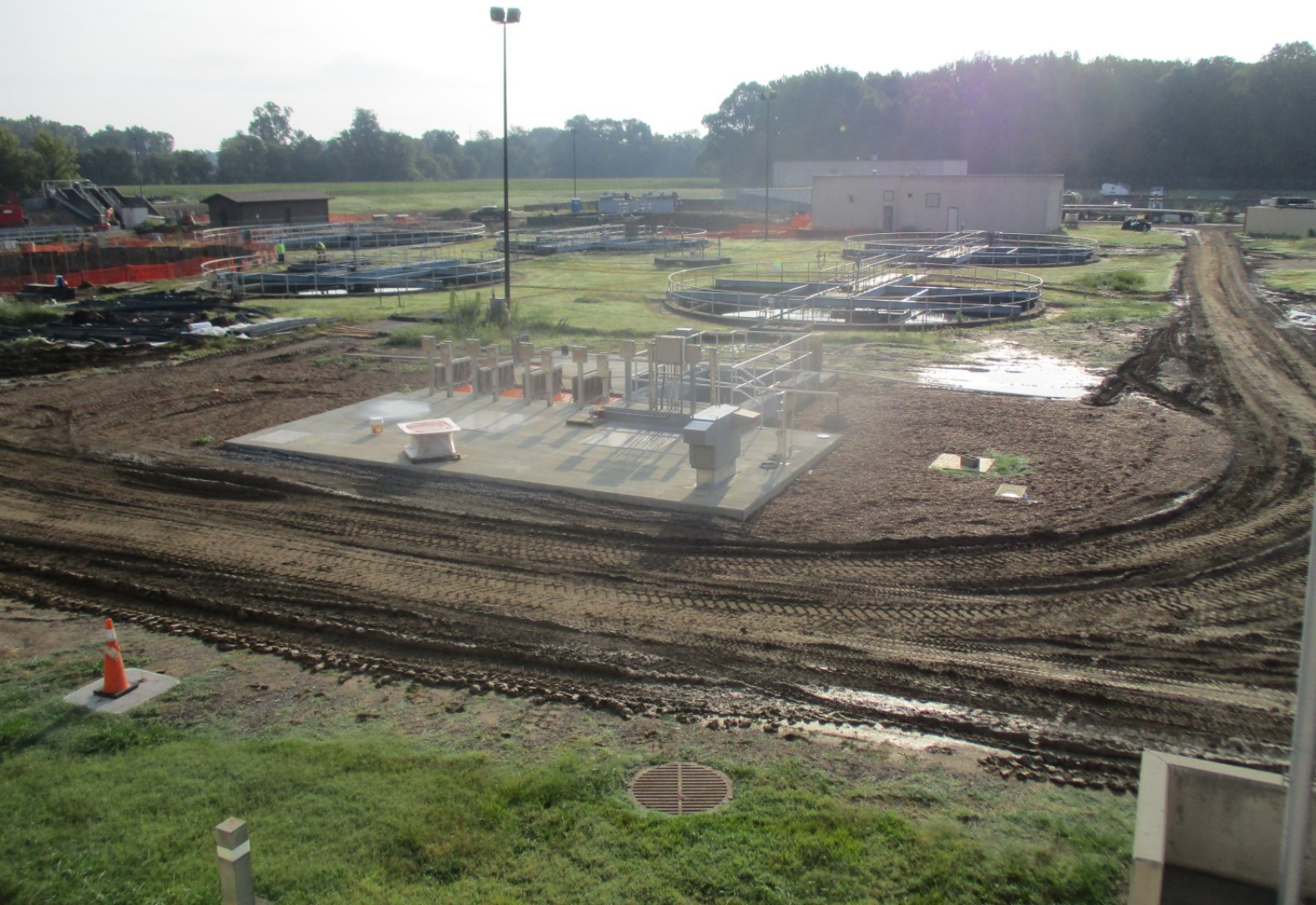
RAS Pump Station - Photo 1
