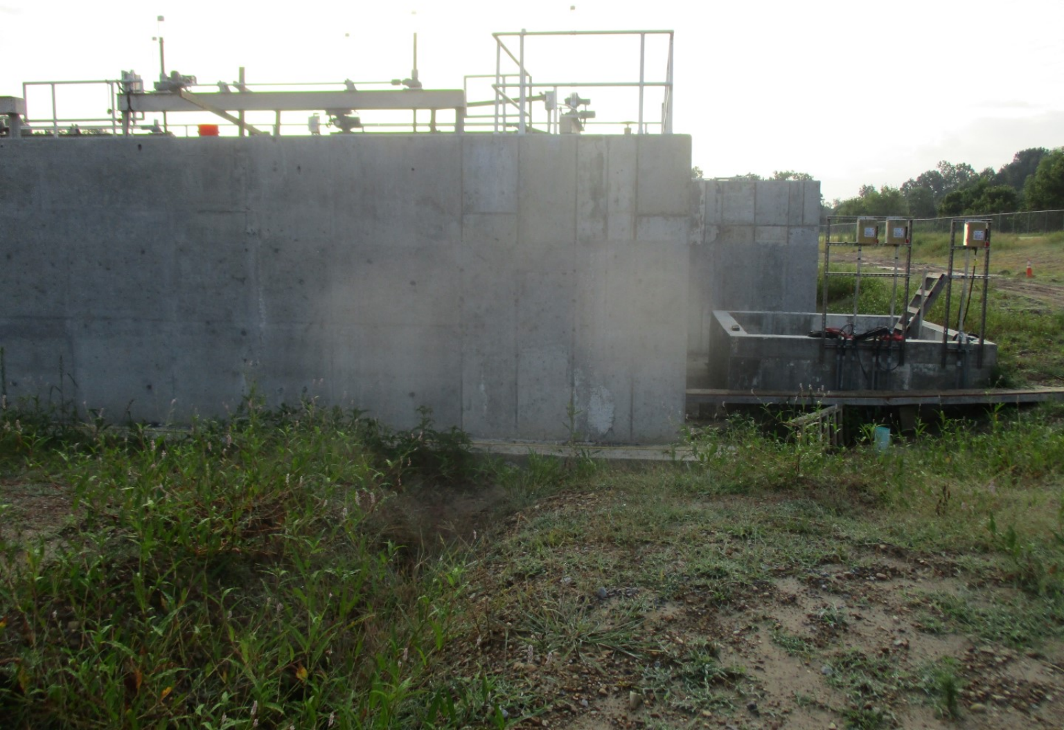
Vertical Loop Reactor - Photo 3
