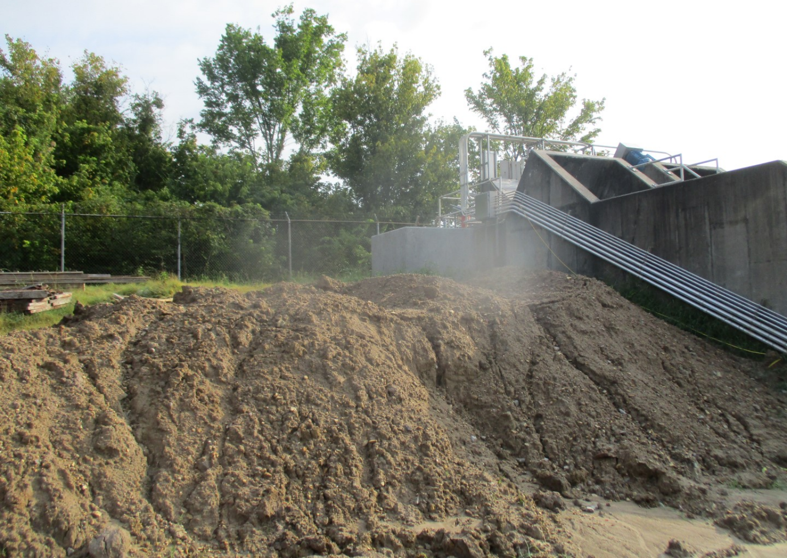
NPW Pump Station Influent - Photo 2
