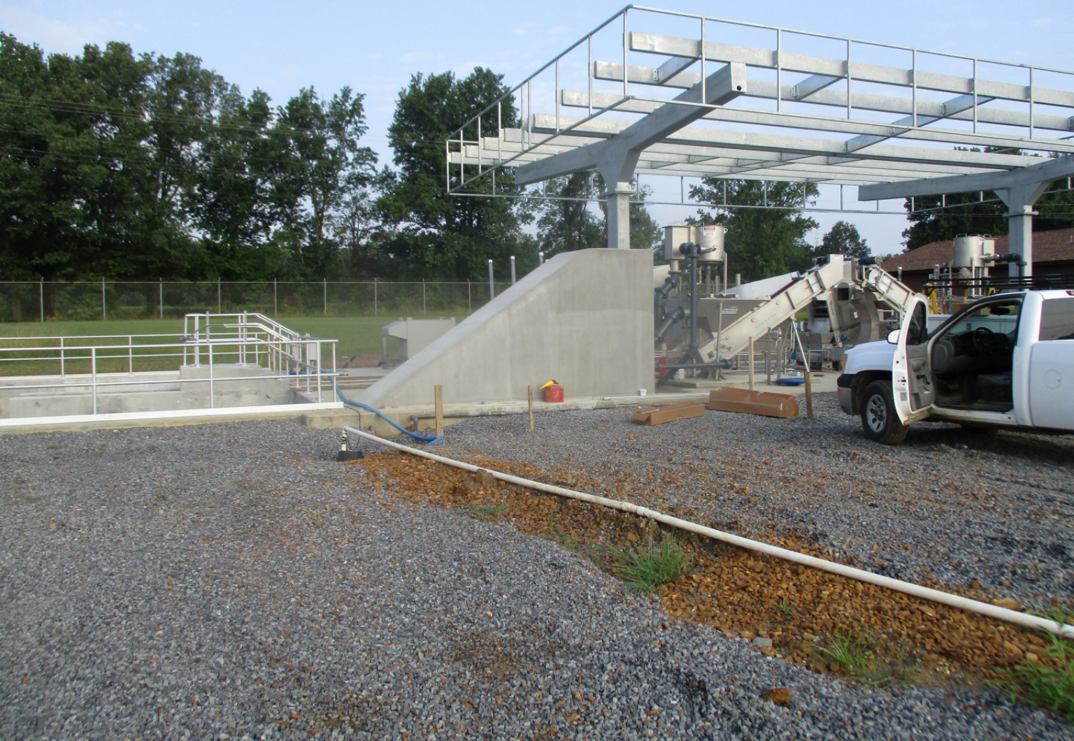
Pretreatment Facilities - Photo 5
