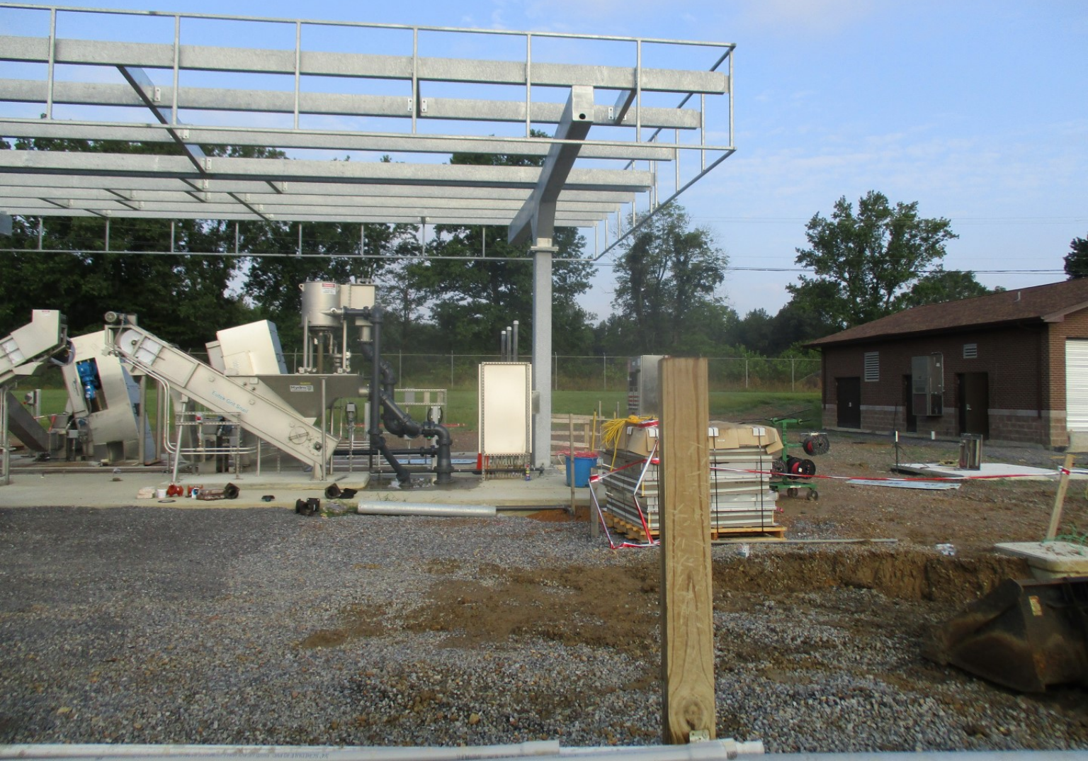
Pretreatment Facilities - Photo 6
