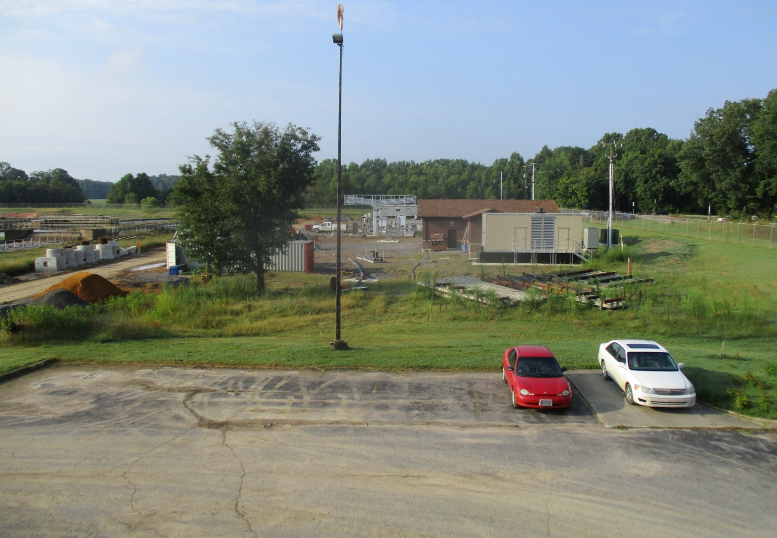
Pretreatment Facilities - Photo 7
