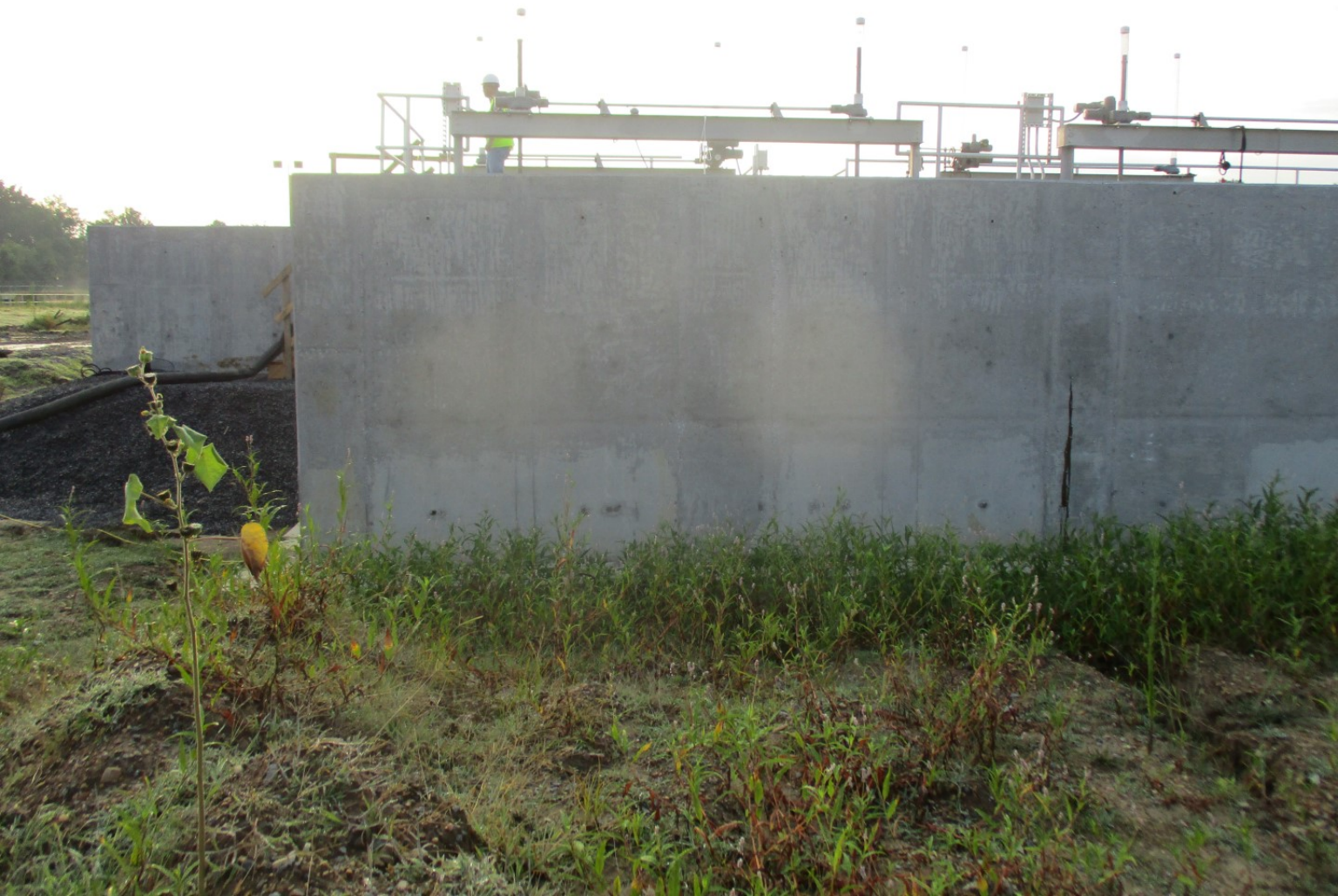
Vertical Loop Reactor - Photo 1
