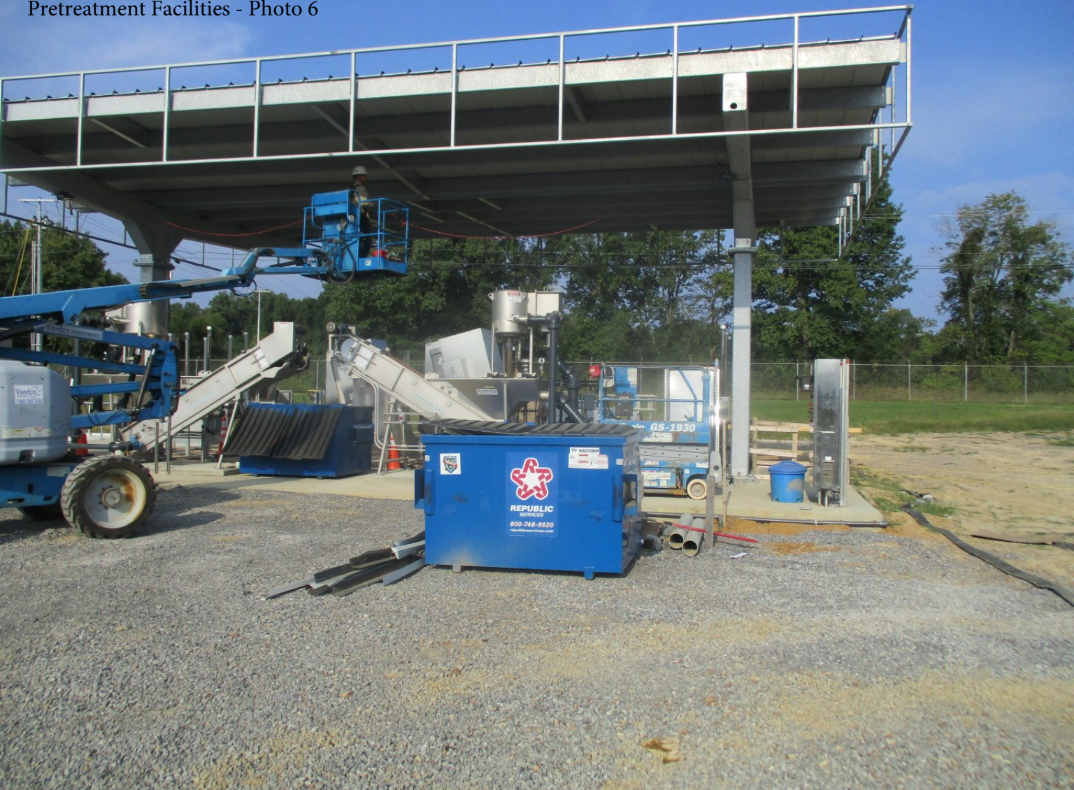
Pretreatment Facilities - Photo 6
