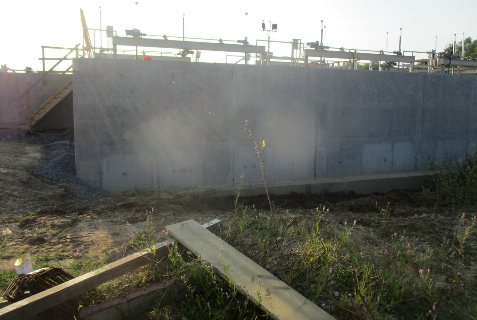
Vertical Loop Reactor - Photo 1
