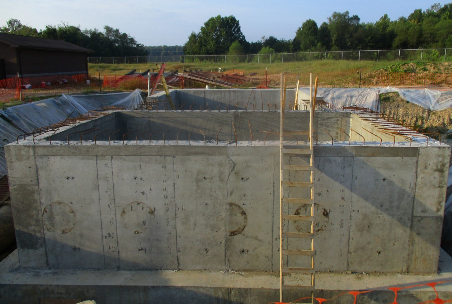
Nitrate Pump Station - Photo 2
