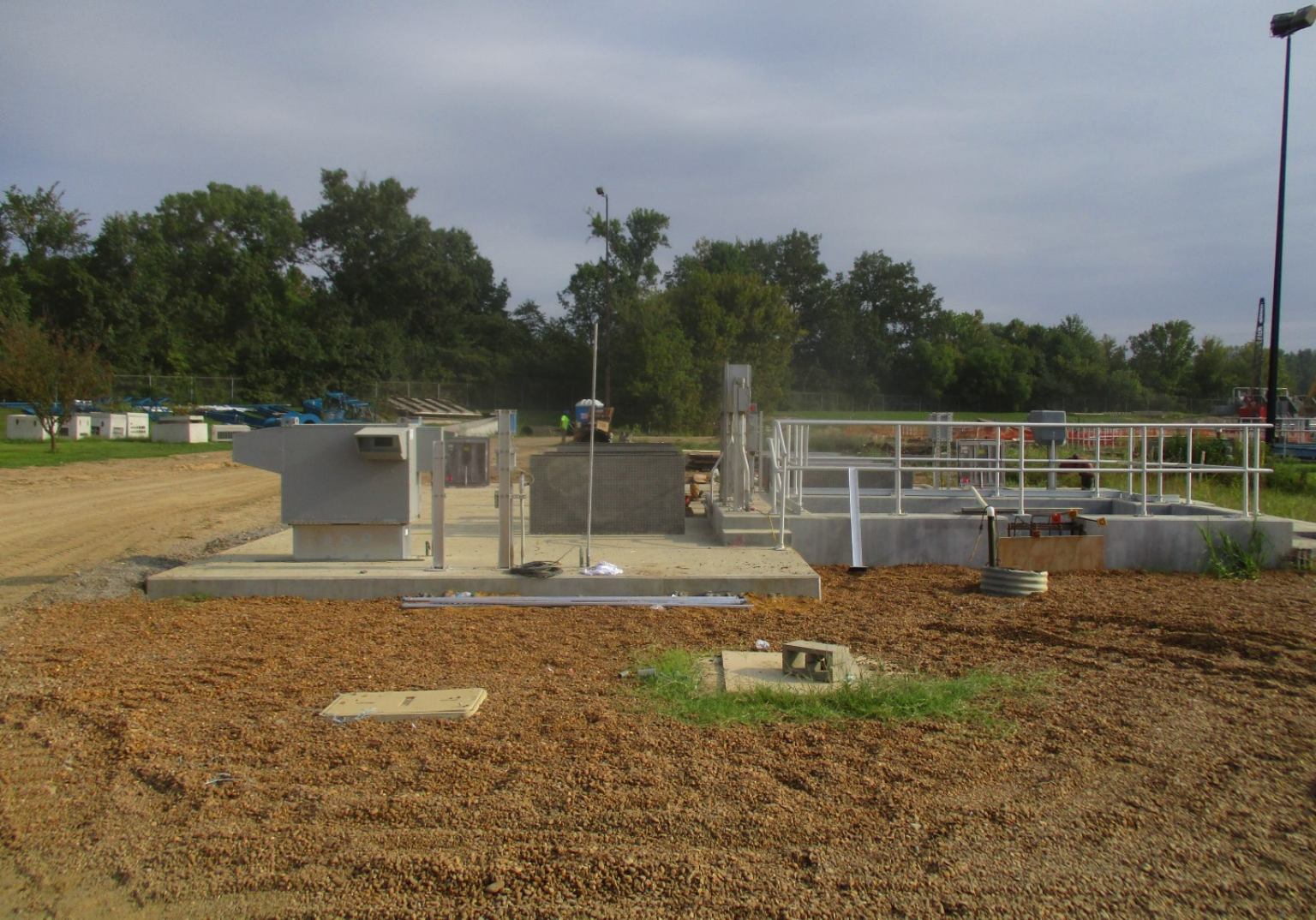
RAS Pump Station - Photo - 2
