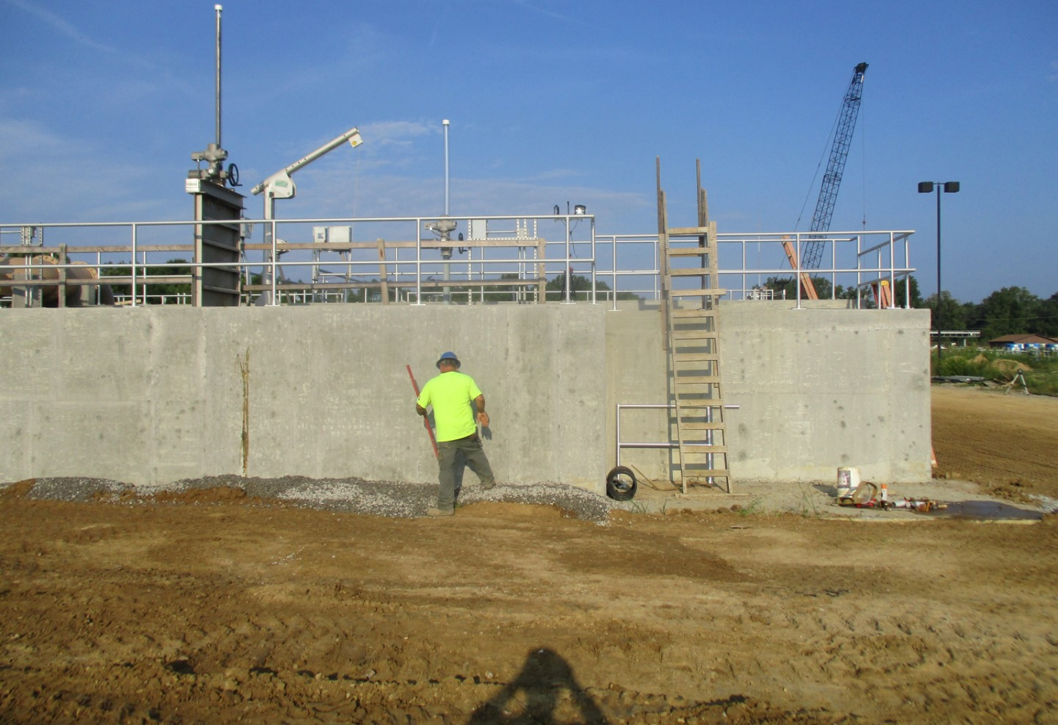
Vertical Loop Reactor - Photo 7
