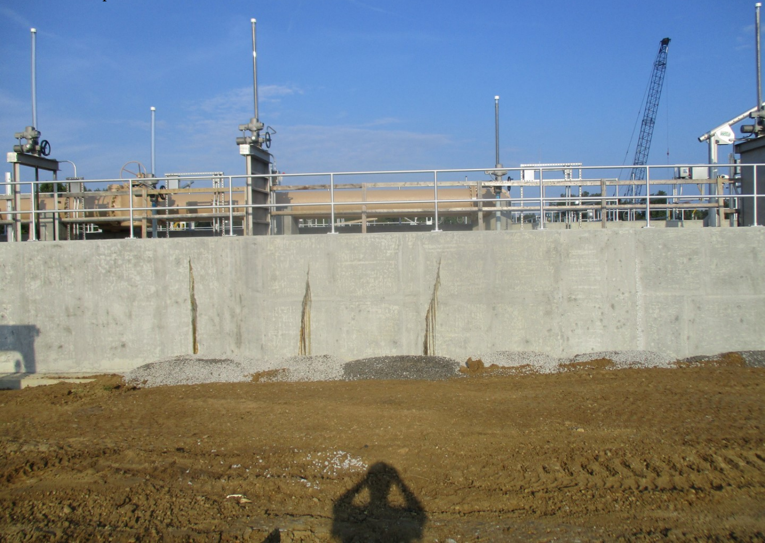
Vertical Loop Reactor - Photo 6
