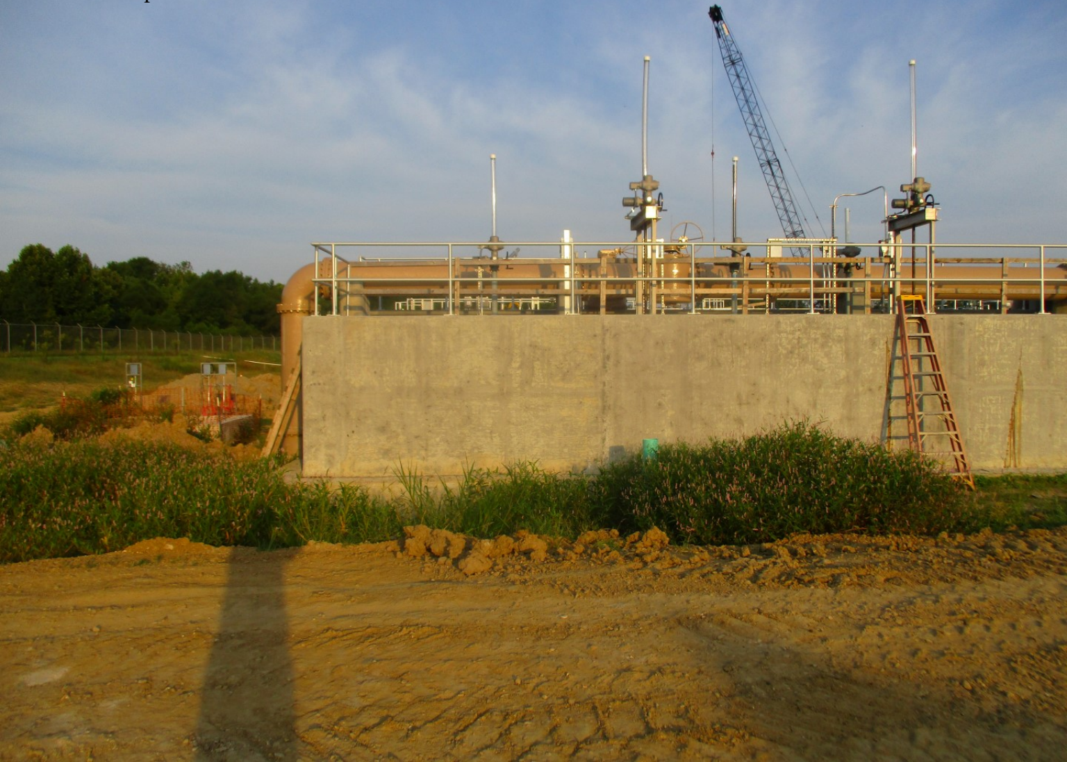
Vertical Loop Reactor - Photo 5
