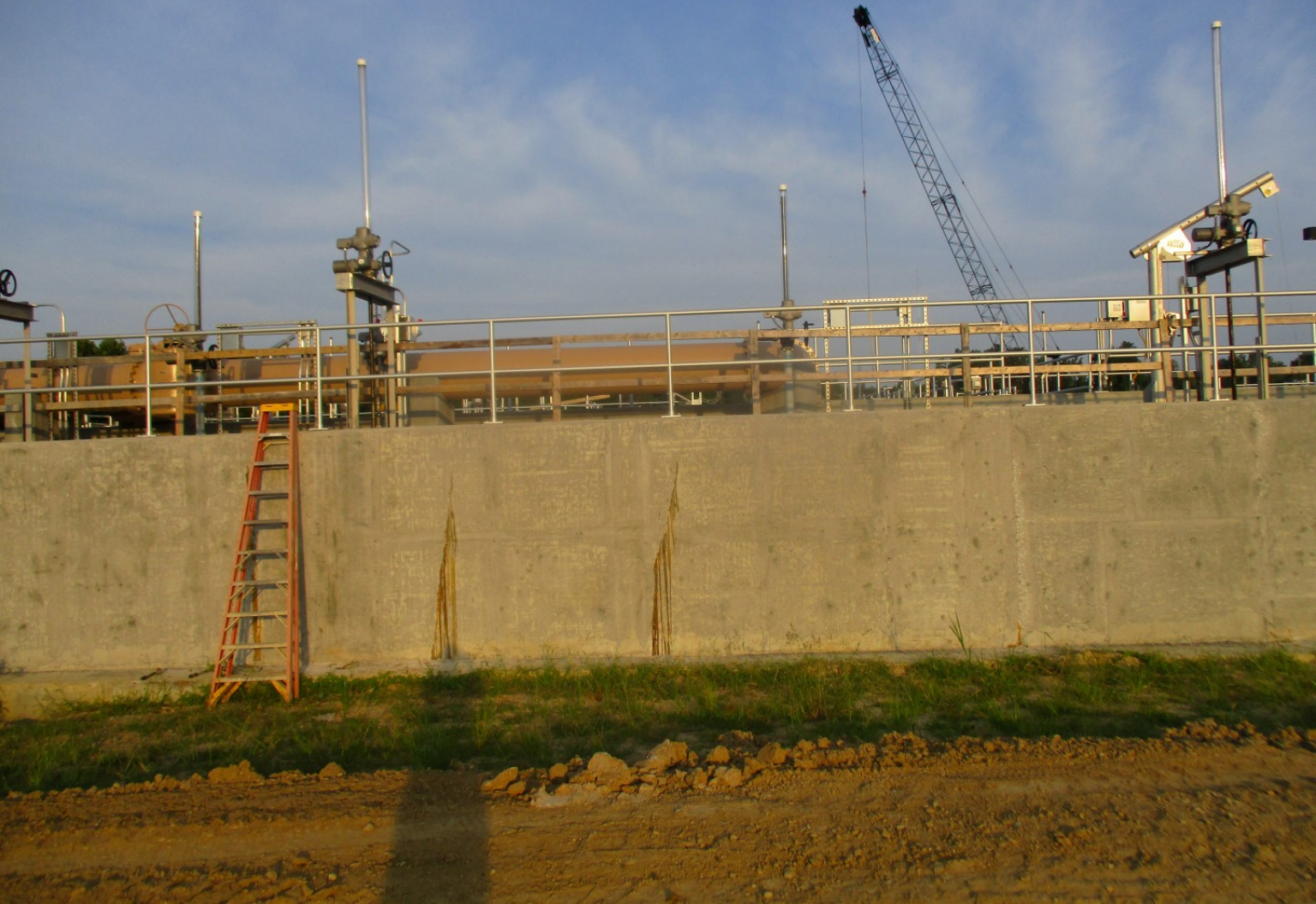
Vertical Loop Reactor - Photo 6
