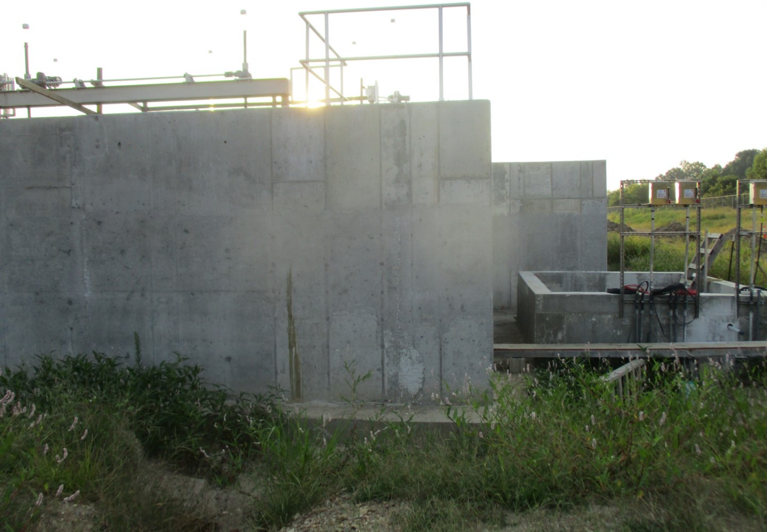
Vertical Loop Reactor - Photo 3
