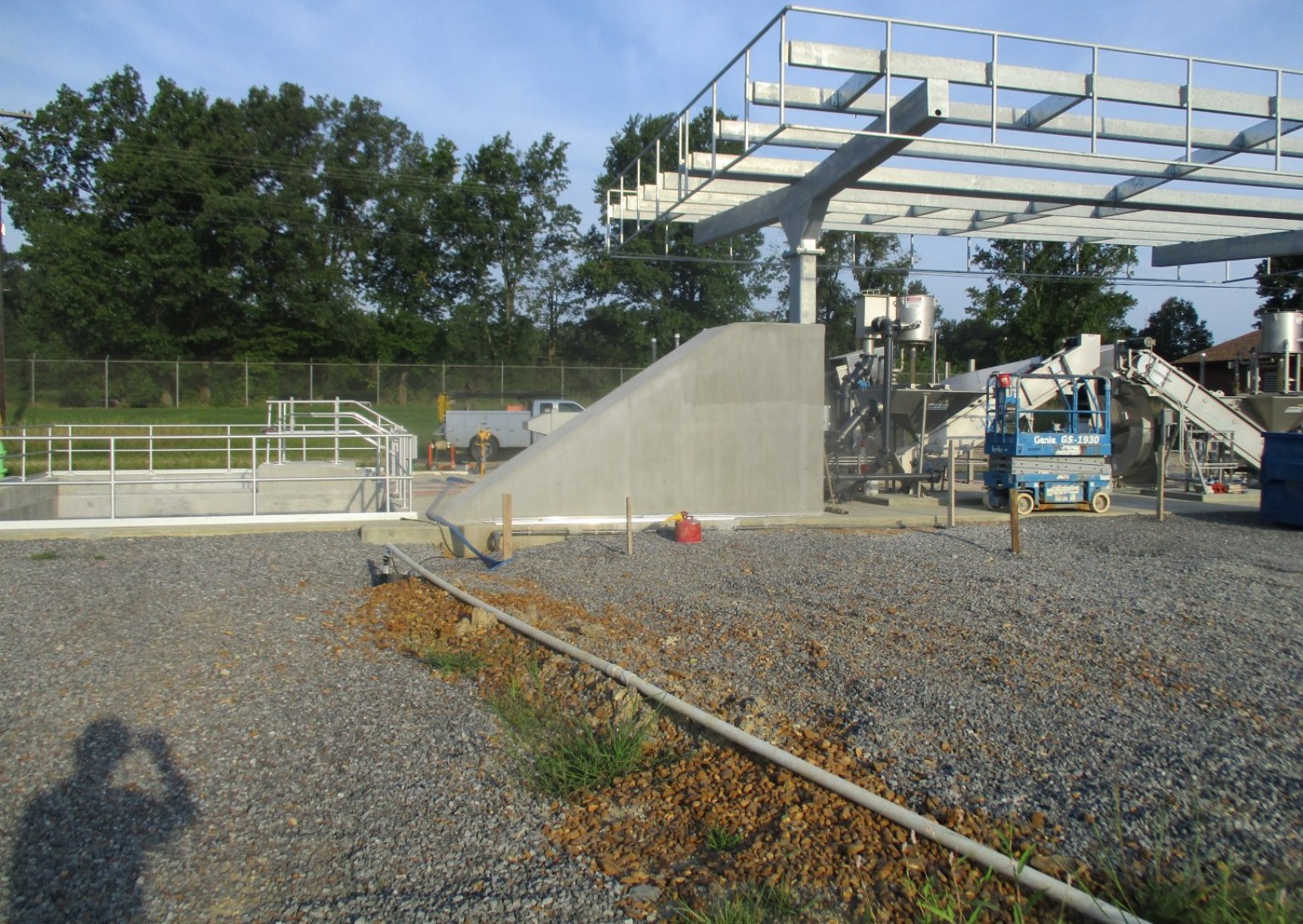
Pretreatment Facilities - Photo 5
