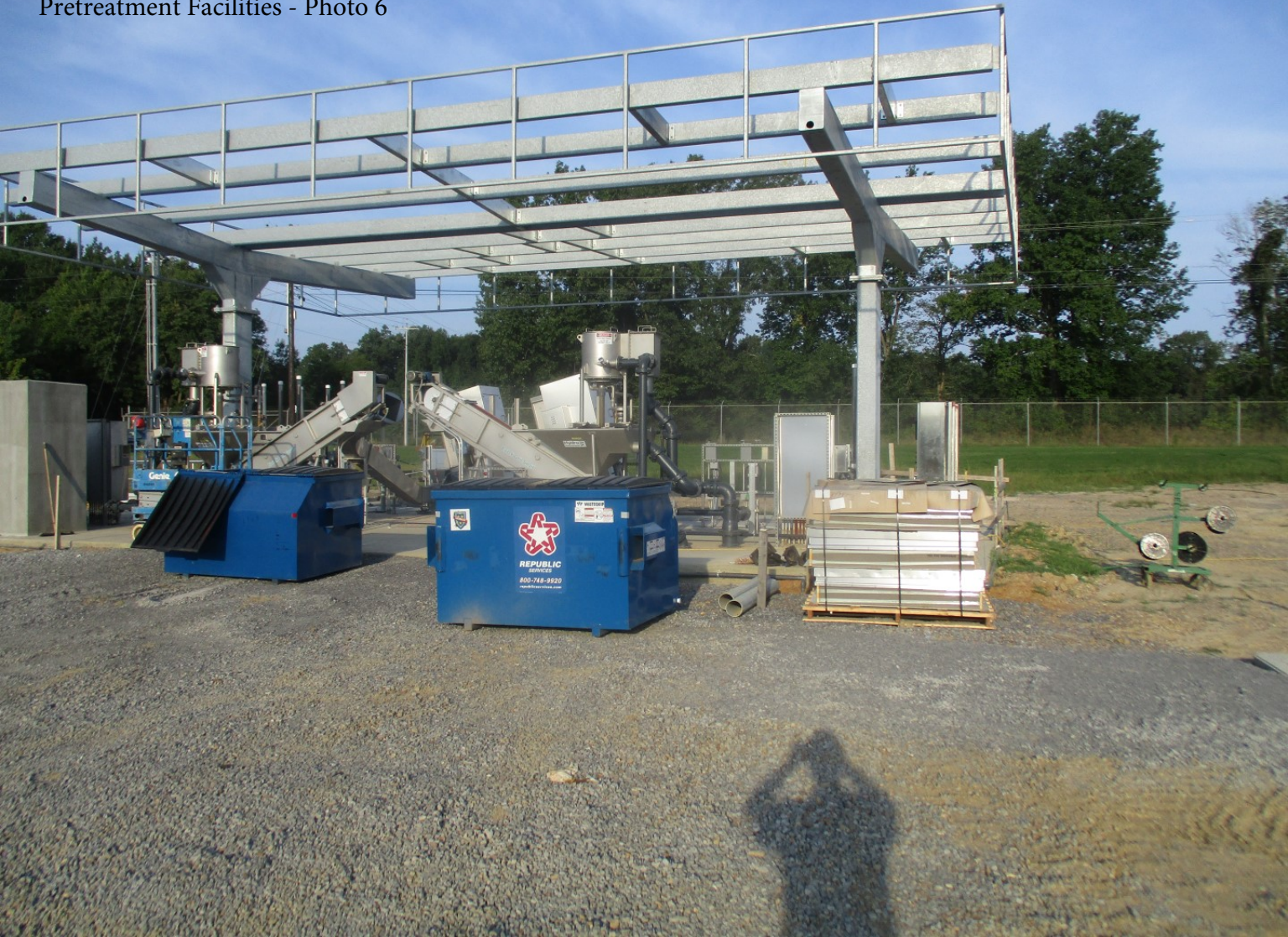
Pretreatment Facilities - Photo 6
