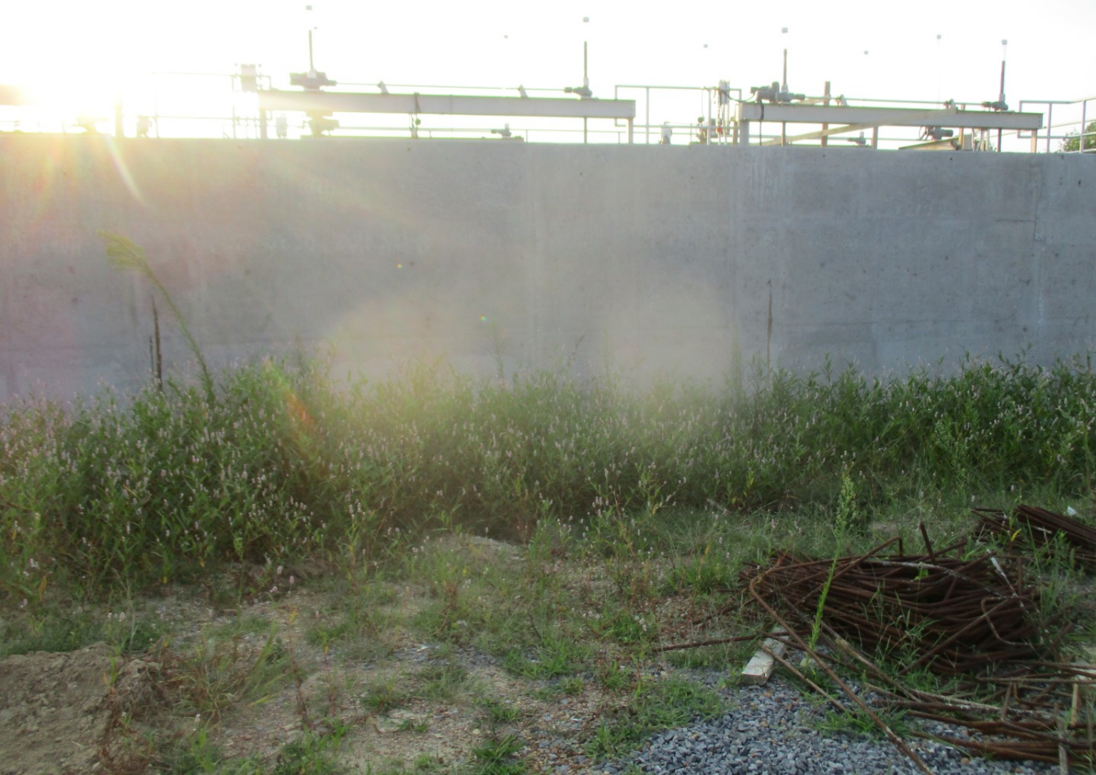
Vertical Loop Reactor - Photo 2
