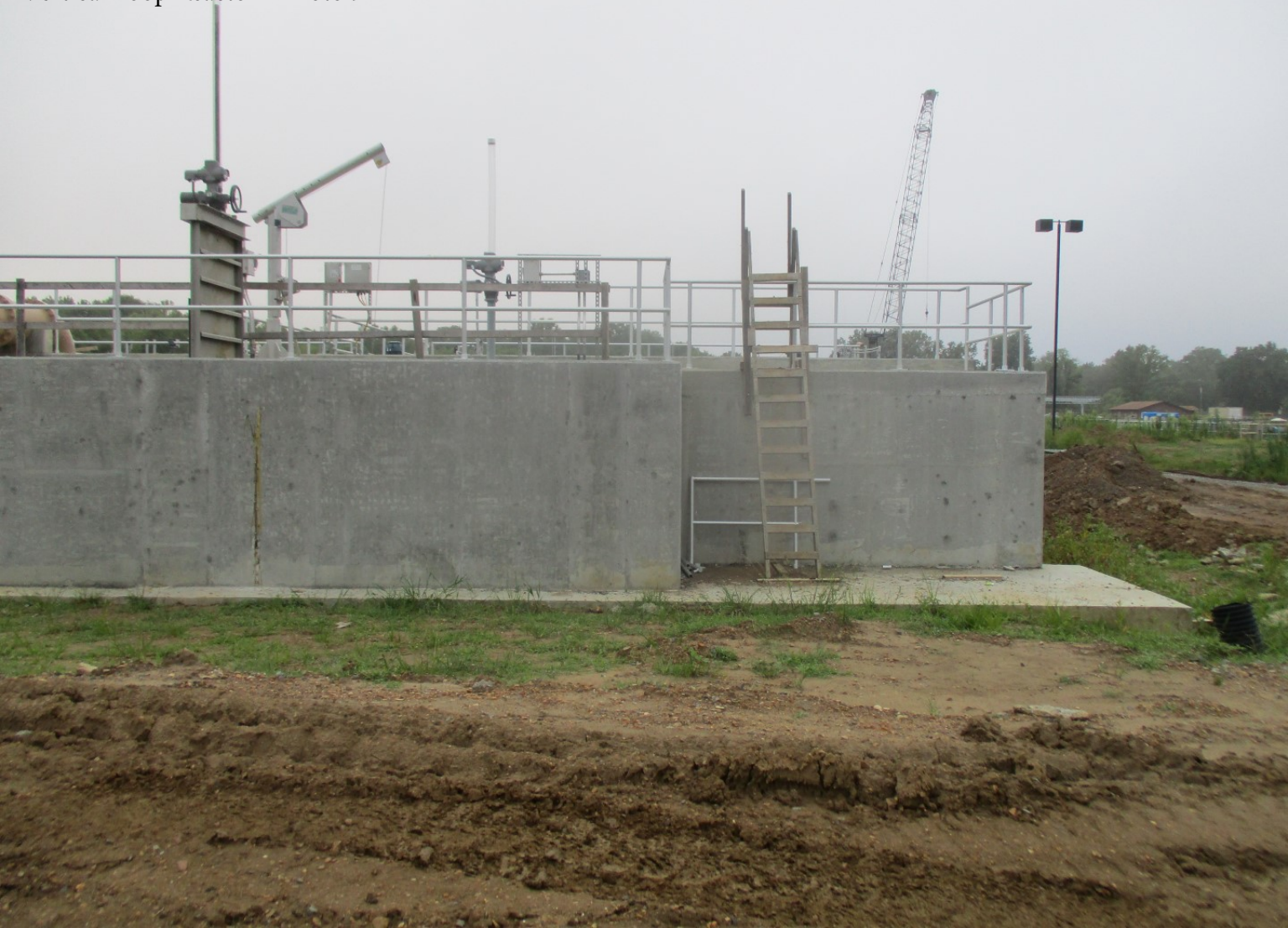
Vertical Loop Reactor - Photo 7
