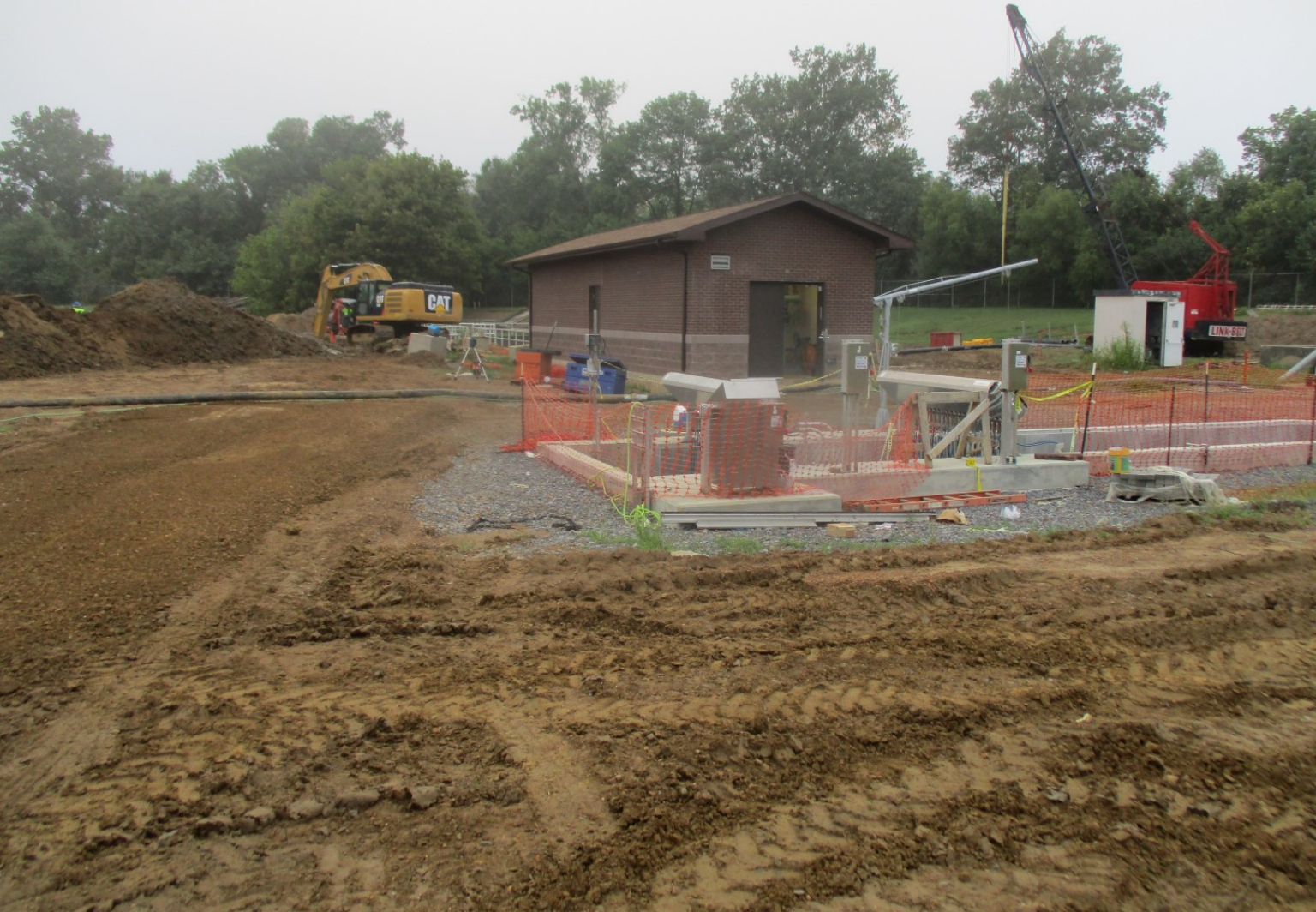
Electrical Building No. 3 - Photo 2
