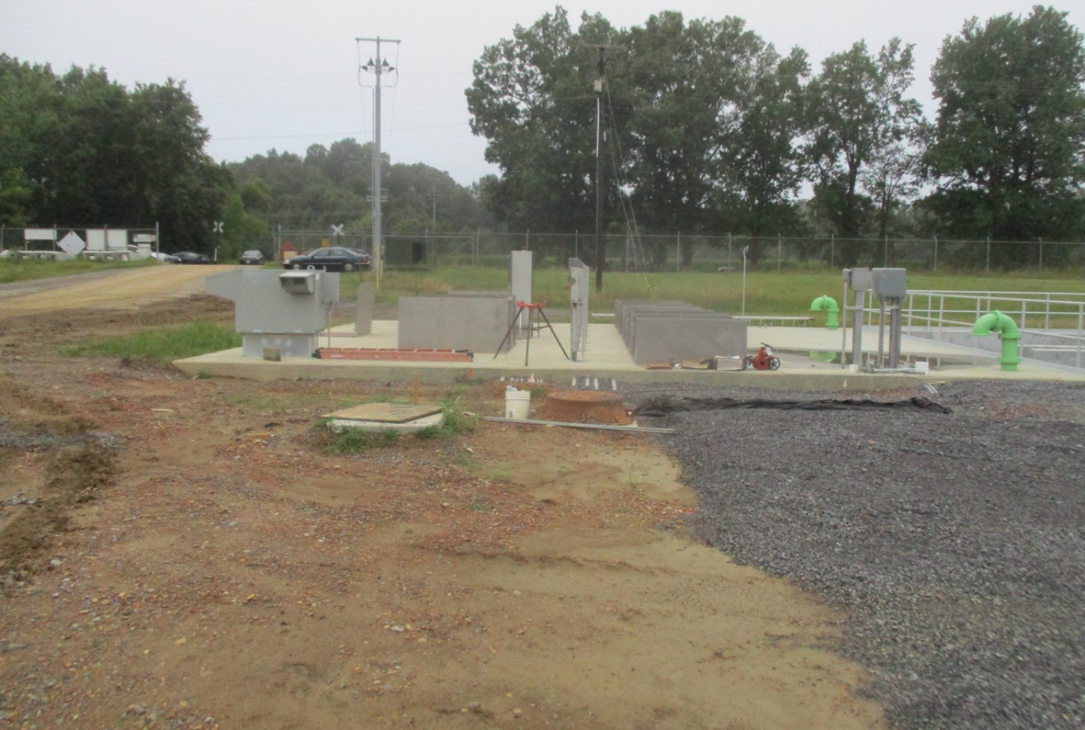
Pretreatment Facilities - Photo 4
