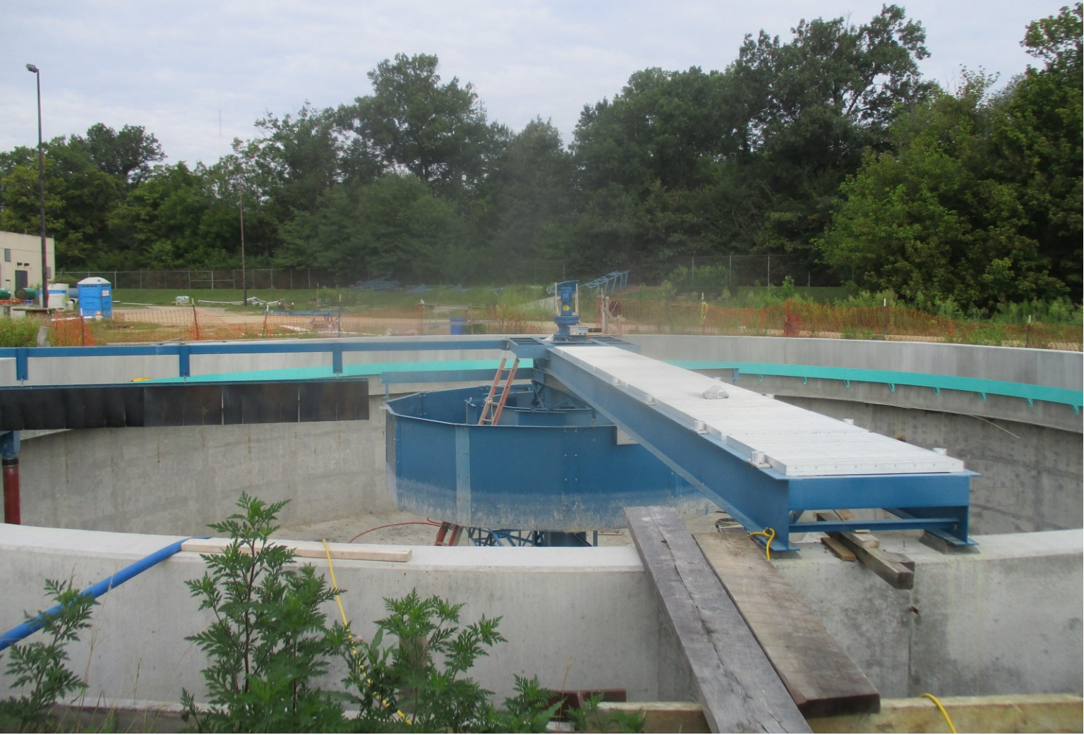
Clarifier No. 6 - Photo 1
