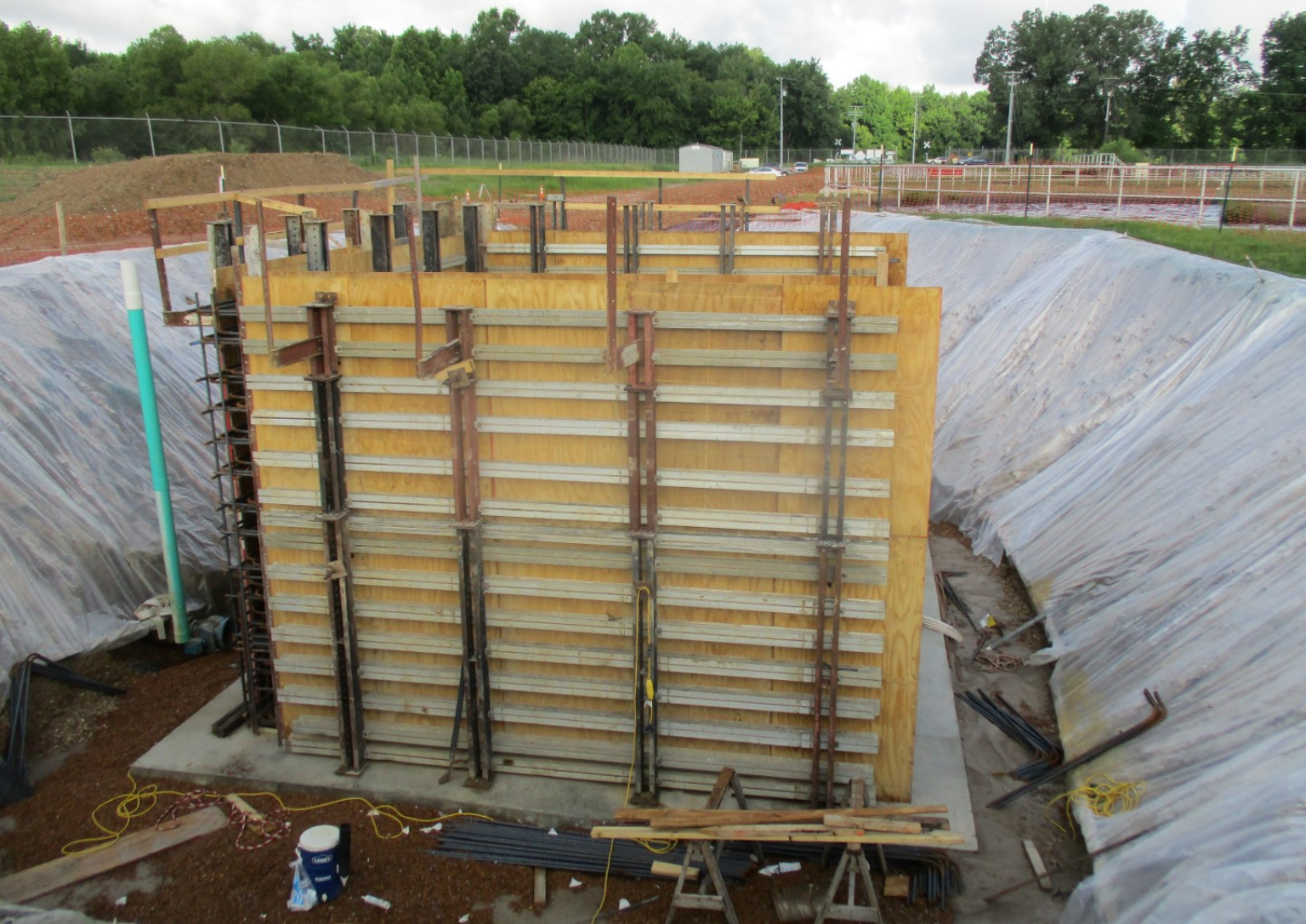
Nitrate Pump Station - Photo 1
