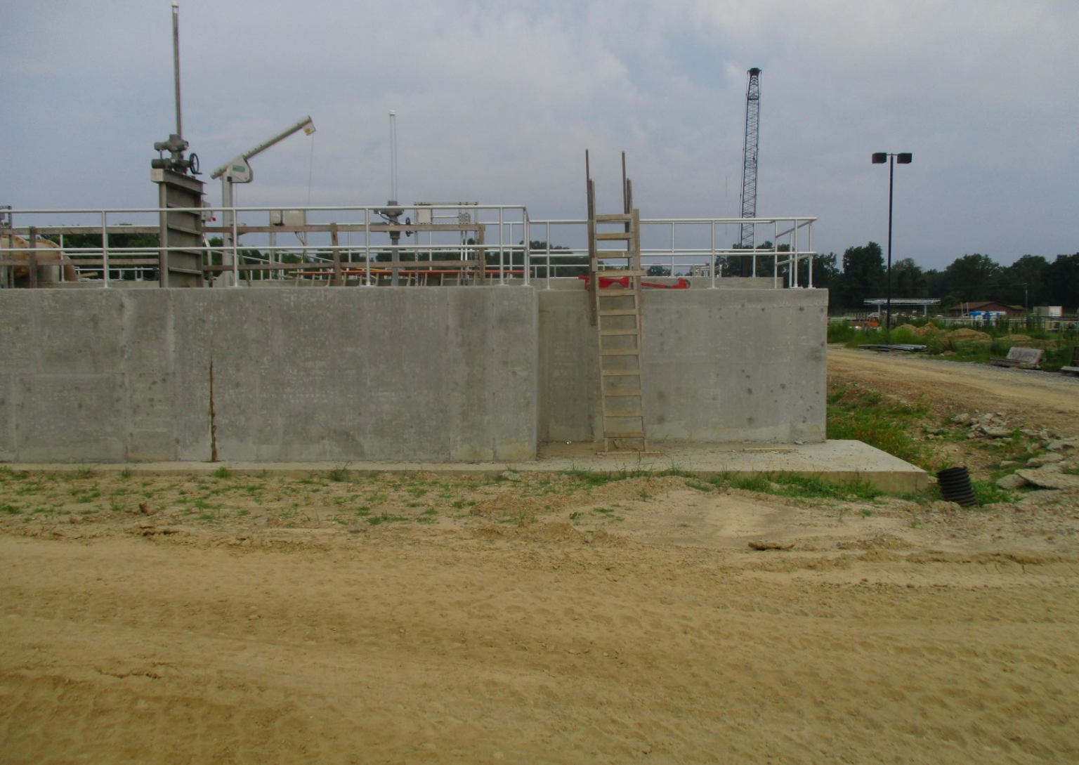
Vertical Loop Reactor - Photo 7
