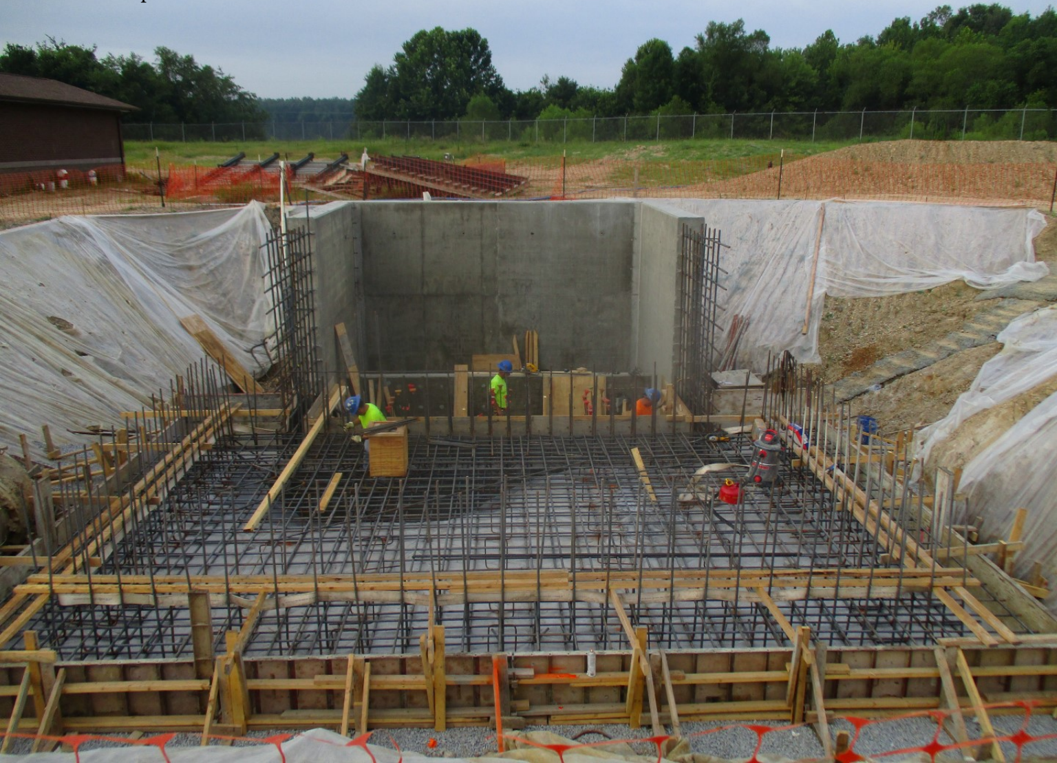
Nitrate Pump Station - Photo 2
