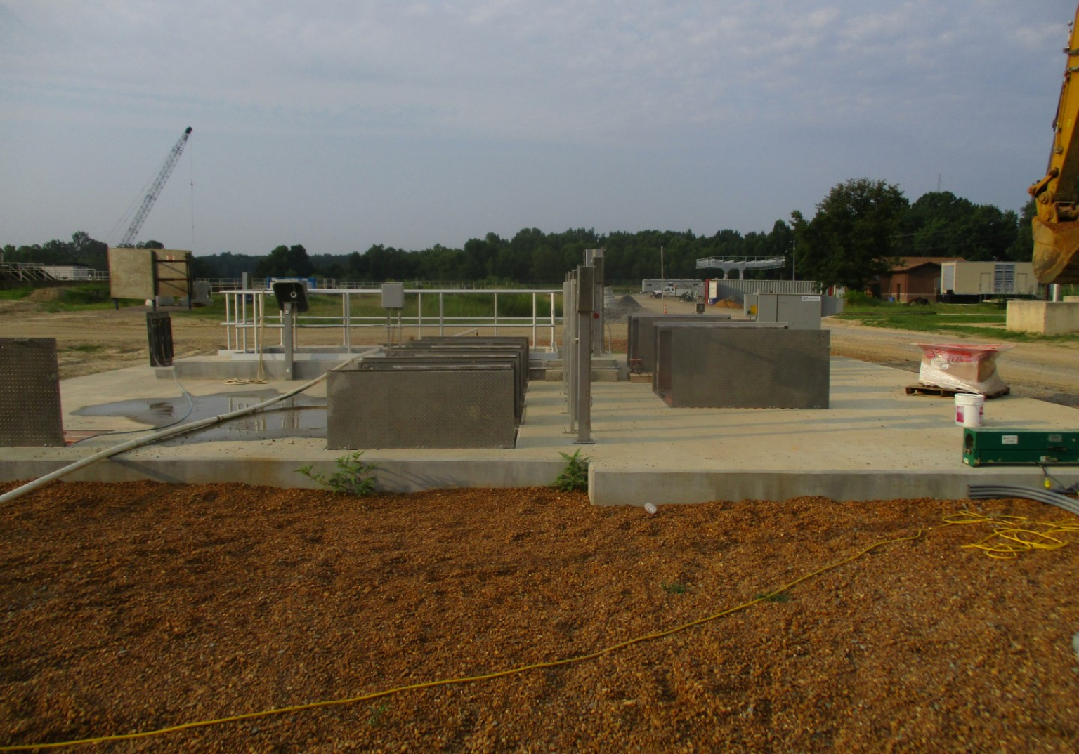
RAS Pump Station - Photo 3
