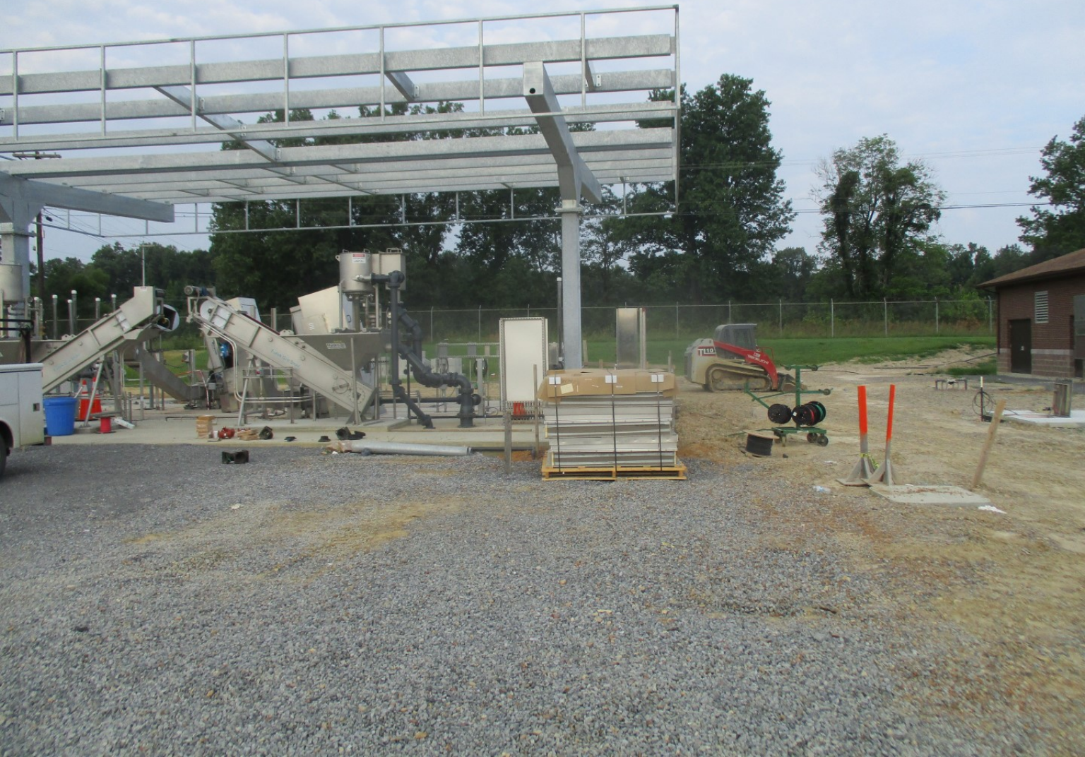
Pretreatment Facilities - Photo 6
