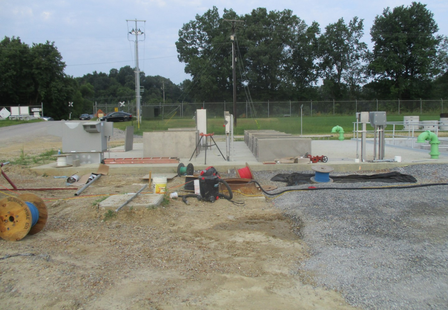
Pretreatment Facilities - Photo 4
