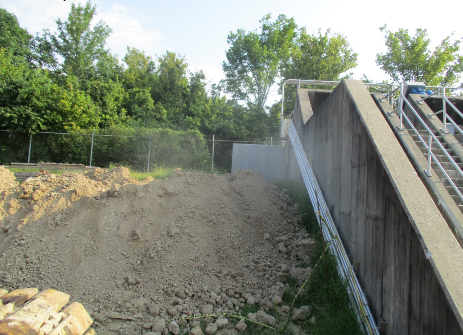
NPW Pump Station Influent - Photo 2
