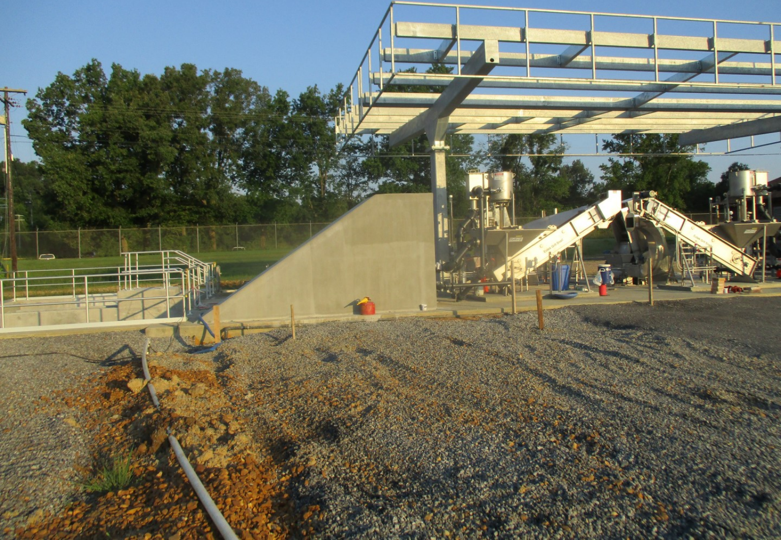
Pretreatment Facilities - Photo 5
