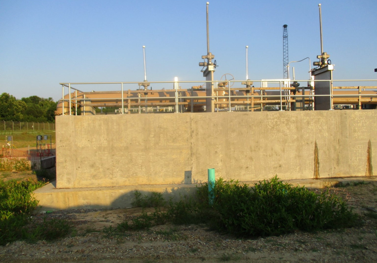
Vertical Loop Reactor - Photo 5
