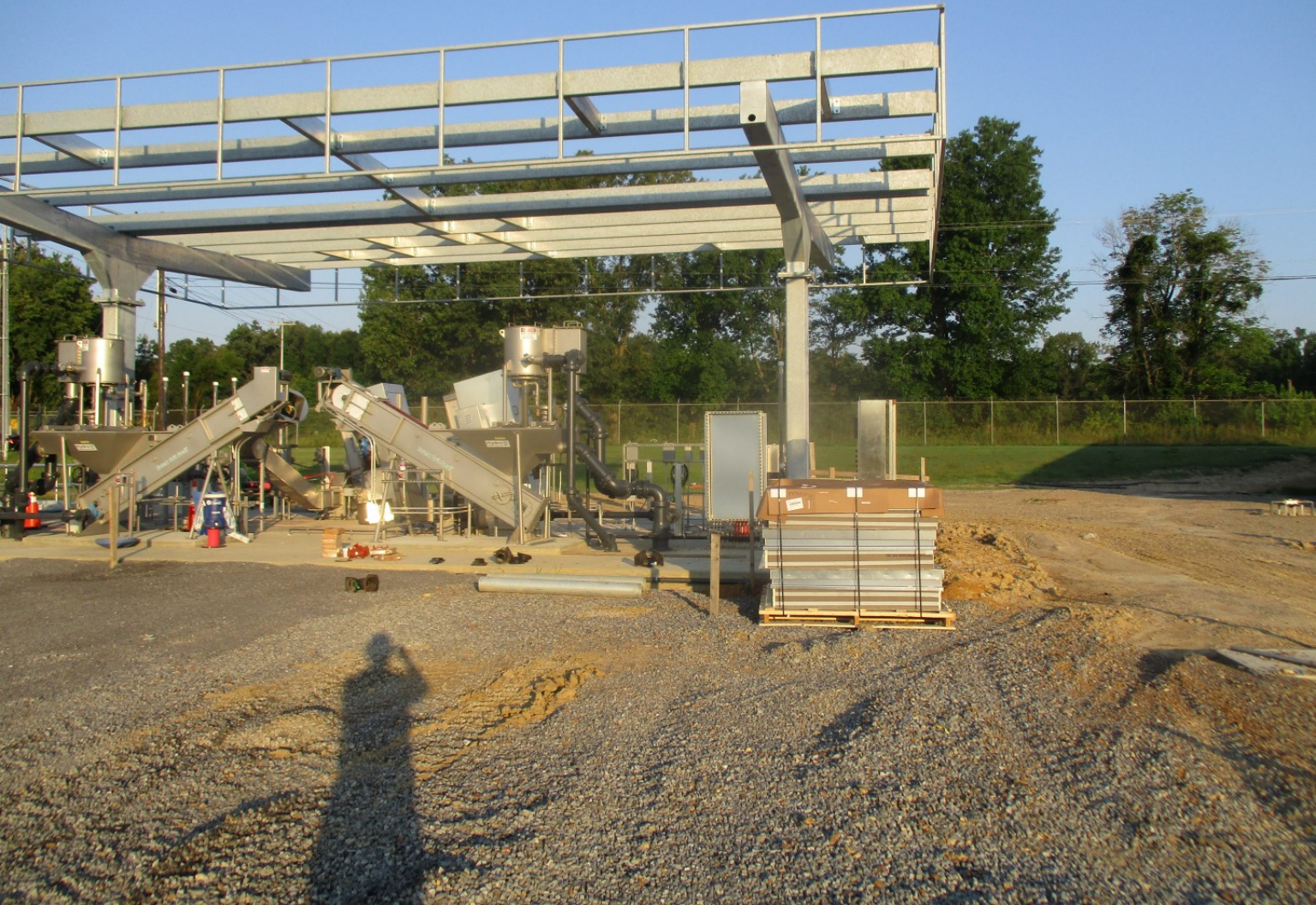
Pretreatment Facilities - Photo 6
