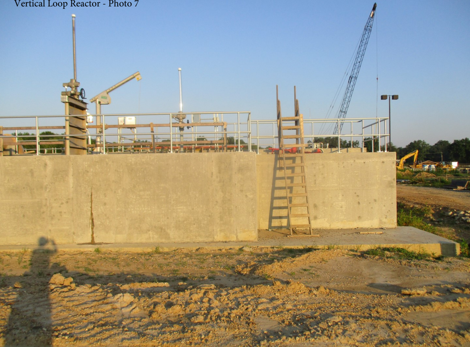
Vertical Loop Reactor - Photo 7
