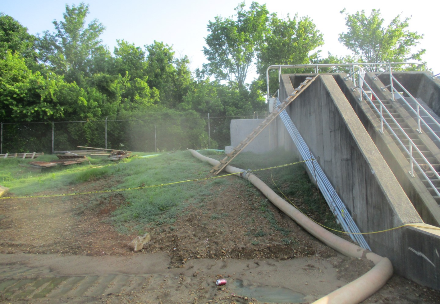
NPW Pump Station Influent - Photo 2
