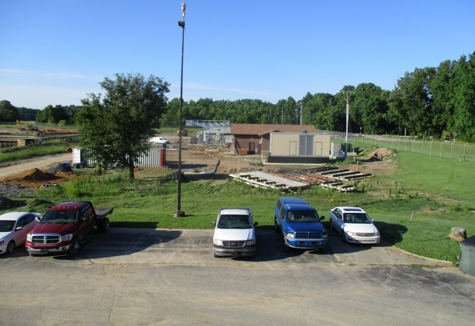
Pretreatment Facilities - Photo 7
