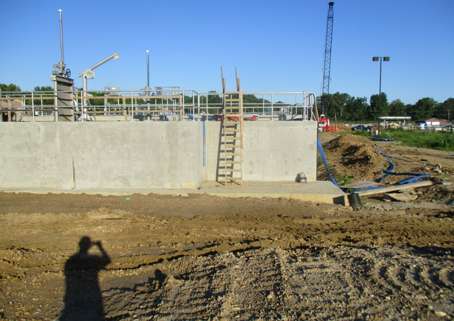
Vertical Loop Reactor - Photo 7
