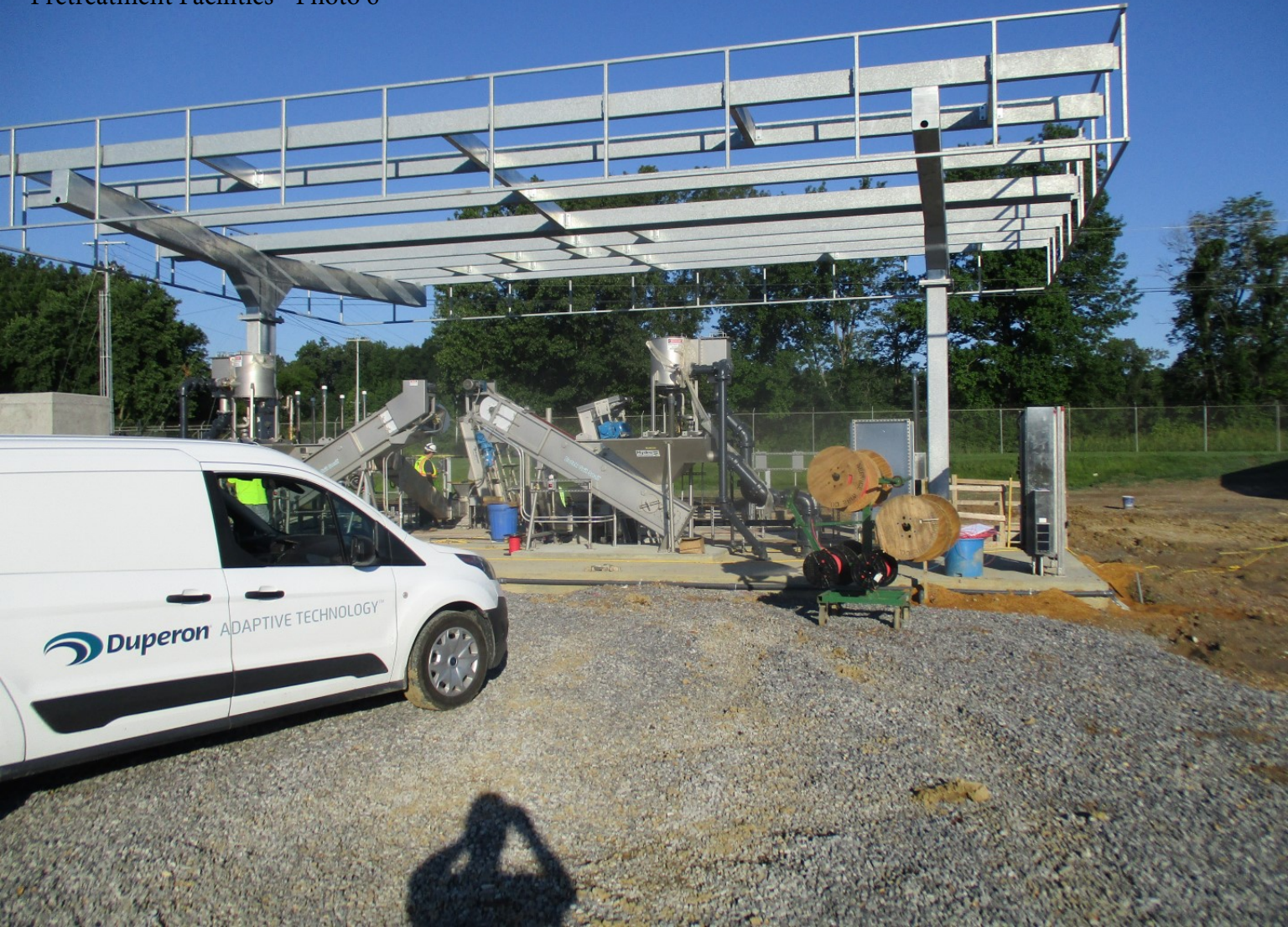
Pretreatment Facilities - Photo 6
