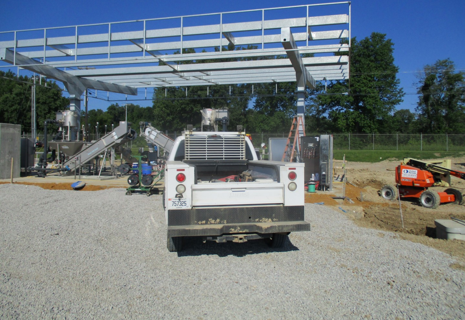
Pretreatment Facilities - Photo 6
