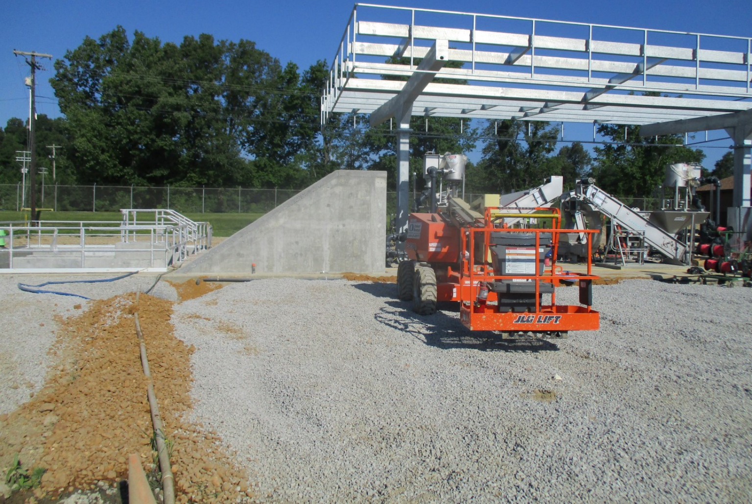
Pretreatment Facilities - Photo 5
