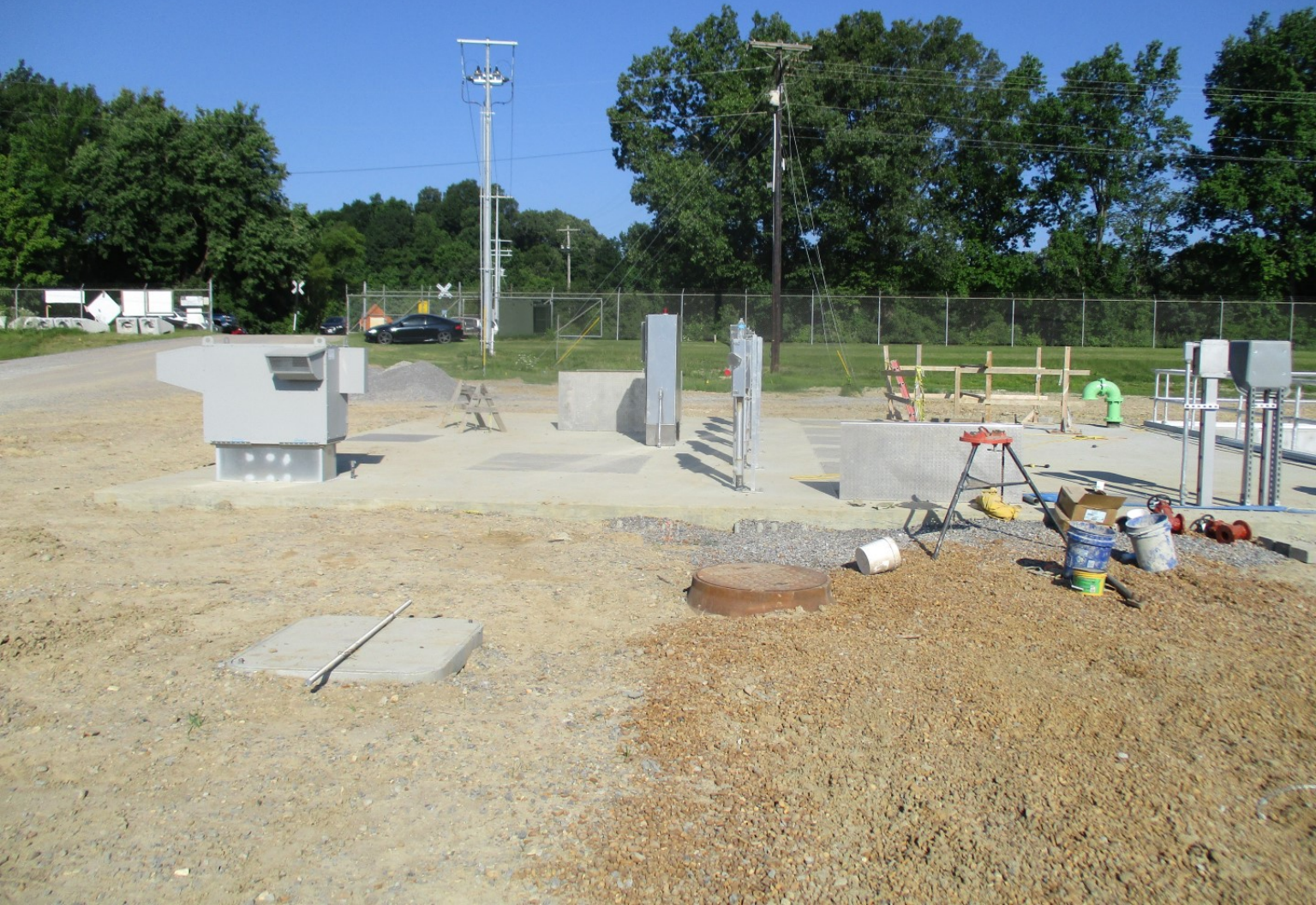
Pretreatment Facilities - Photo 4
