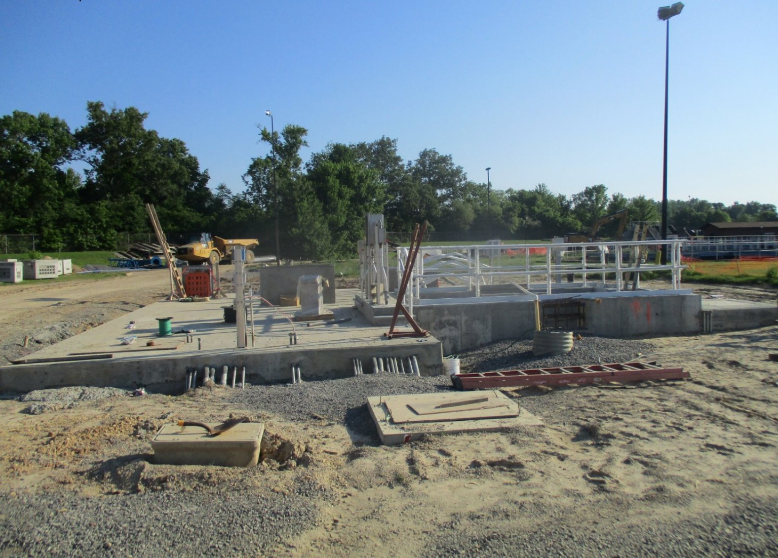
RAS Pump Station - Photo 2
