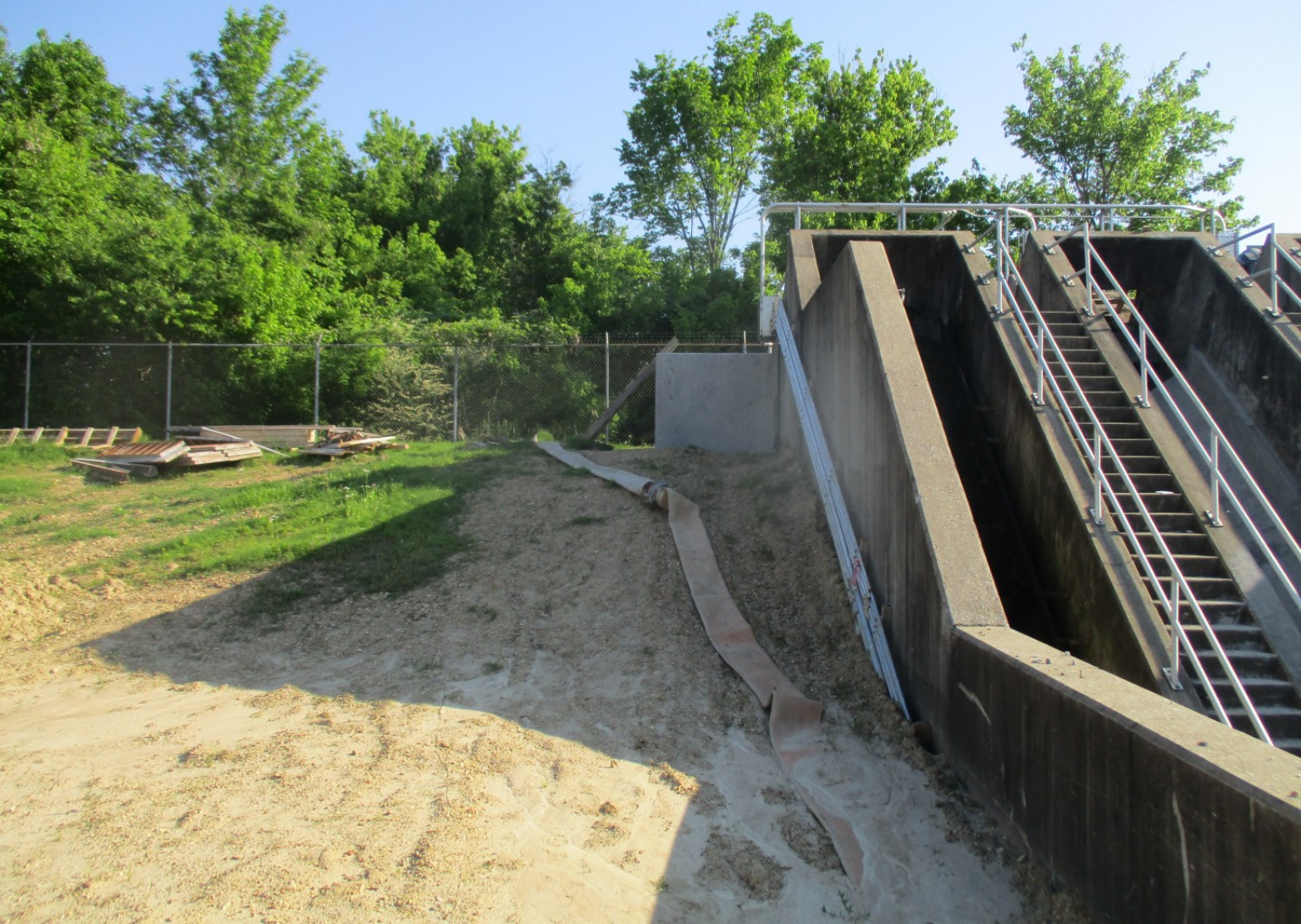
NPW Pump Station Influent - Photo 2
