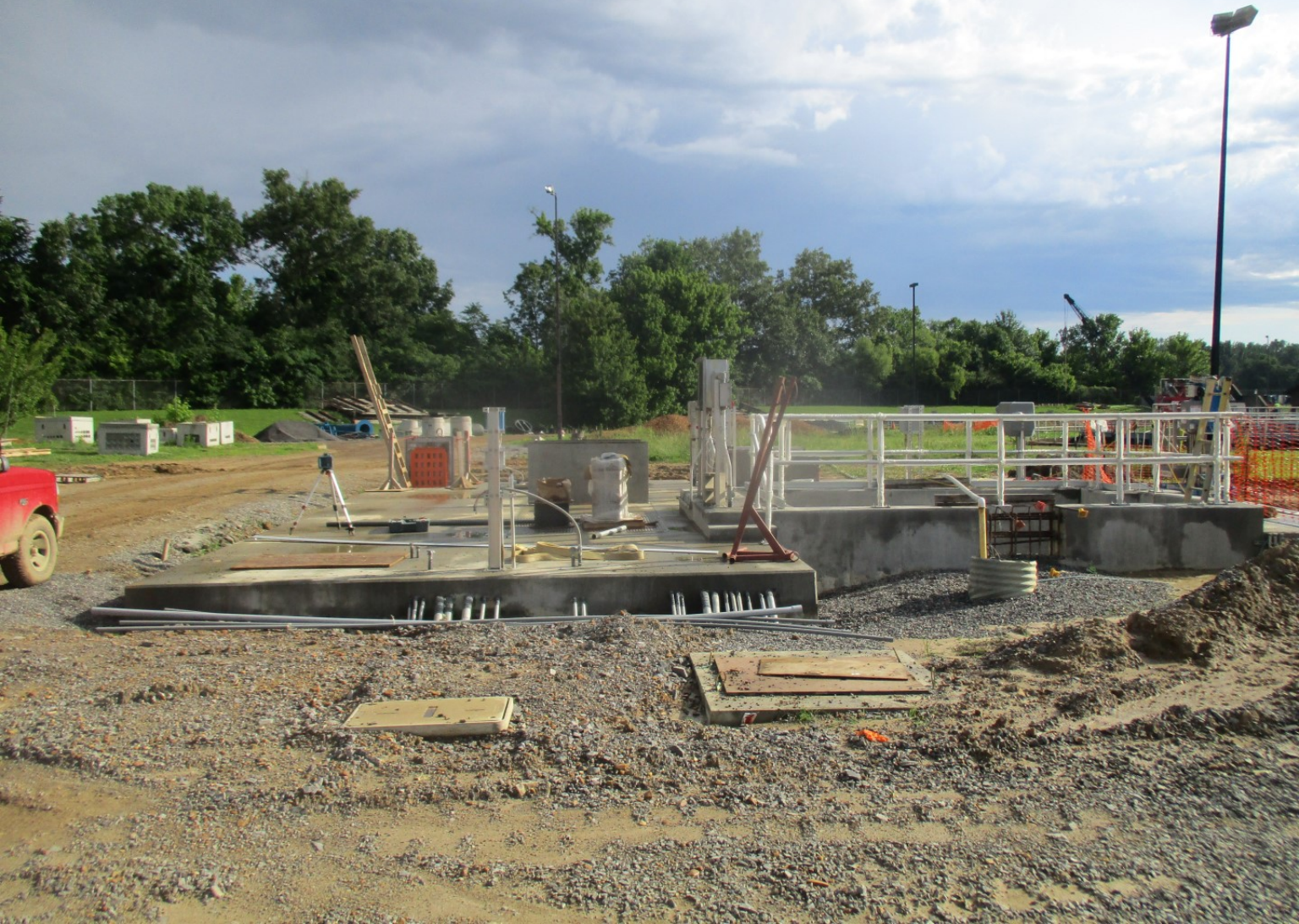
RAS Pump Station - Photo 2
