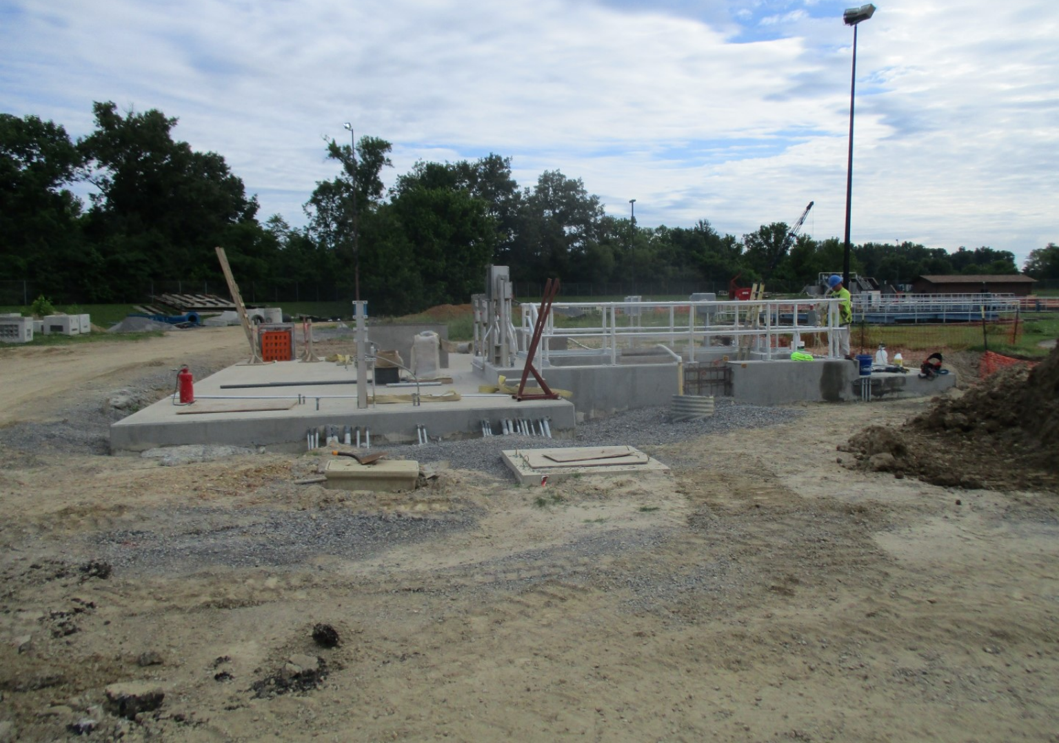
RAS Pump Station - Photo 2
