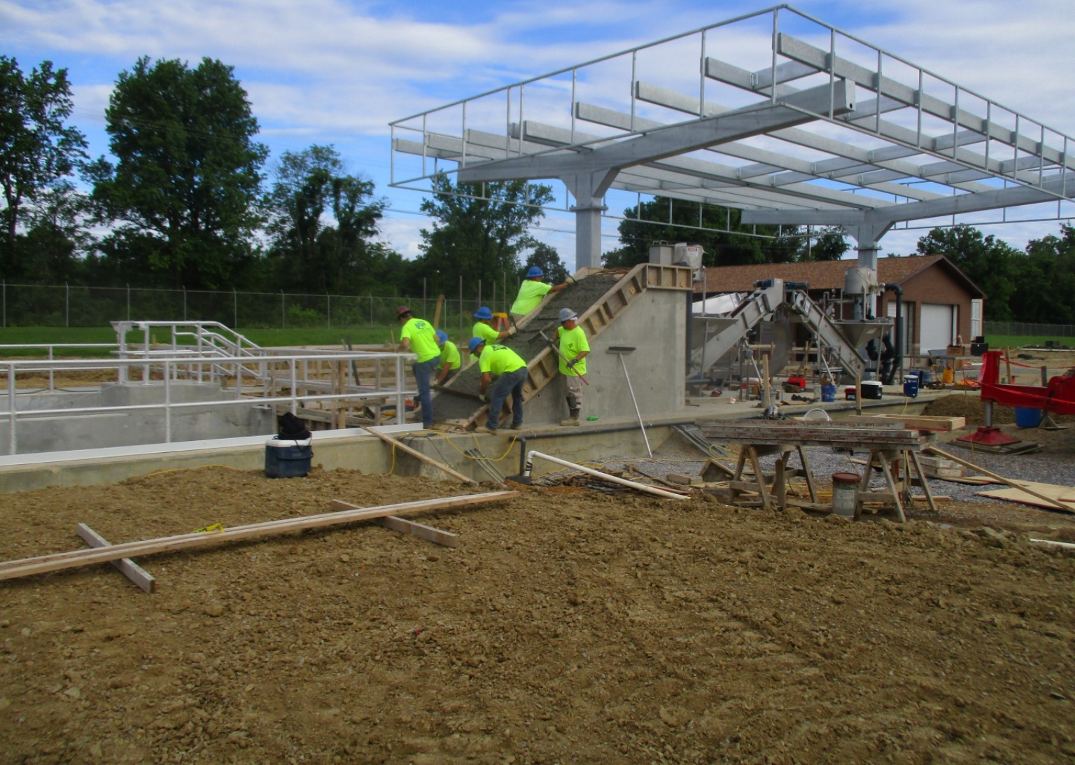
Pretreatment Facilities - Photo 5
