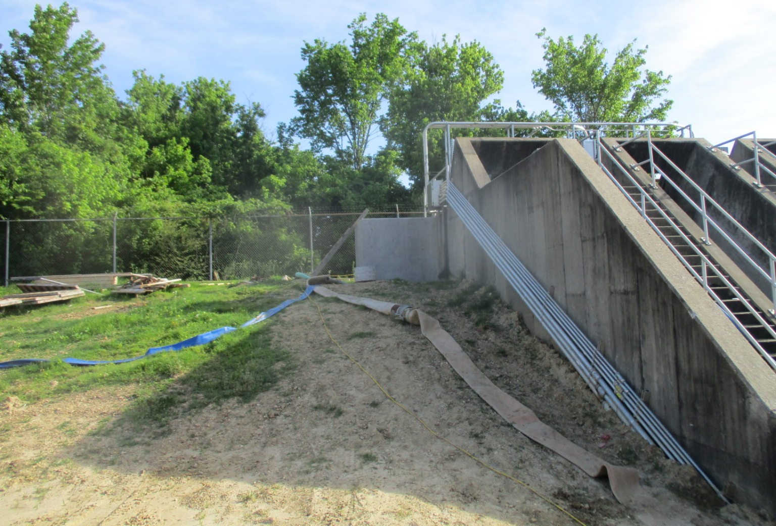
NPW Pump Station Influent - Photo 2
