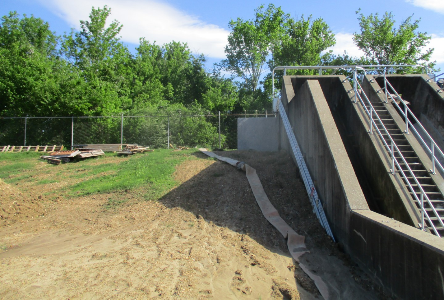
NPW Pump Station Influent - Photo 2
