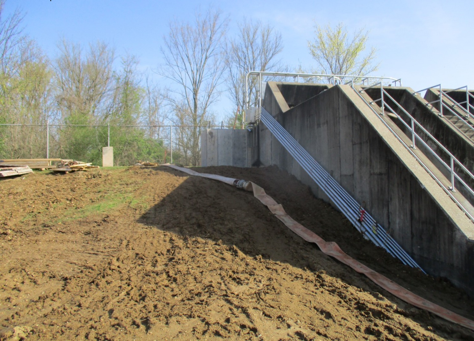
NPW Pump Station Influent - Photo 2
