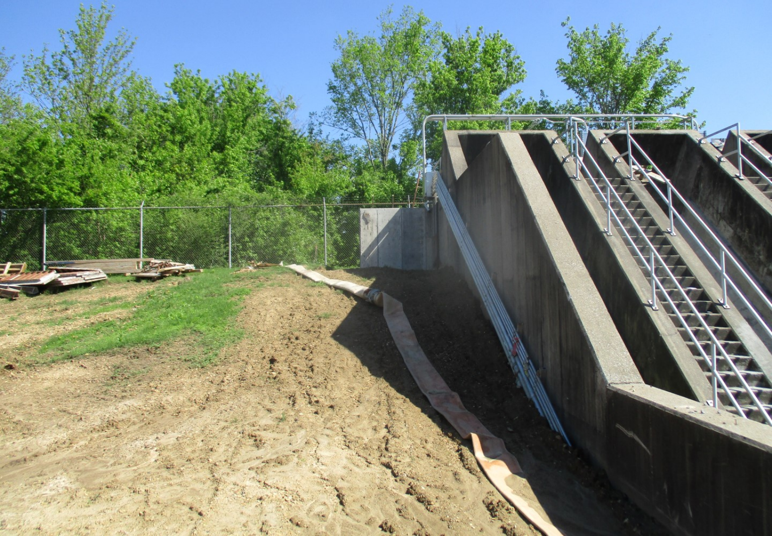
NPW Pump Station Influent - Photo 2
