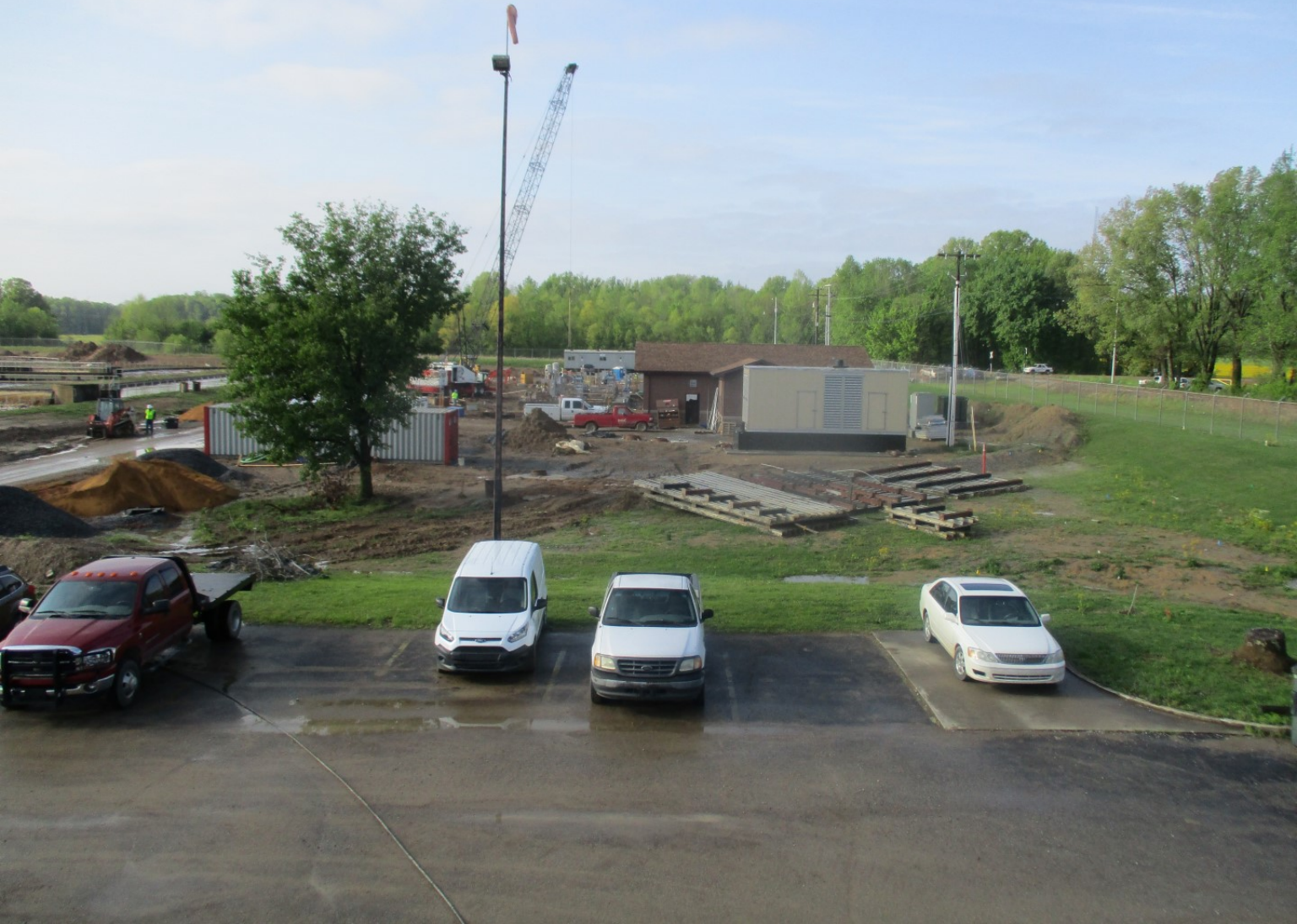
Pretreatment Facilities - Photo 7
