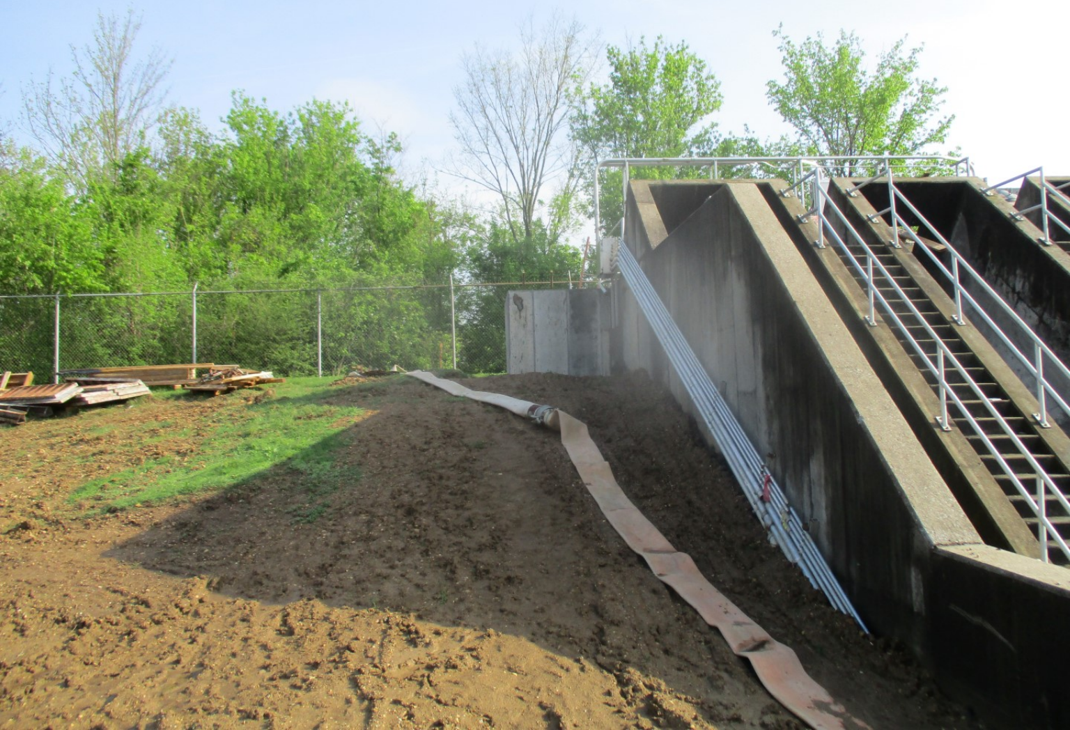
NPW Pump Station Influent - Photo 2
