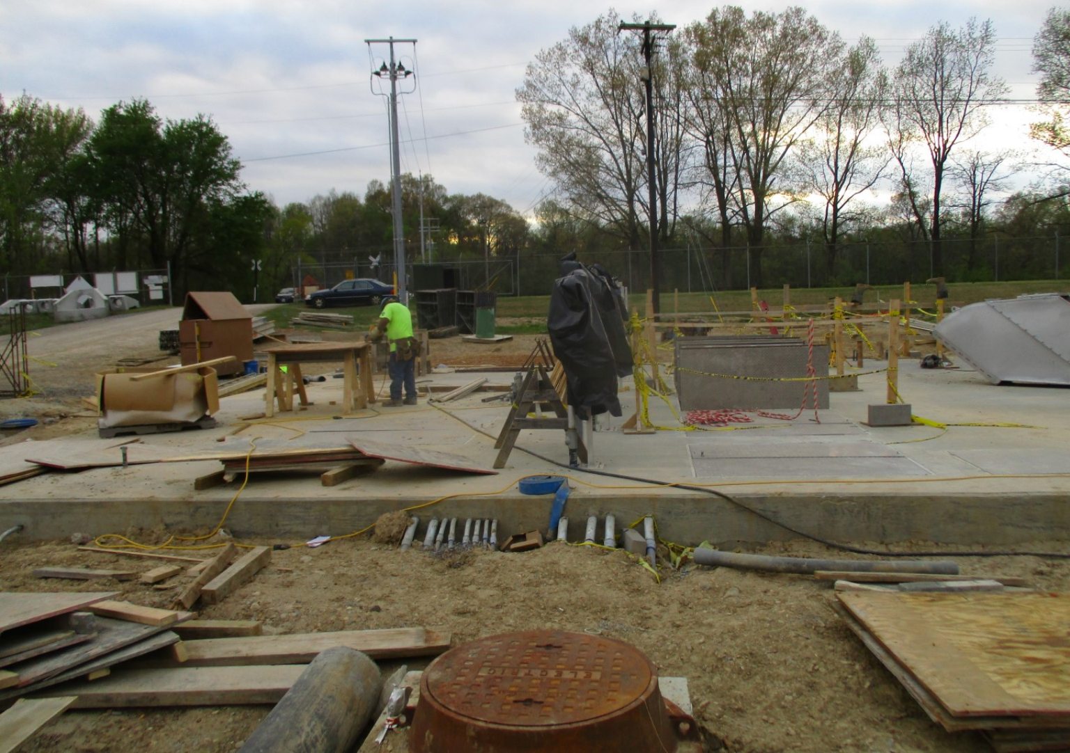
Pretreatment Facilities - Photo 4
