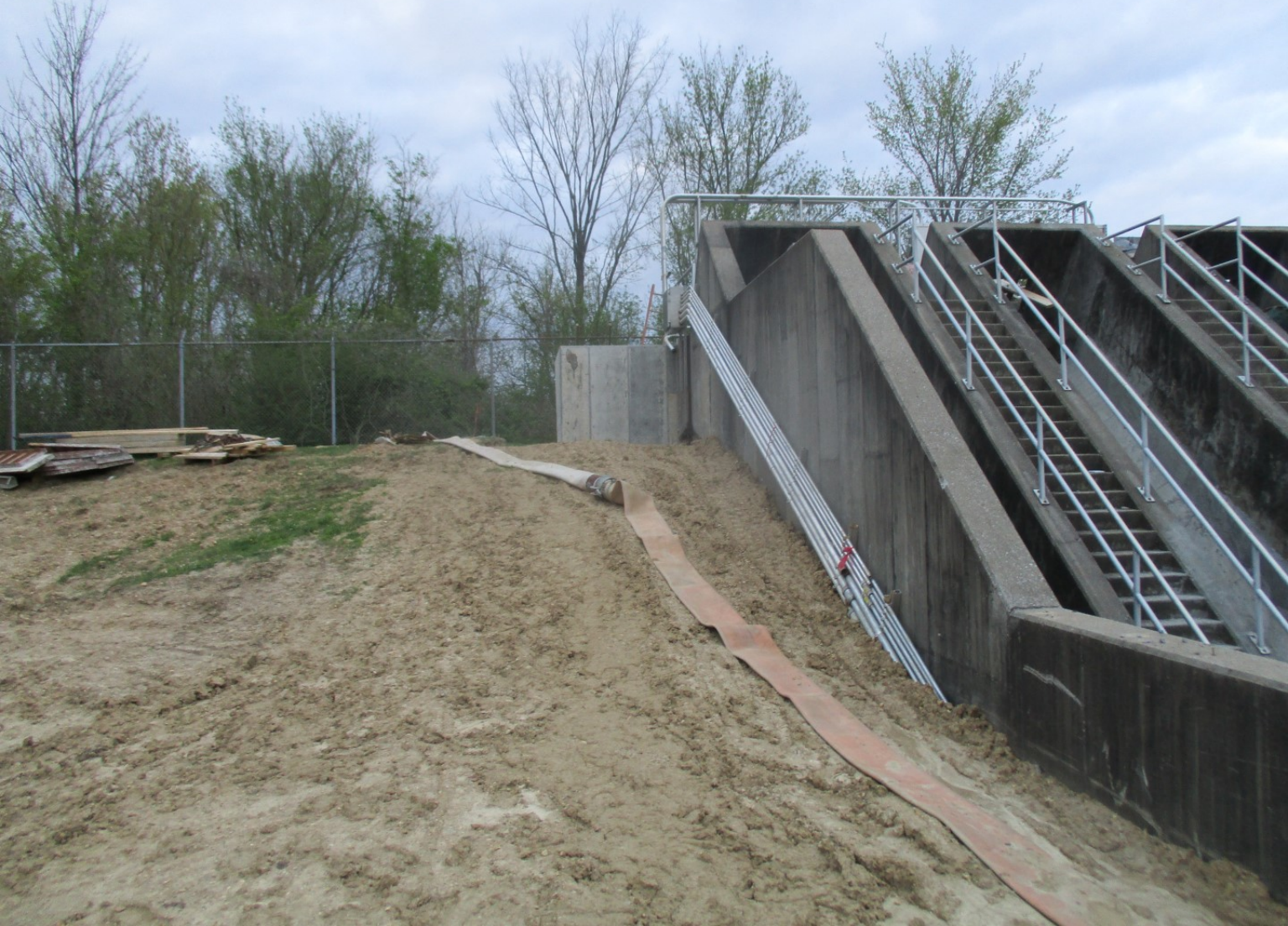
NPW Pump Station Influent - Photo 2
