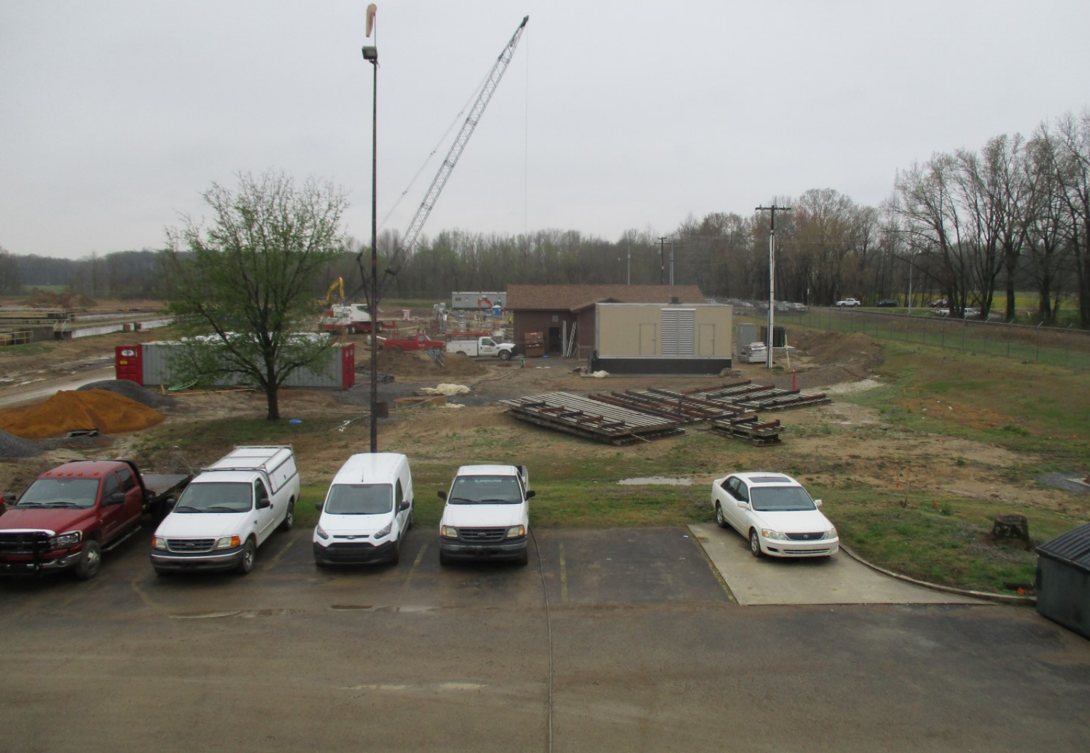
Pretreatment Facilities - Photo 7
