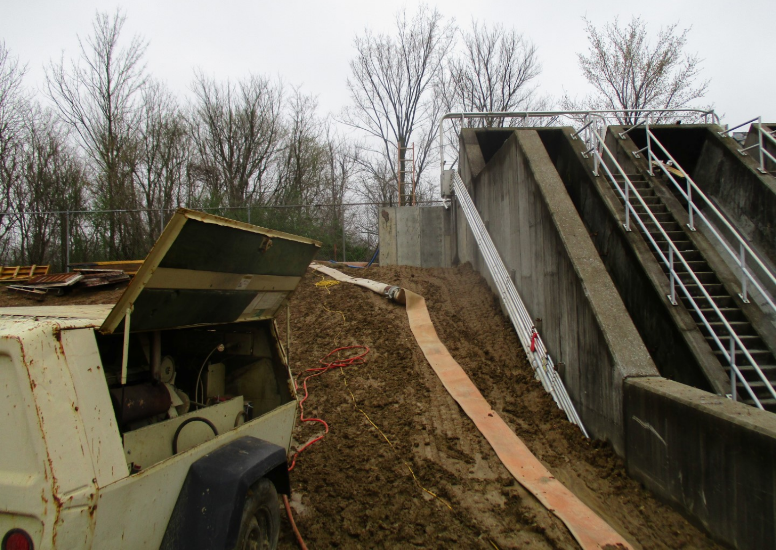
NPW Pump Station Influent - Photo 2
