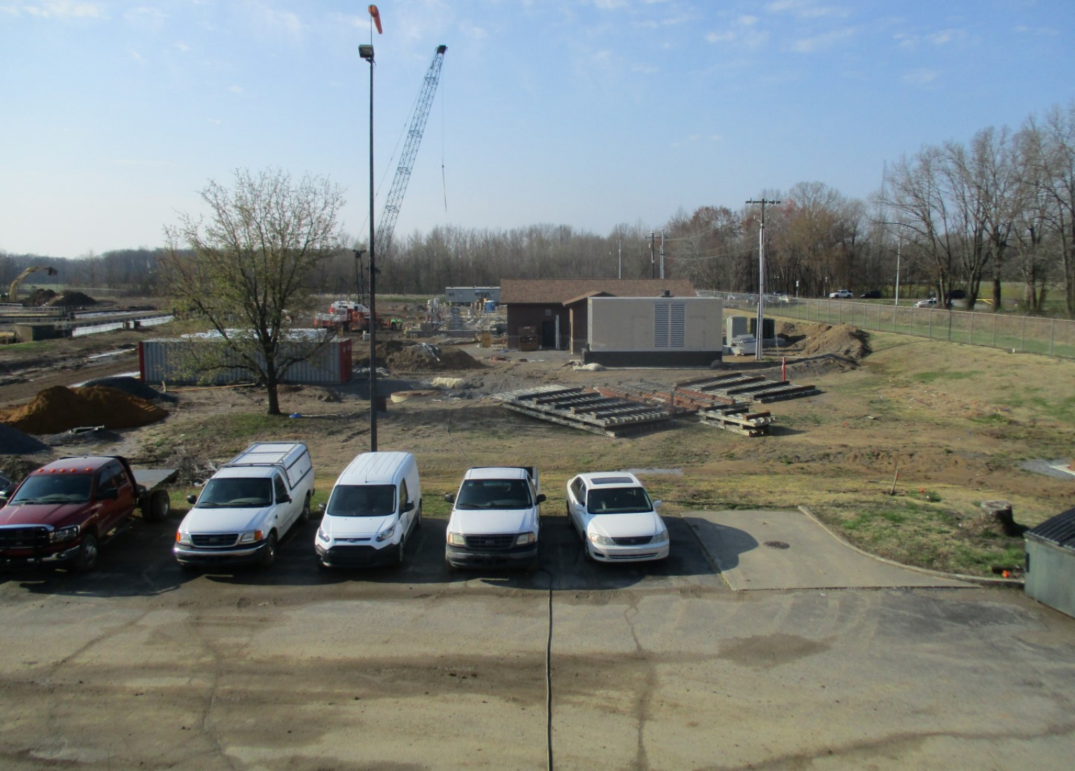
Pretreatment Facilities - Photo 7
