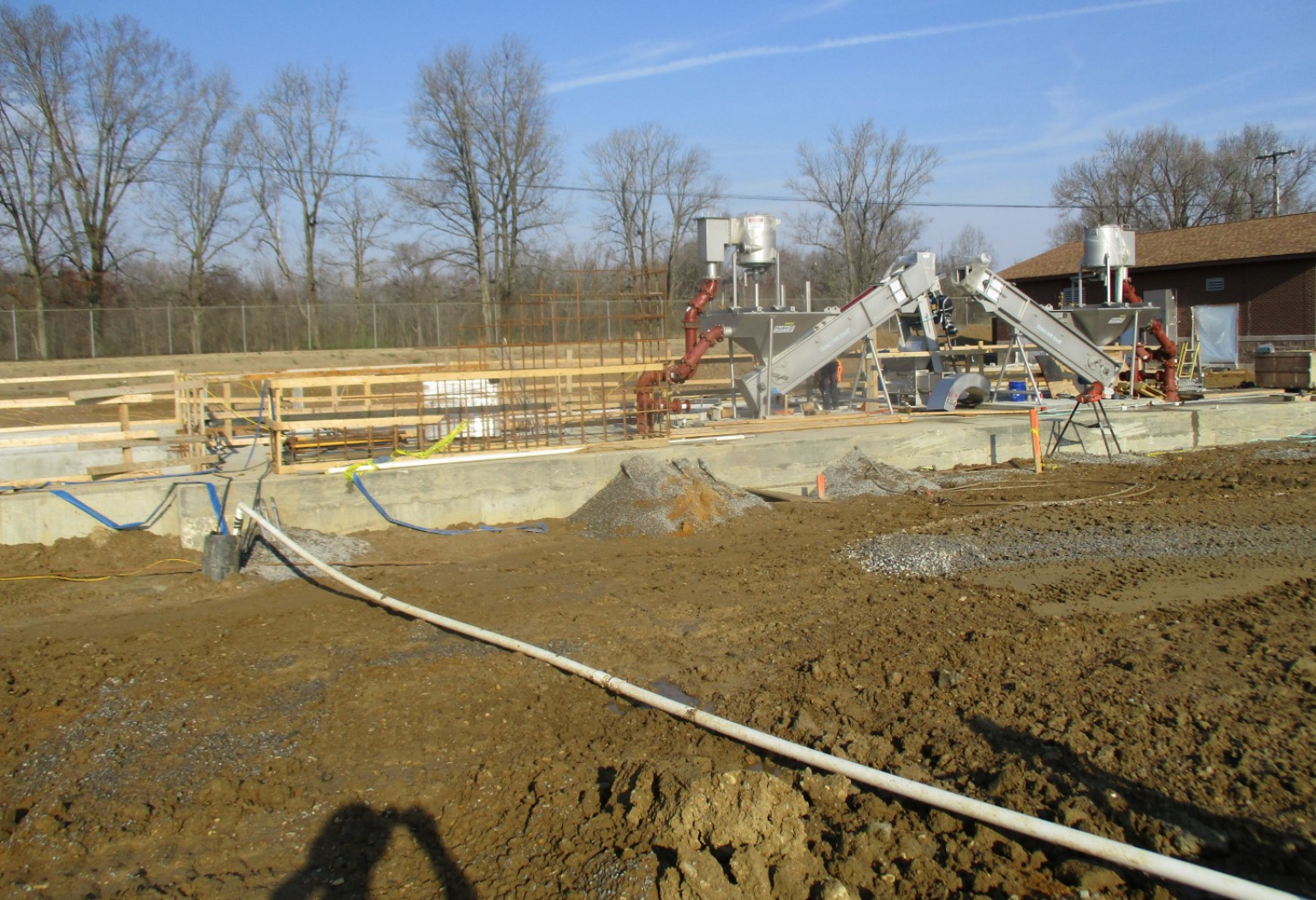
Pretreatment Facilities - Photo 5
