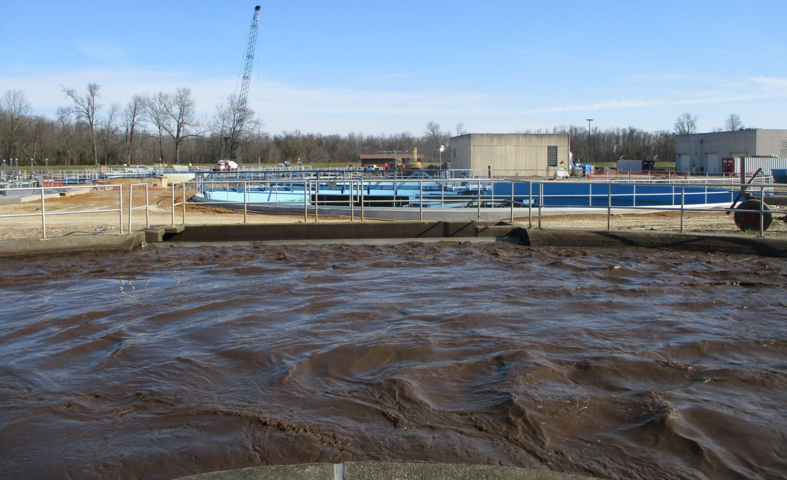
Oxidation Ditch No. 2 - Photo 4
