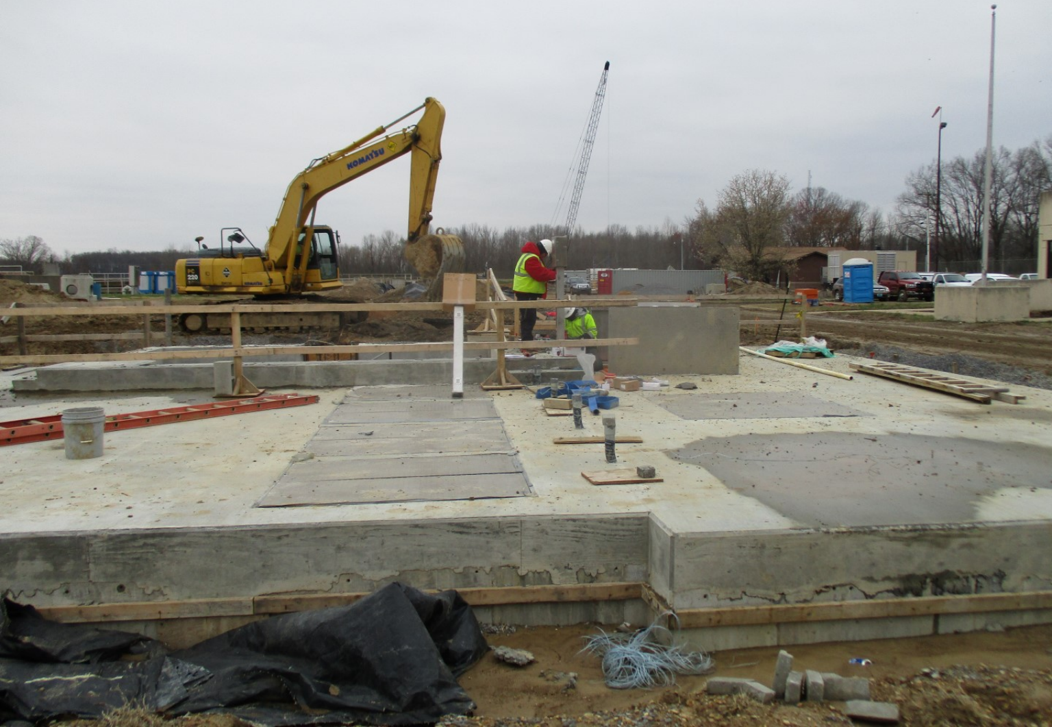
RAS Pump Station - Photo 3
