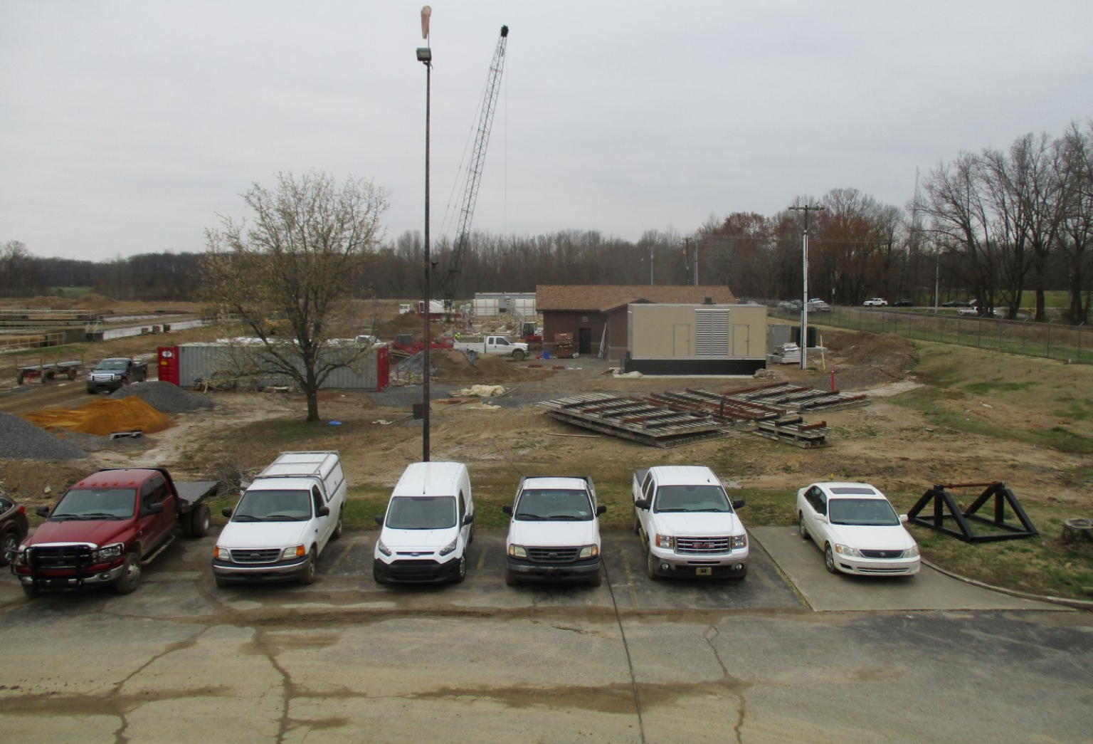
Pretreatment Facilities - Photo 7
