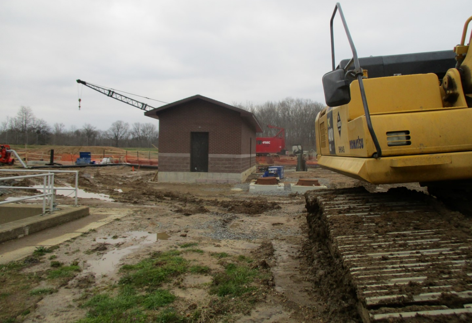
Electrical Building No. 3 - Photo 1
