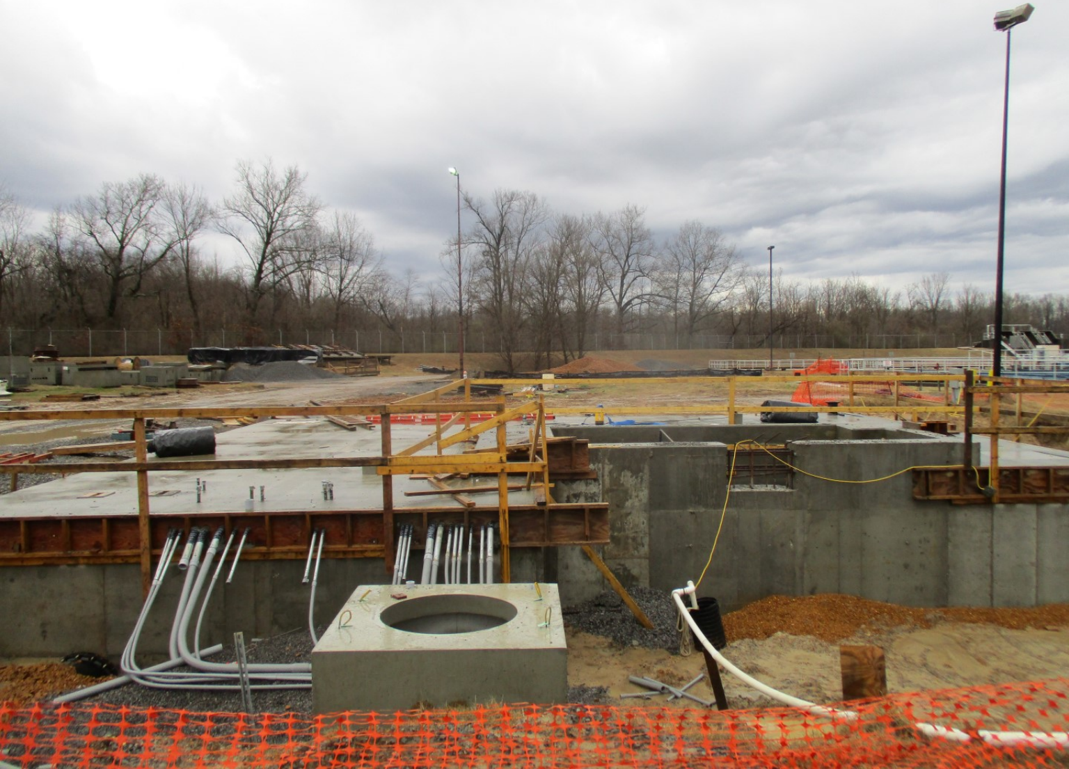
RAS Pump Station - Photo 2
