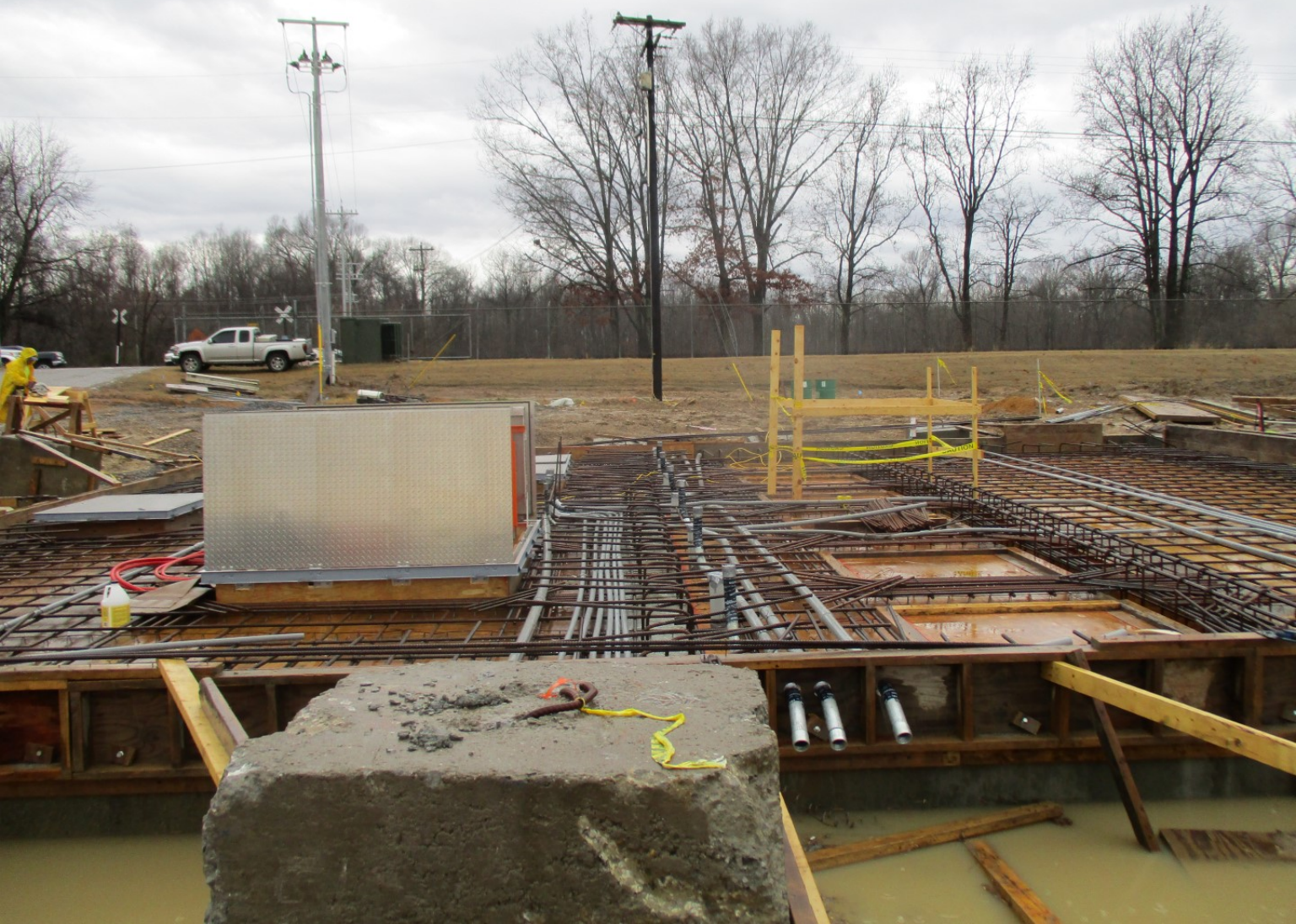
Pretreatment Facilities - Photo 4
