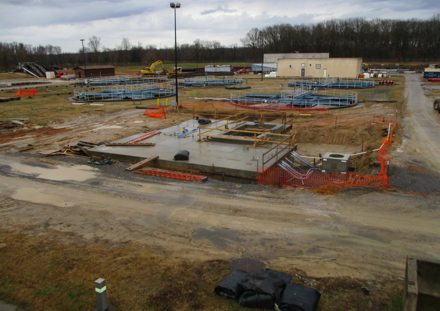
RAS Pump Station - Photo 1
