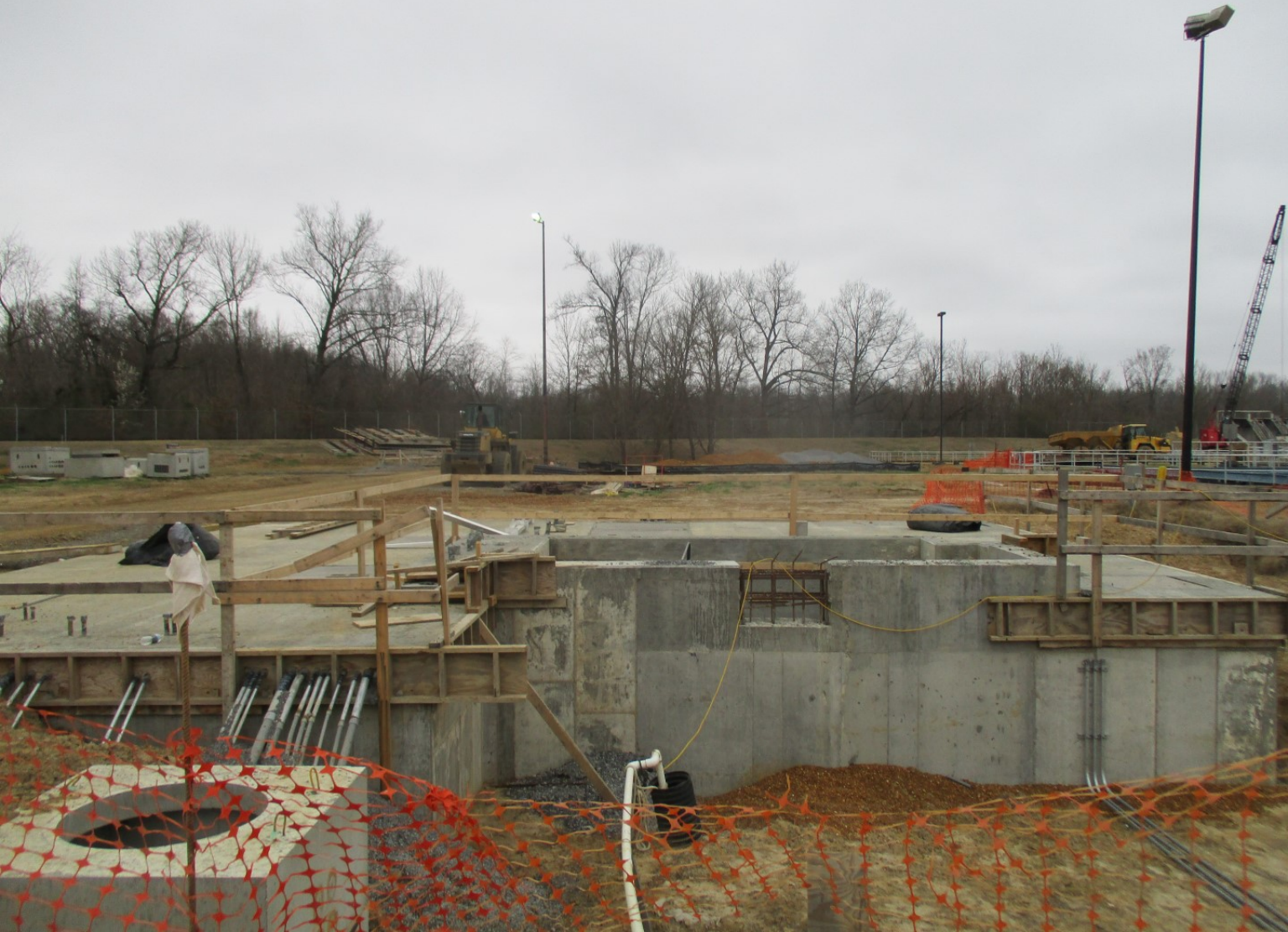
RAS Pump Station - Photo 2
