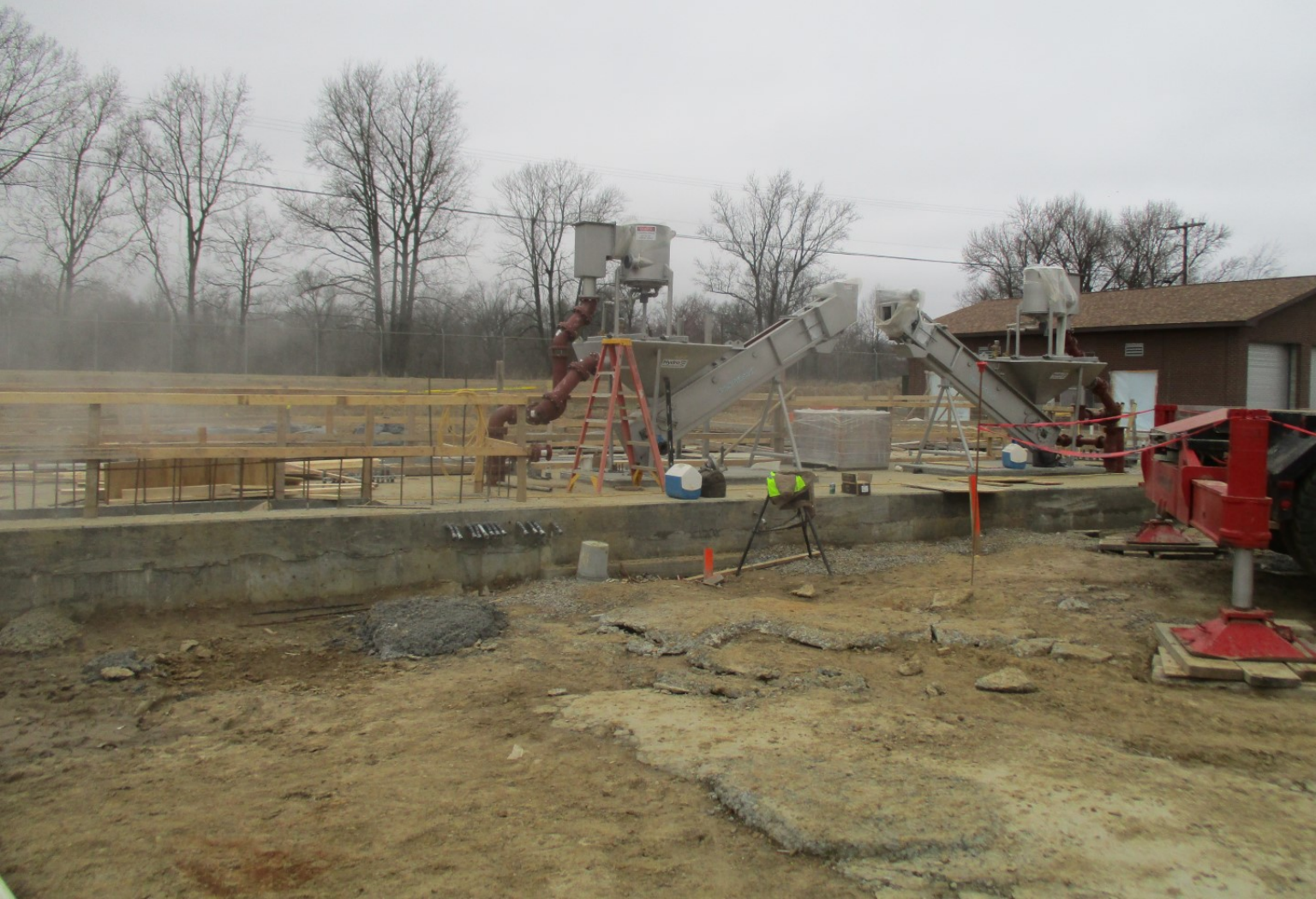
Pretreatment Facilities - Photo 5
