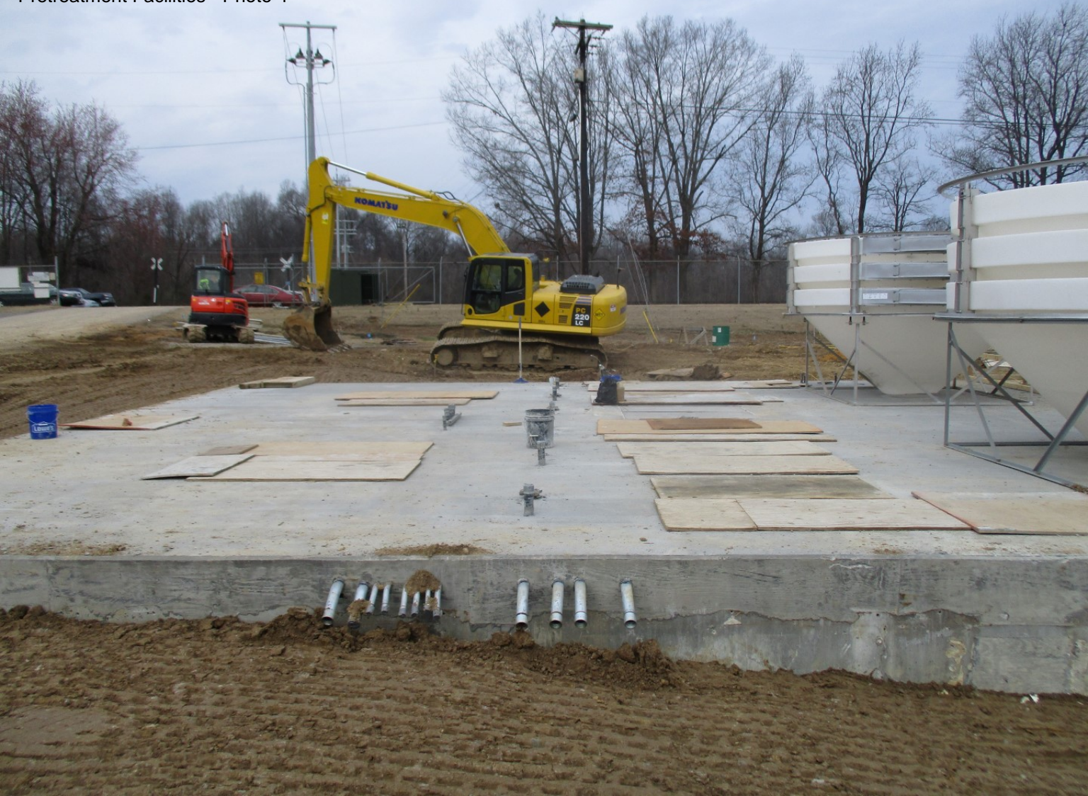
Pretreatment Facilities - Photo 4
