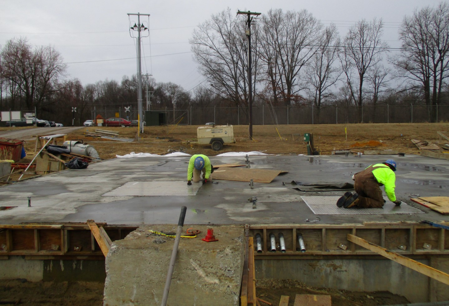
Pretreatment Facilities - Photo 4
