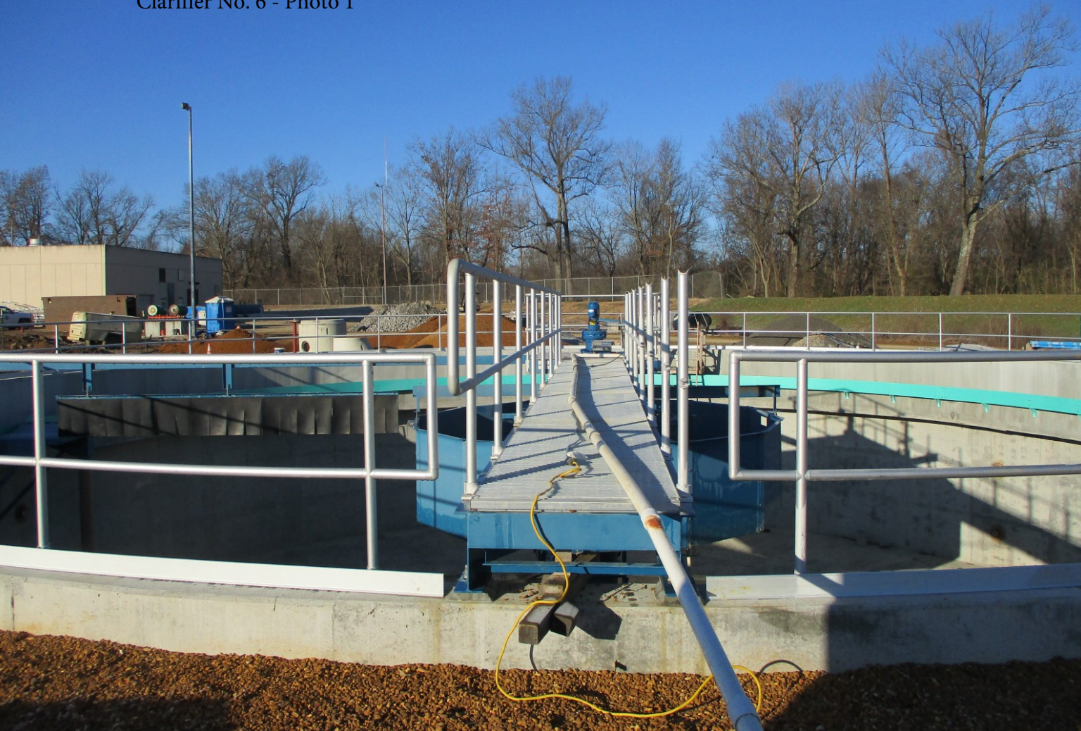
Clarifier No. 6 - Photo 1
