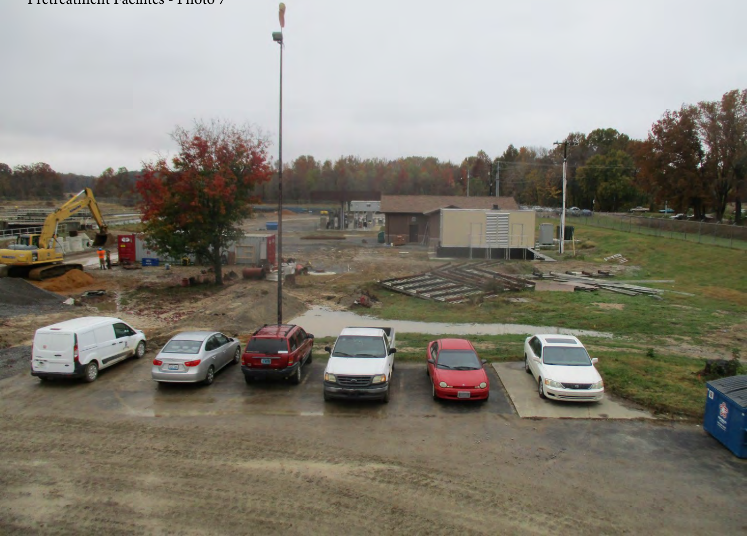
Pretreatment Facilities - Photo 7
