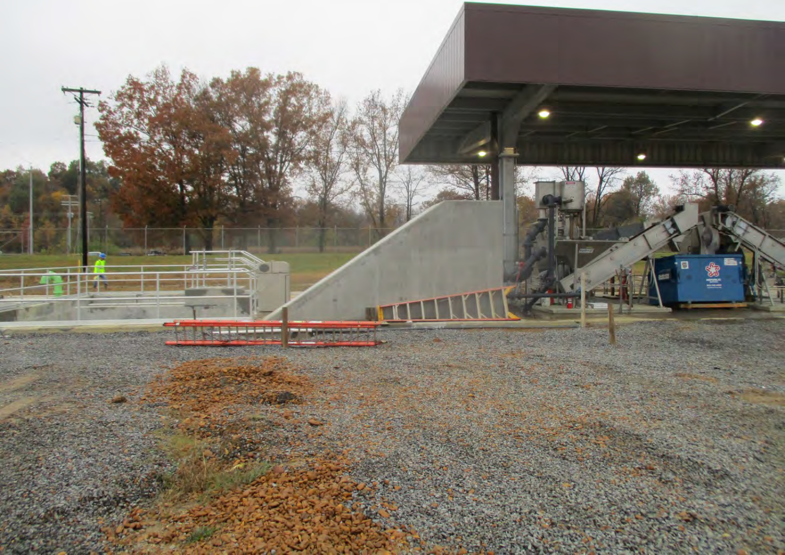
Pretreatment Facilities - Photo 5
