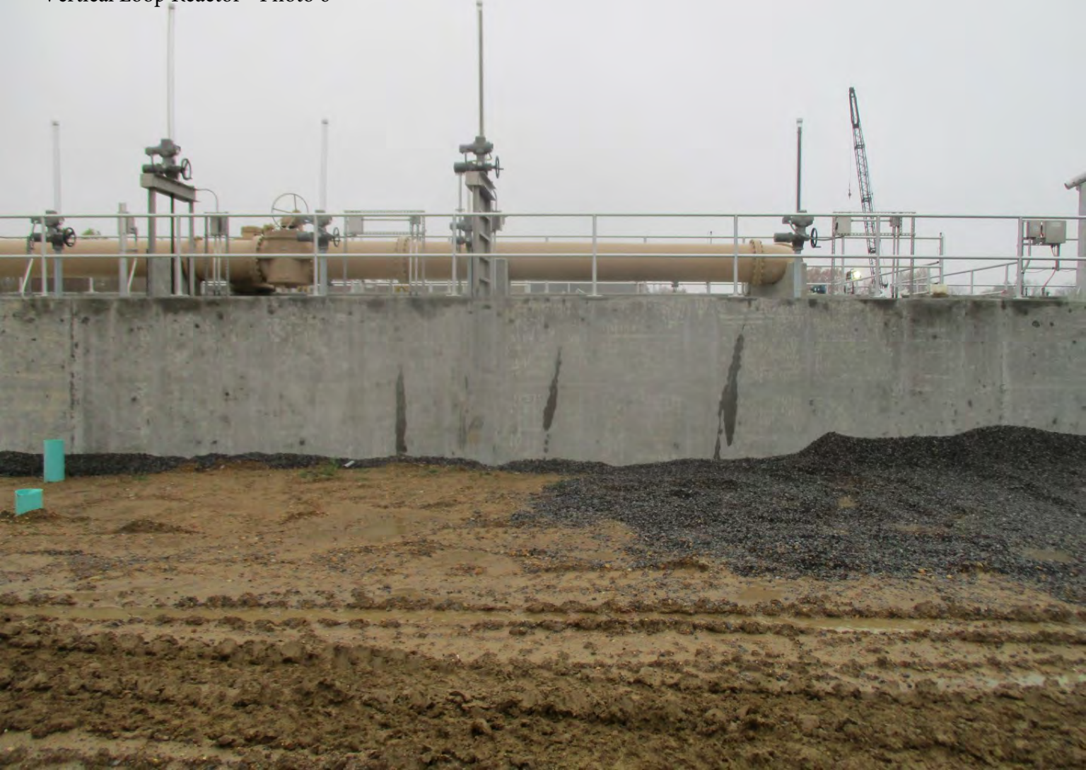
Vertical Loop Reactor - Photo 6
