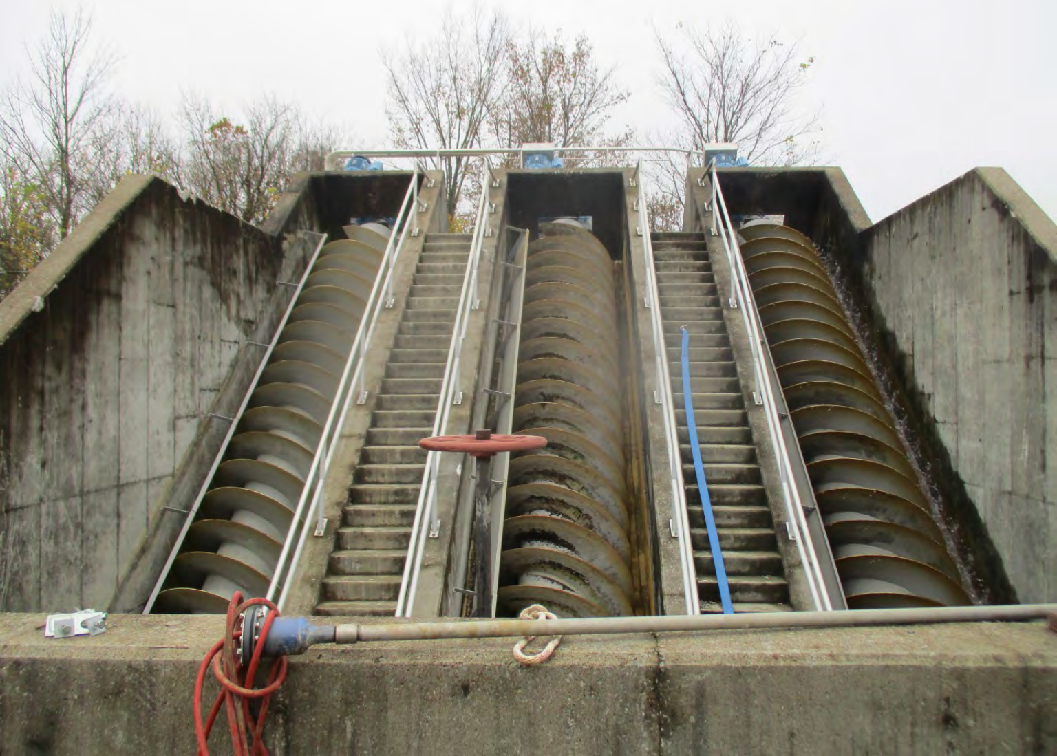
Effluent Pump Station - Photo 2
