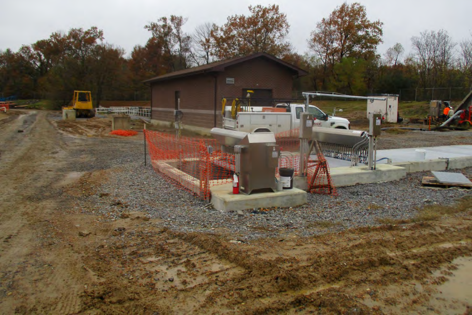
Electrical Building No. 3 - Photo 2
