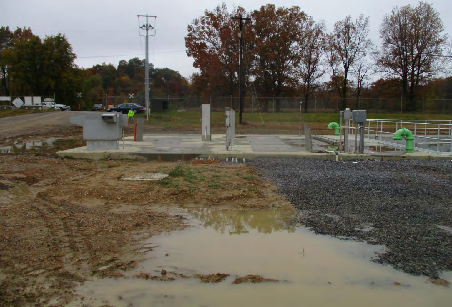
Pretreatment Facilities - Photo 4
