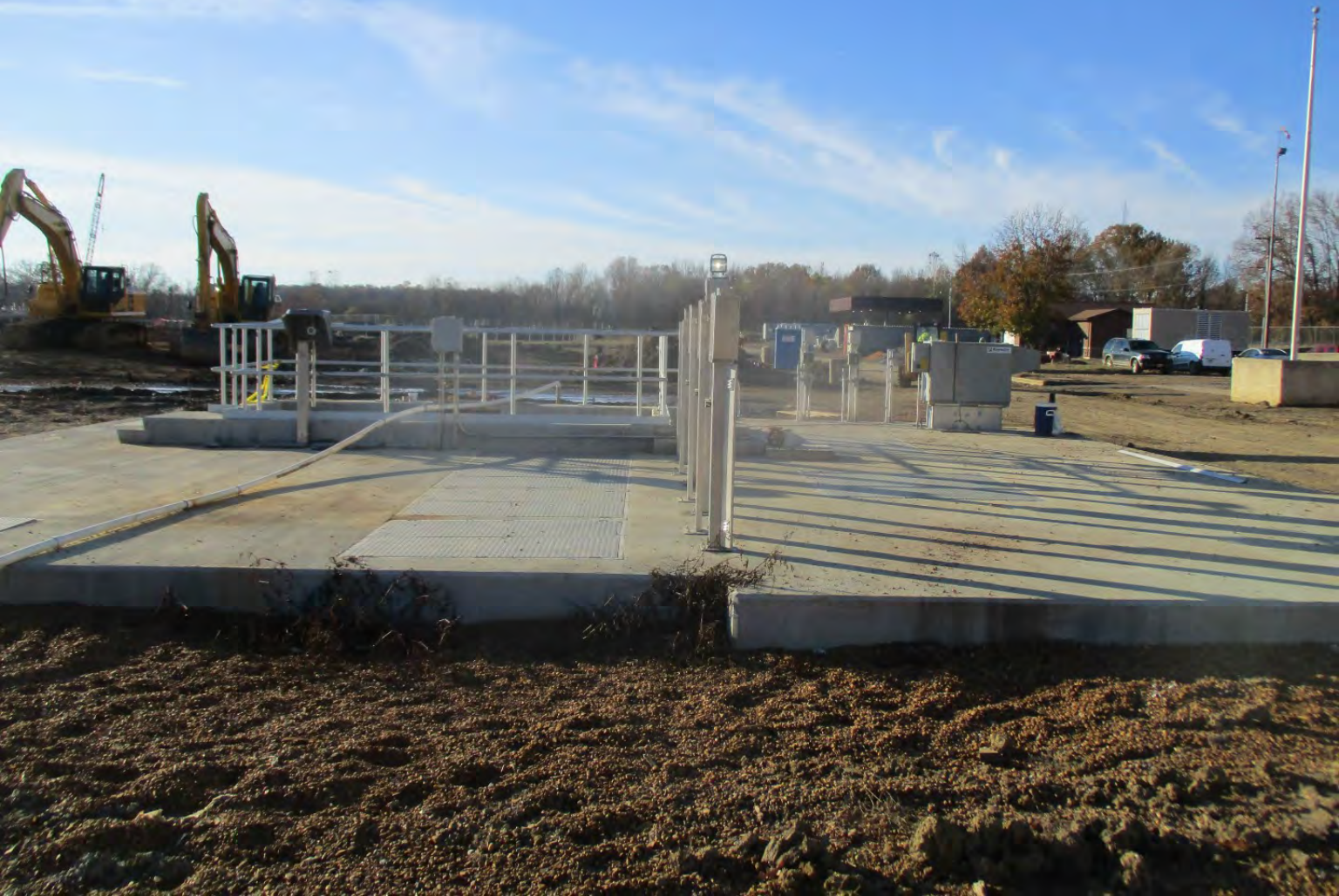
RAS Pump Station - Photo 3
