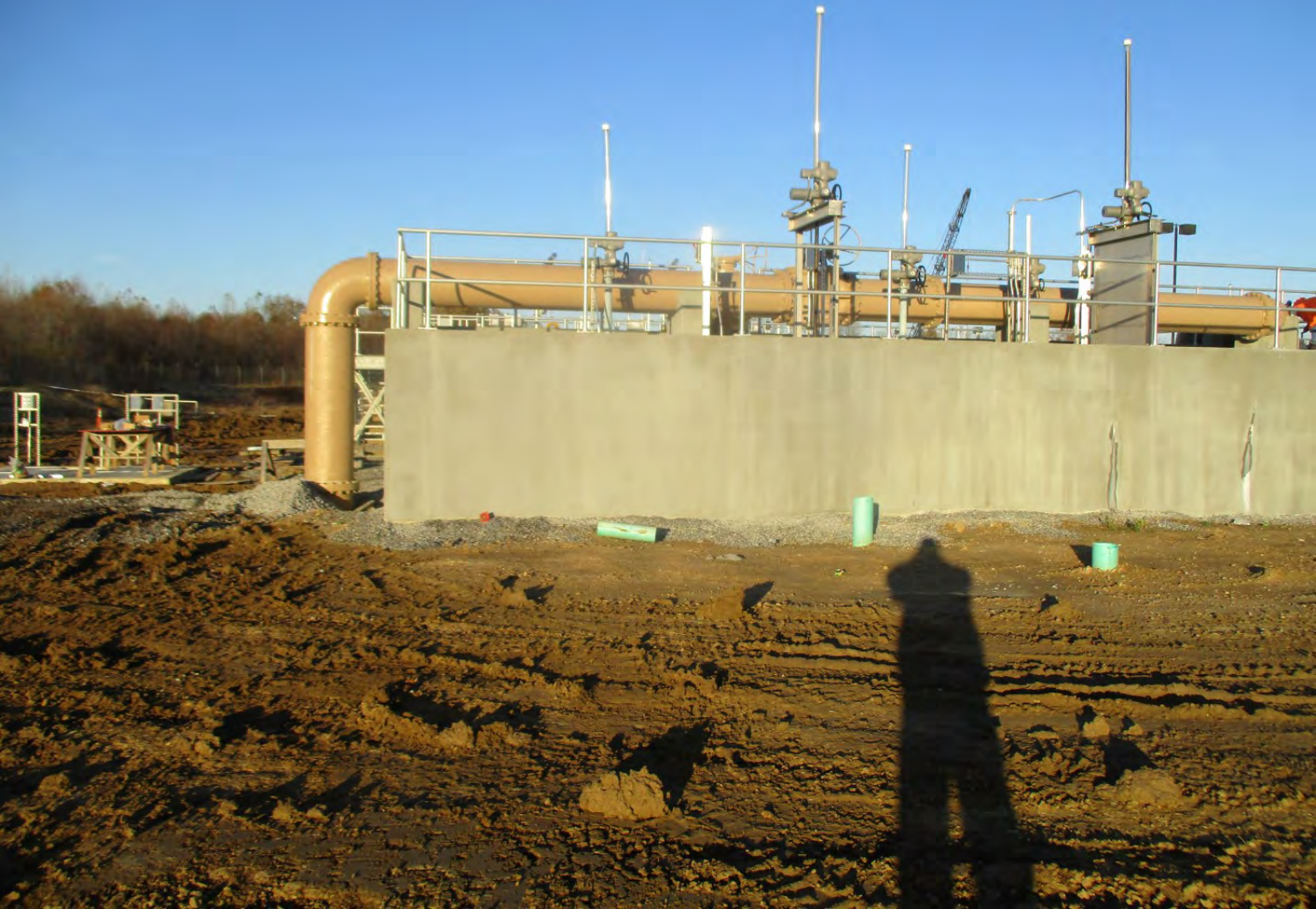
Vertical Loop Reactor - Photo 5
