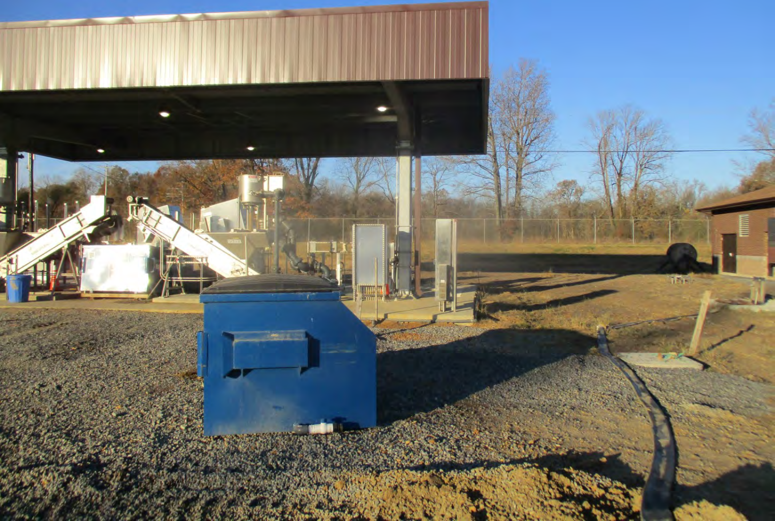
Pretreatment Facilities - Photo 6
