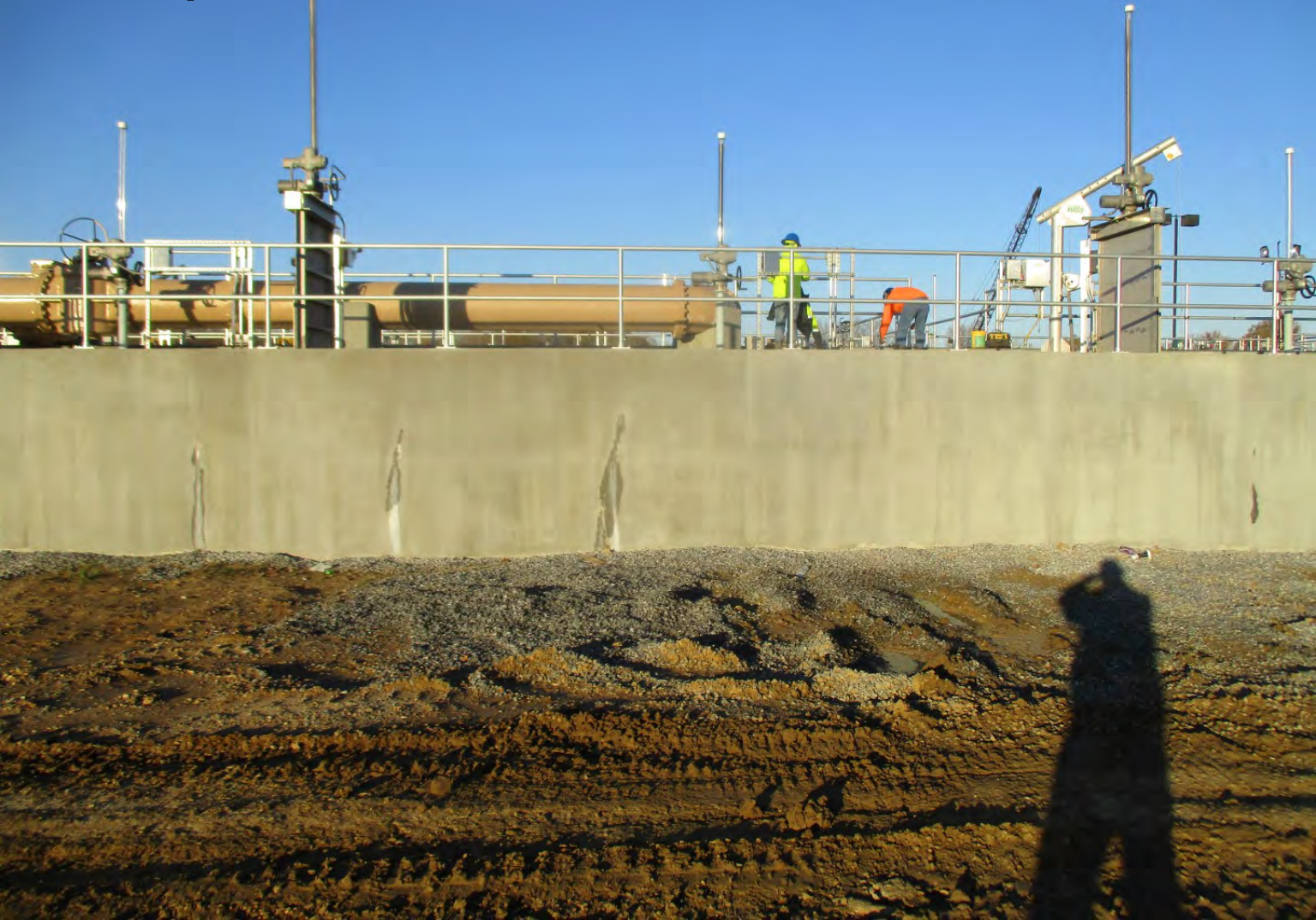
Vertical Loop Reactor - Photo 6
