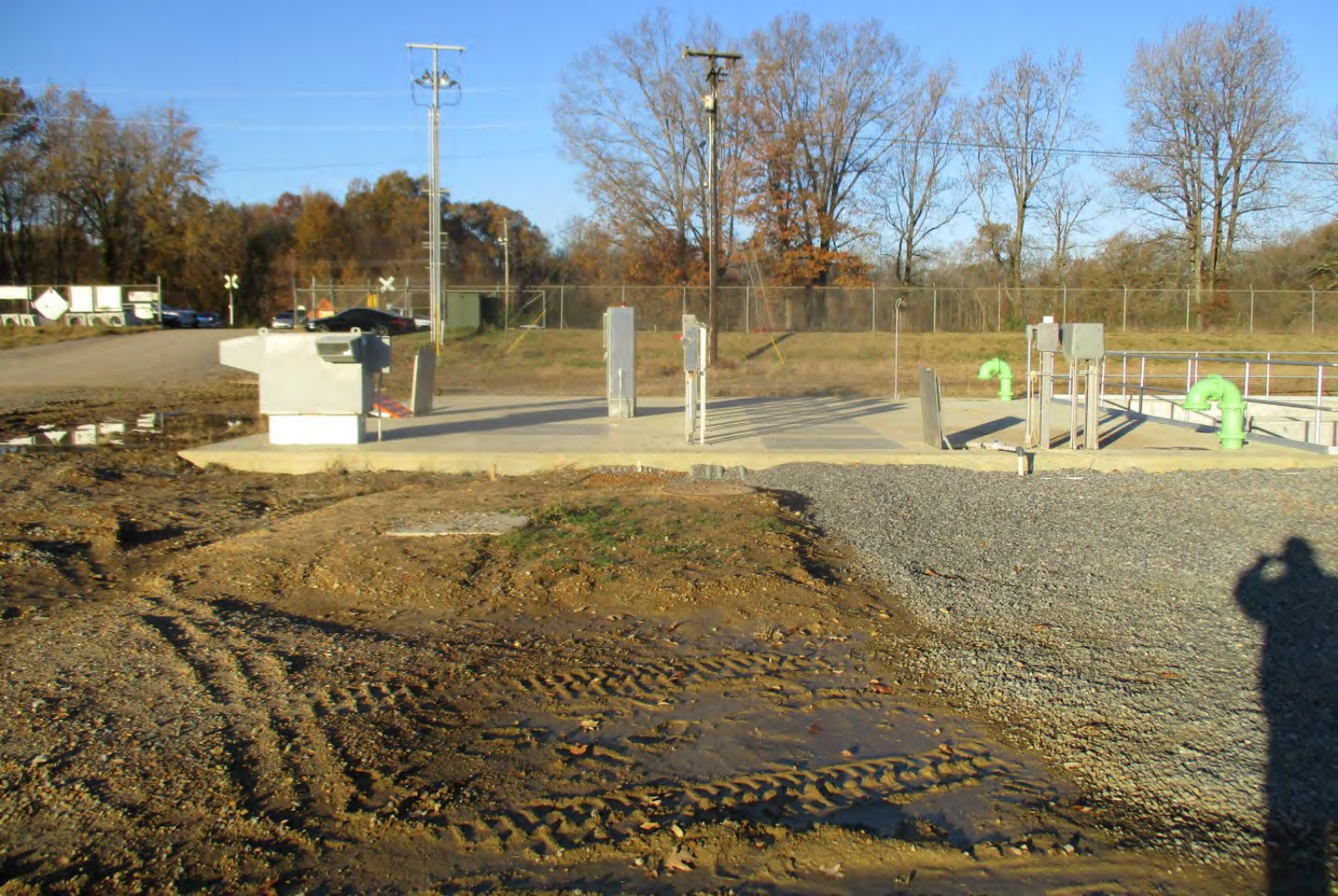
Pretreatment Facilities - Photo 4
