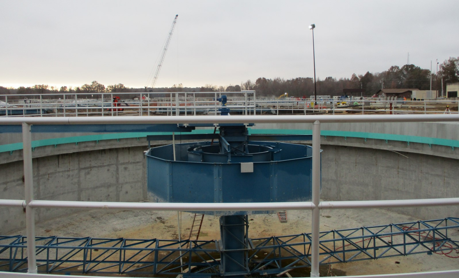
Clarifier No. 6 - Photo 2
