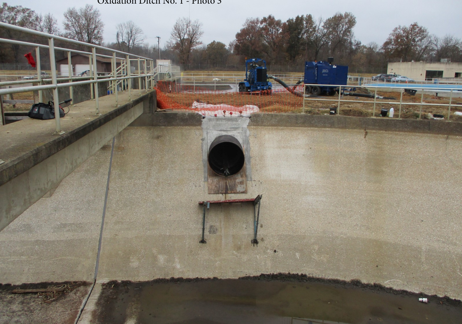
Oxidation Ditch No. 1 - Photo 3
