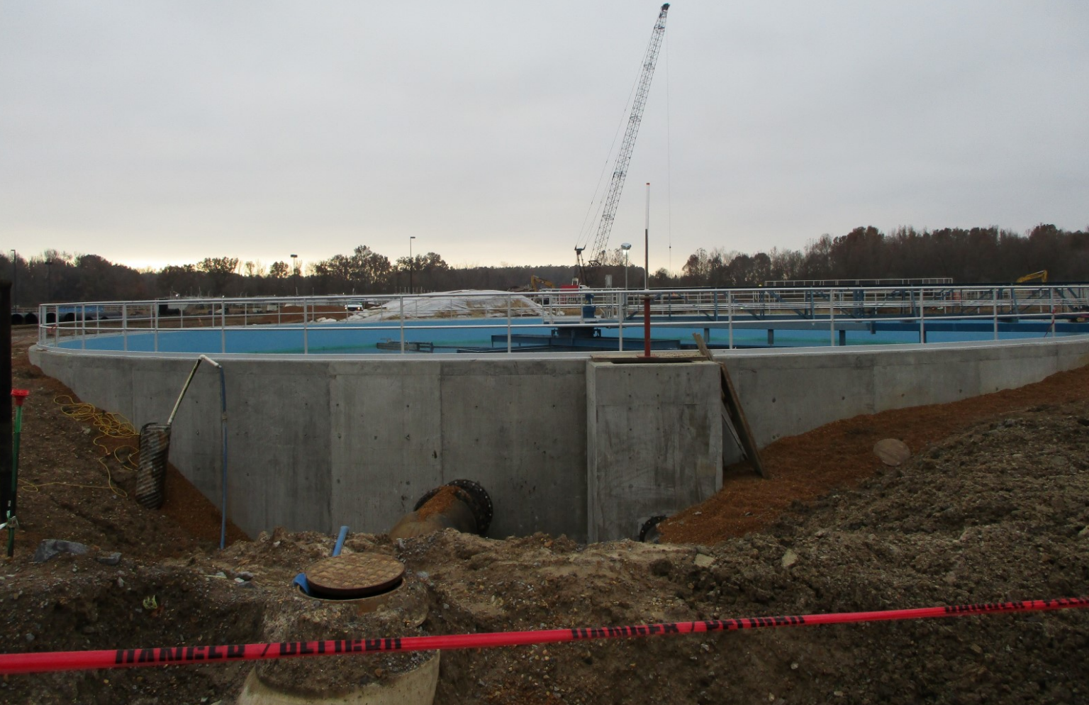
Clarifier No. 7 - Photo 1
