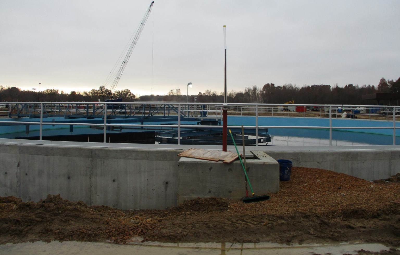
Clarifier No. 8 - Photo 2
