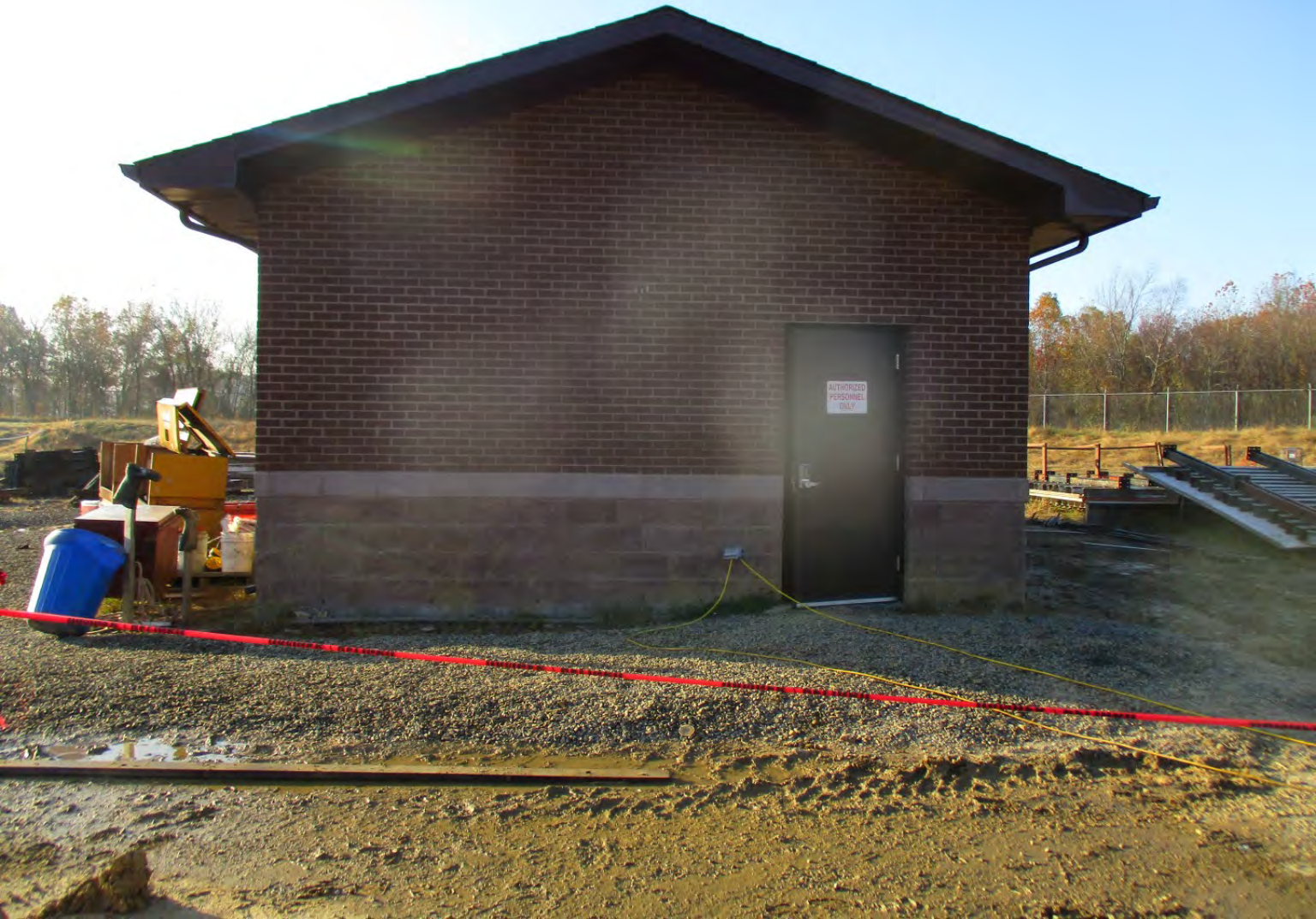
Electrical Building No. 2 - Photo 1
