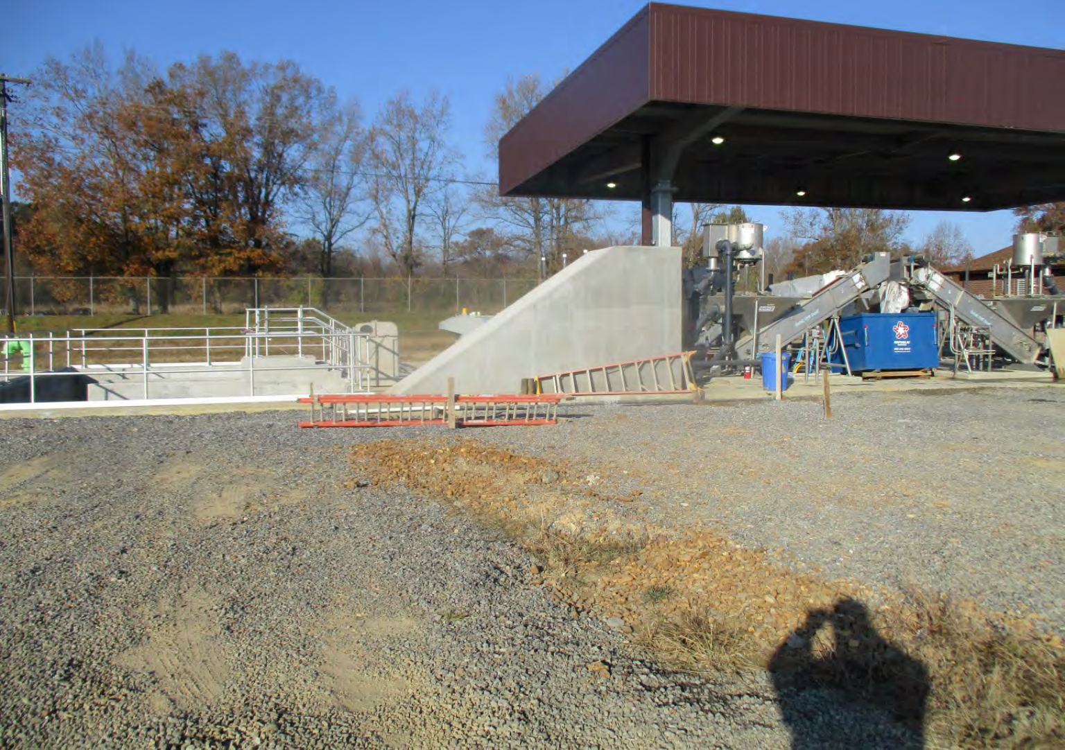
Pretreatment Facilities - Photo 5
