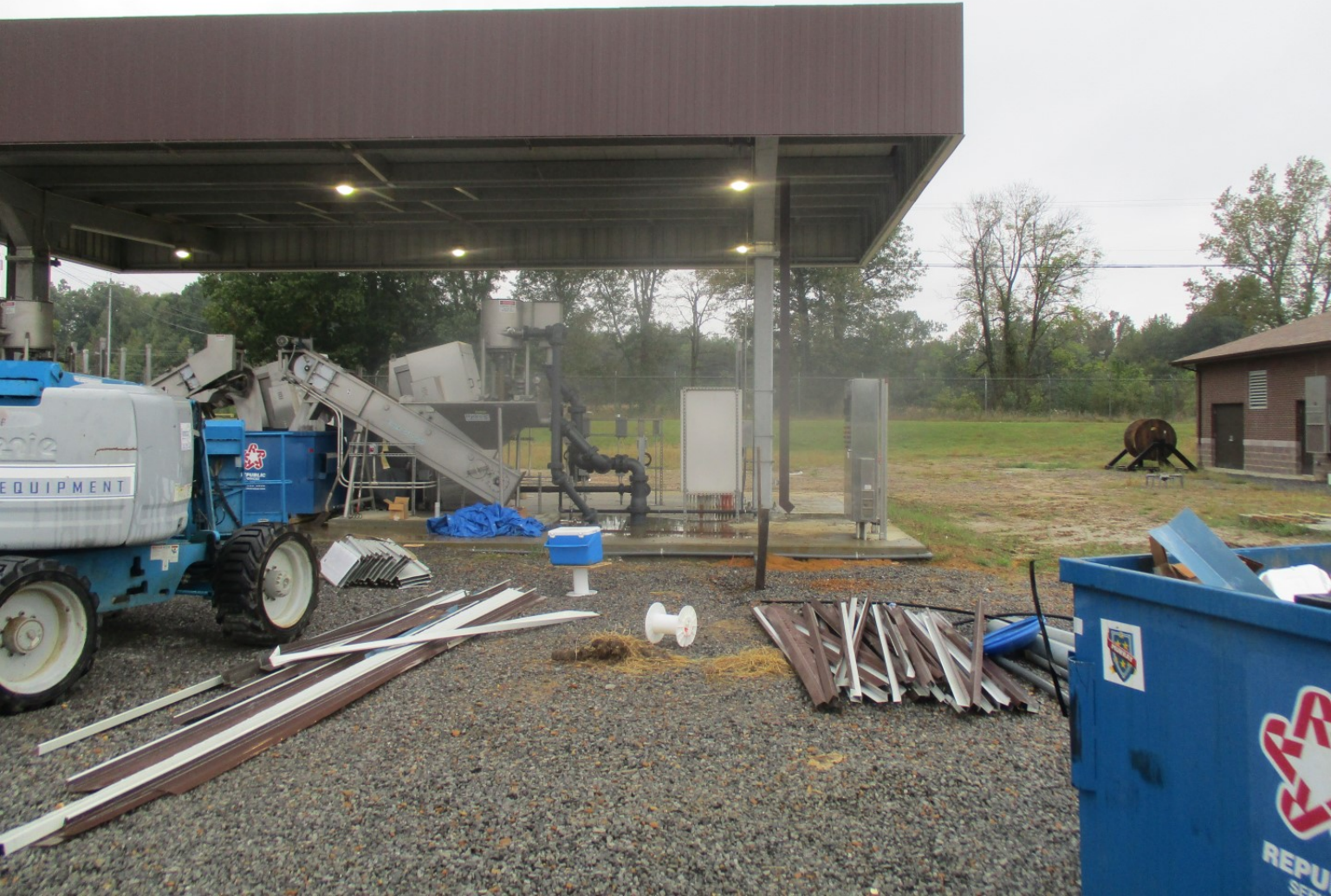
Pretreatment Facilities - Photo 6
