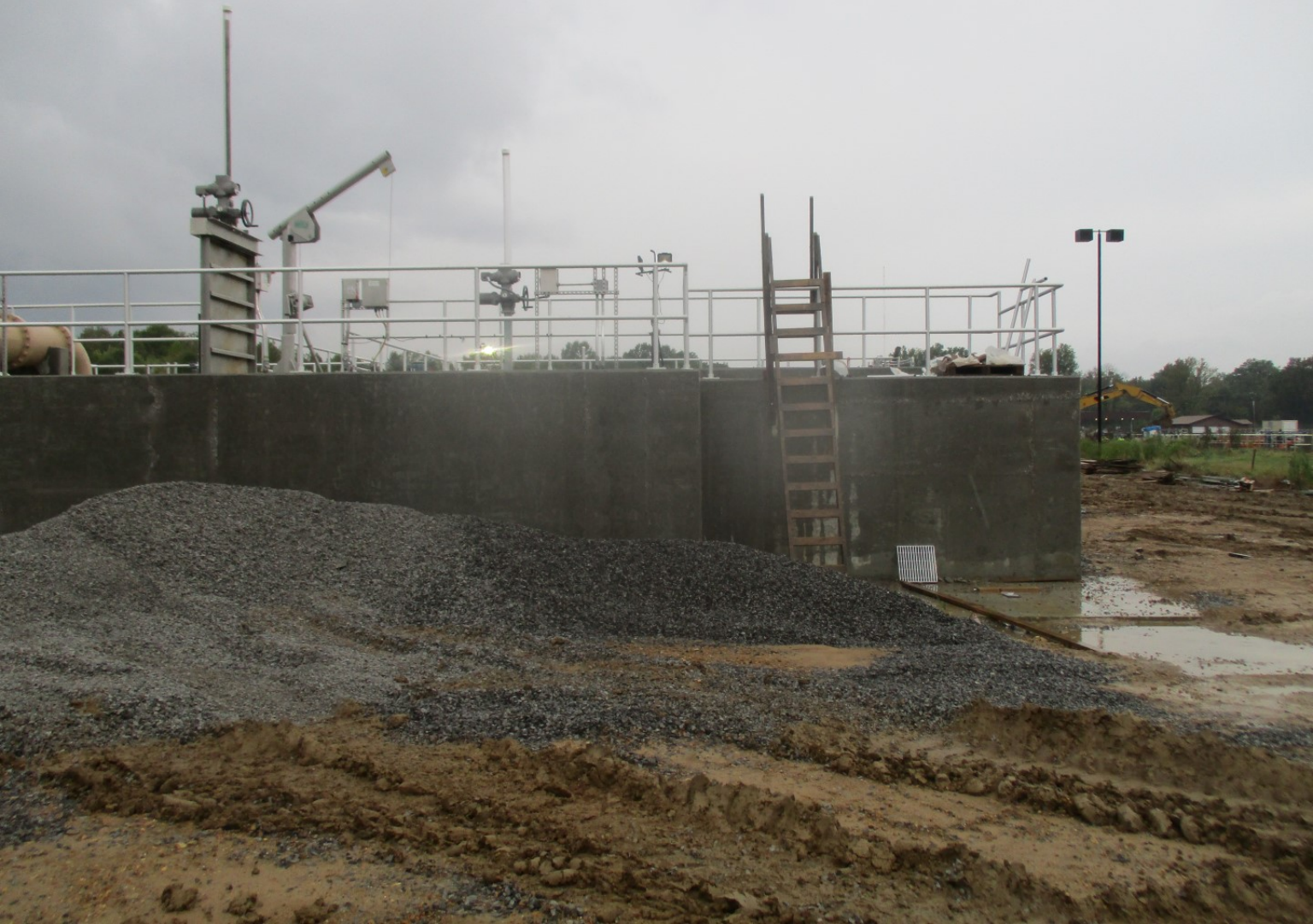
Vertical Loop Reactor - Photo 7
