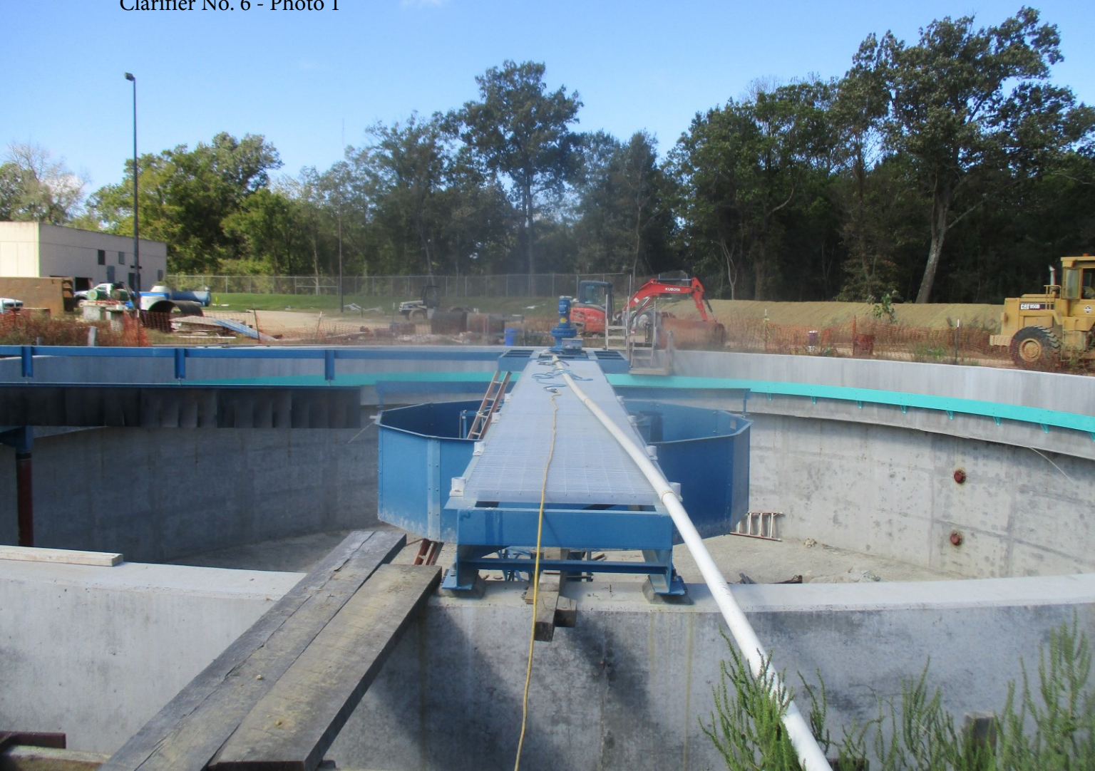
Clarifier No. 6 - Photo 1
