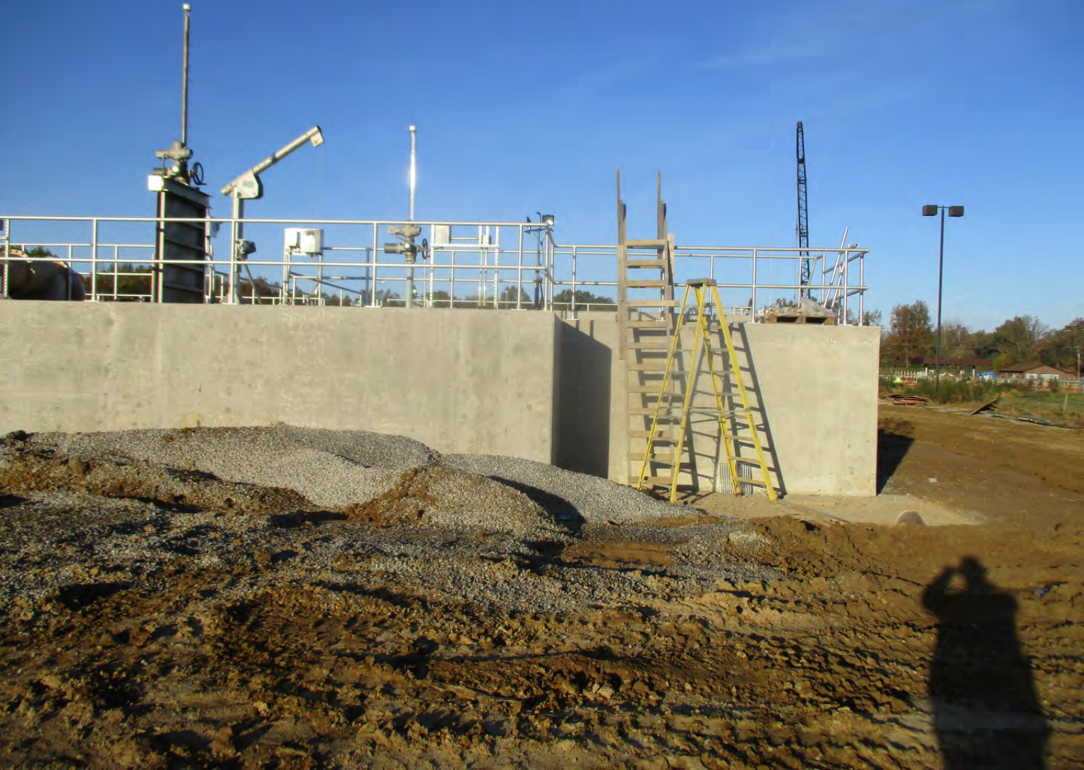
Vertical Loop Reactor - Photo 7
