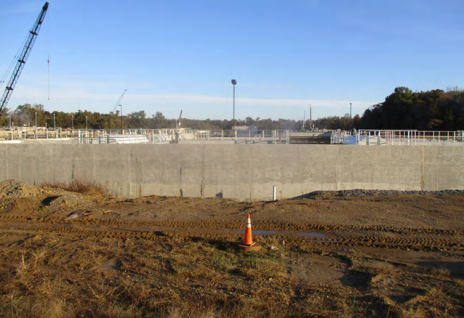
Vertical Loop Reactor - Photo 4
