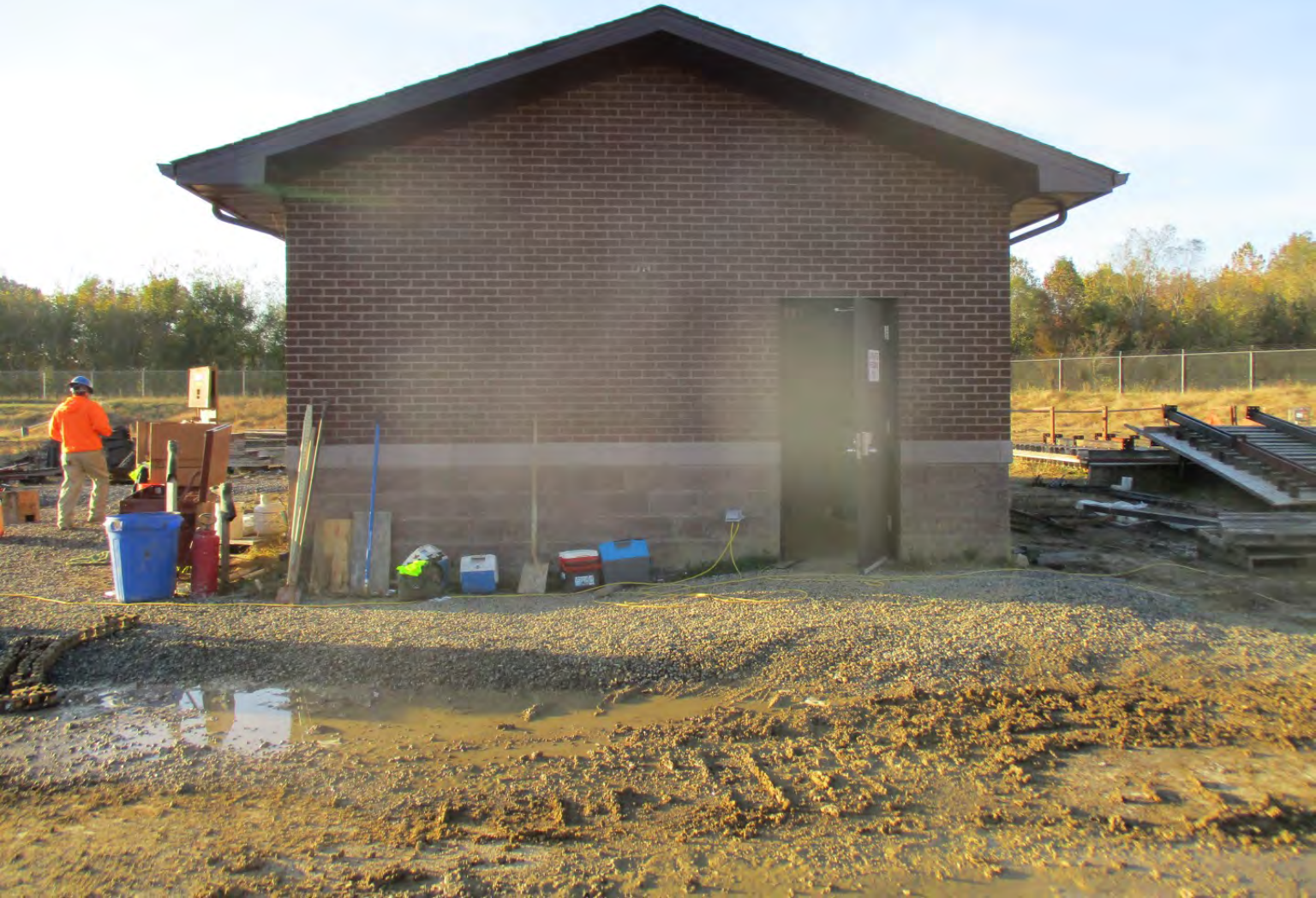
Electrical Building No. 2 - Photo 1
