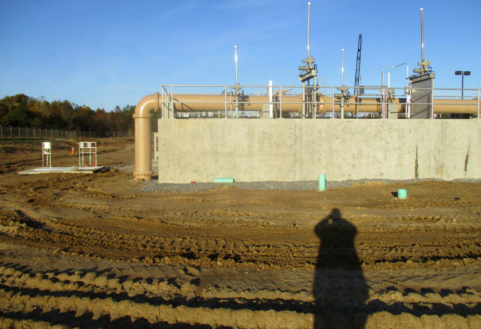
Vertical Loop Reactor - Photo 5
