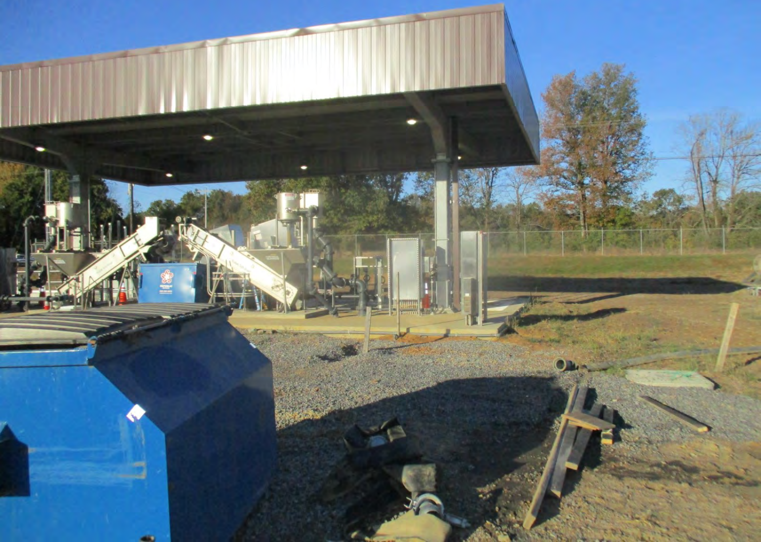
Pretreatment Facilities - Photo 6
