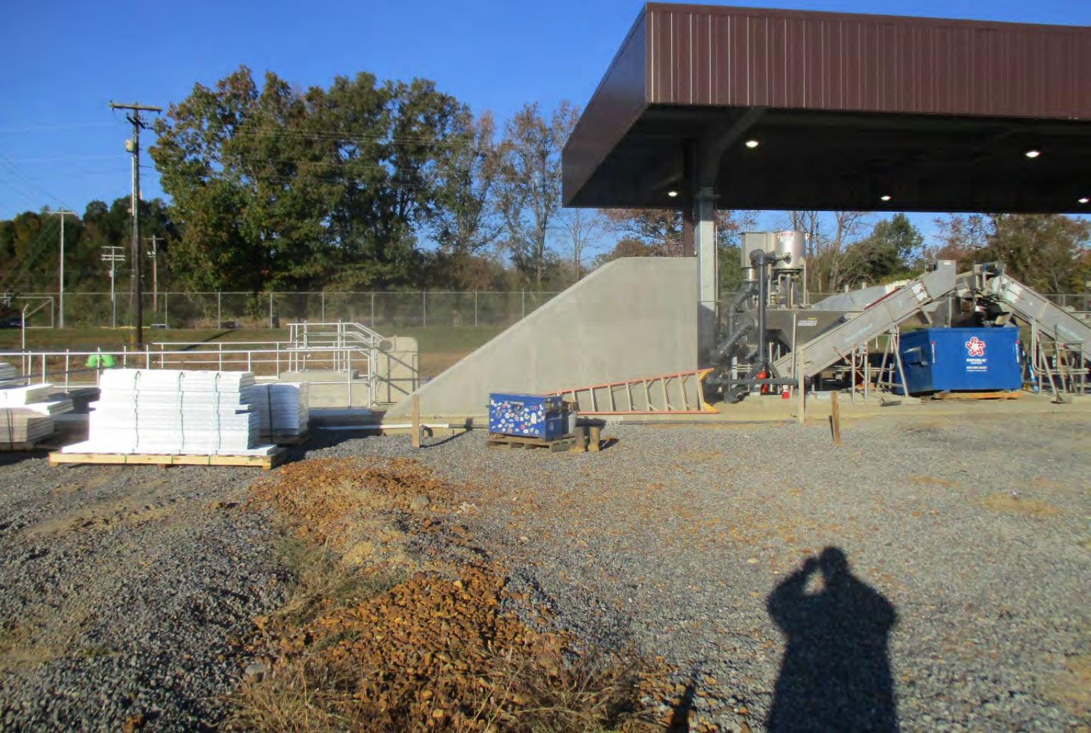
Pretreatment Facilities - Photo 5
