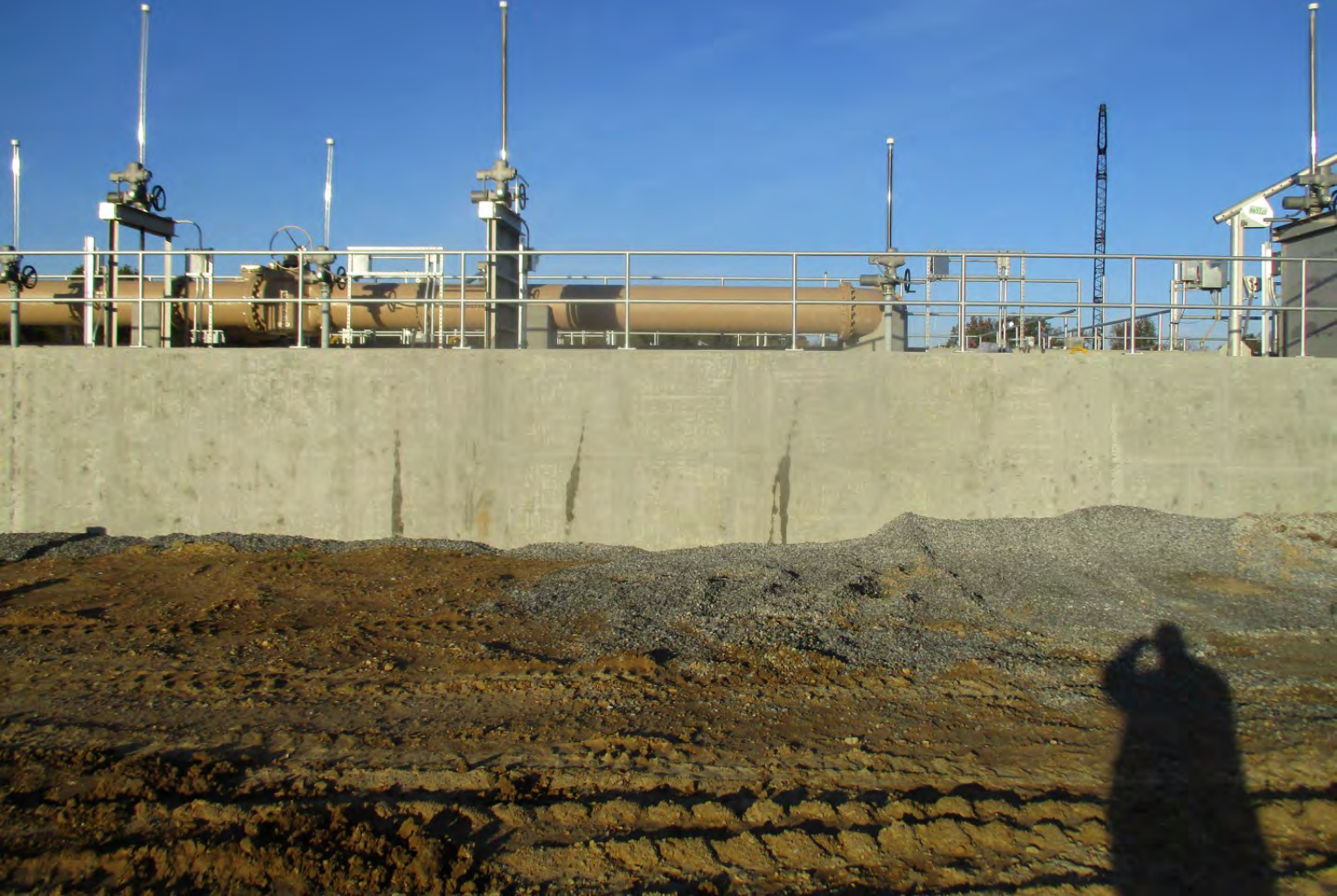
Vertical Loop Reactor - Photo 6
