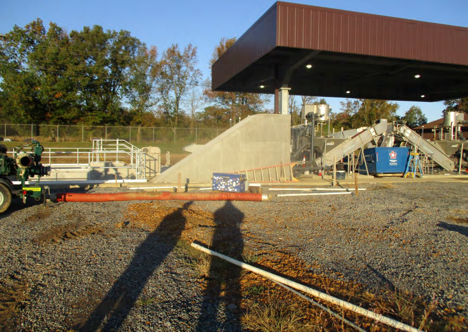
Pretreatment Facilities - Photo 5
