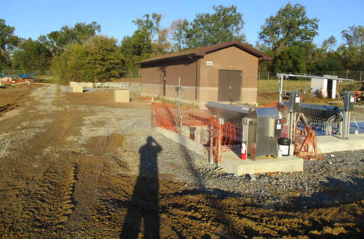
Electrical Building No. 3 - Photo 2
