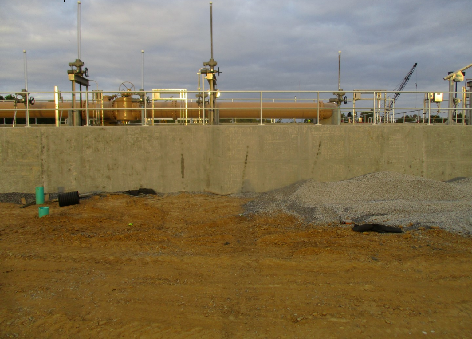
Vertical Loop Reactor - Photo 6
