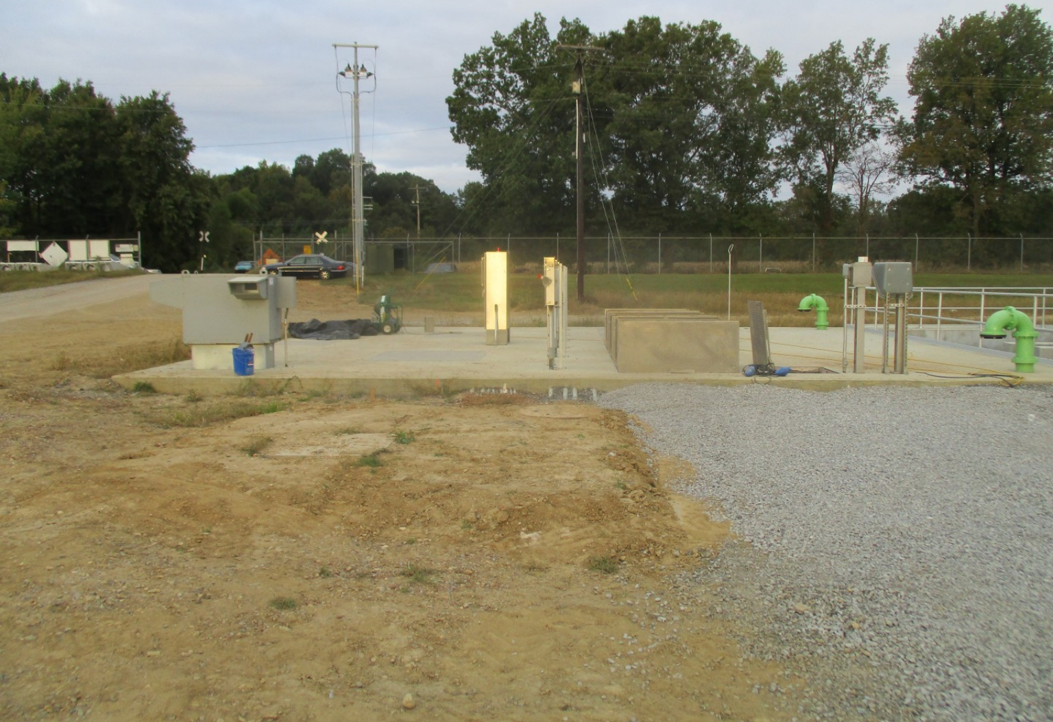
Pretreatment Facilities - Photo 4
