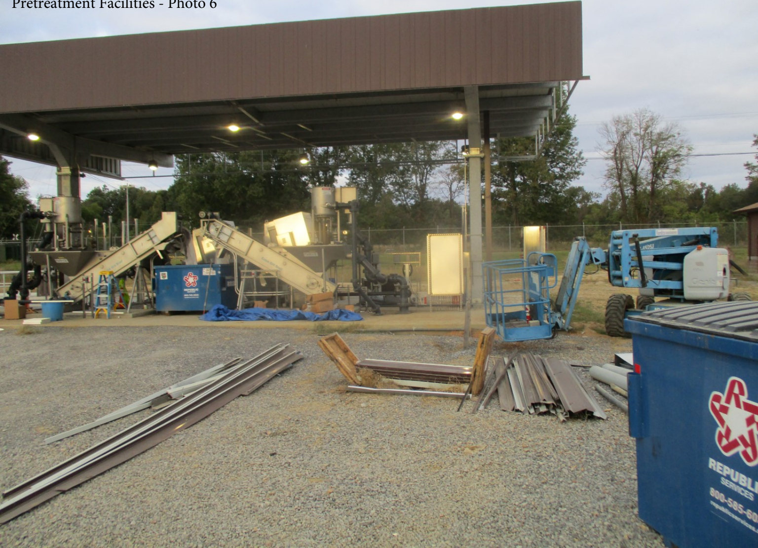
Pretreatment Facilities - Photo 6
