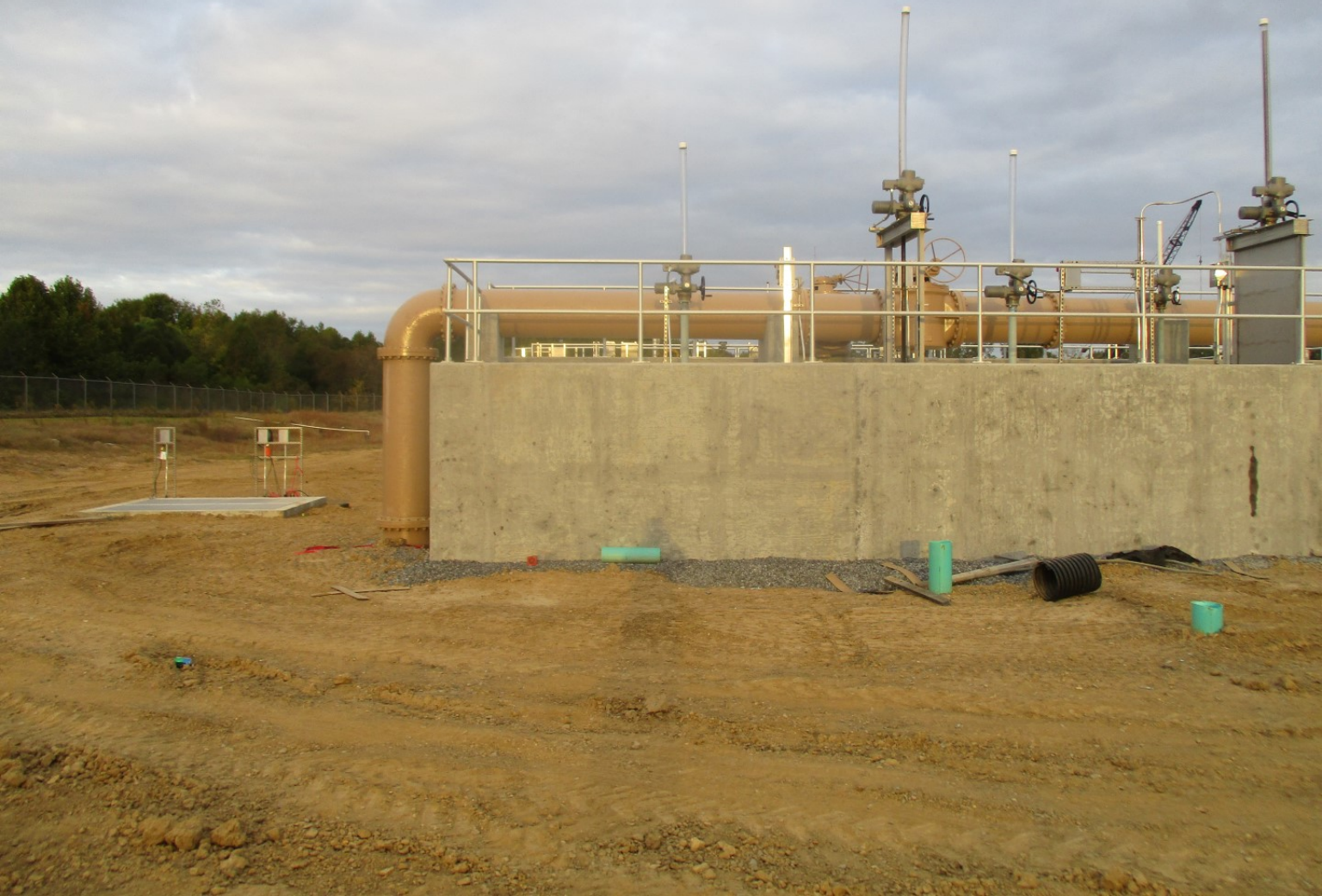
Vertical Loop Reactor - Photo 5
