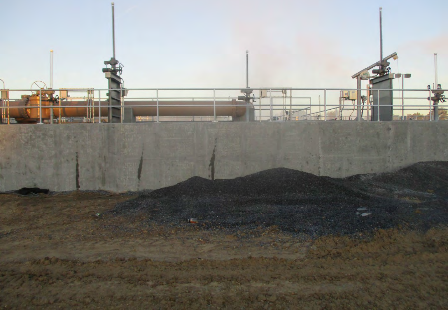
Vertical Loop Reactor - Photo 6
