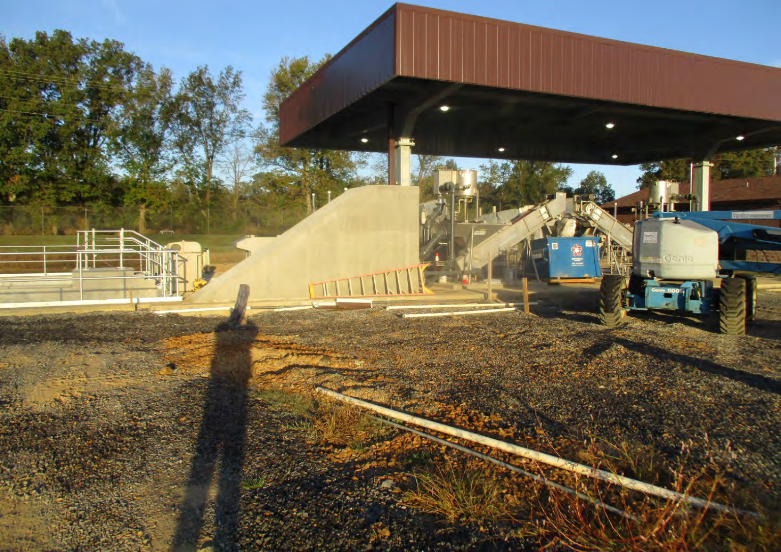
Pretreatment Facilities - Photo 5
