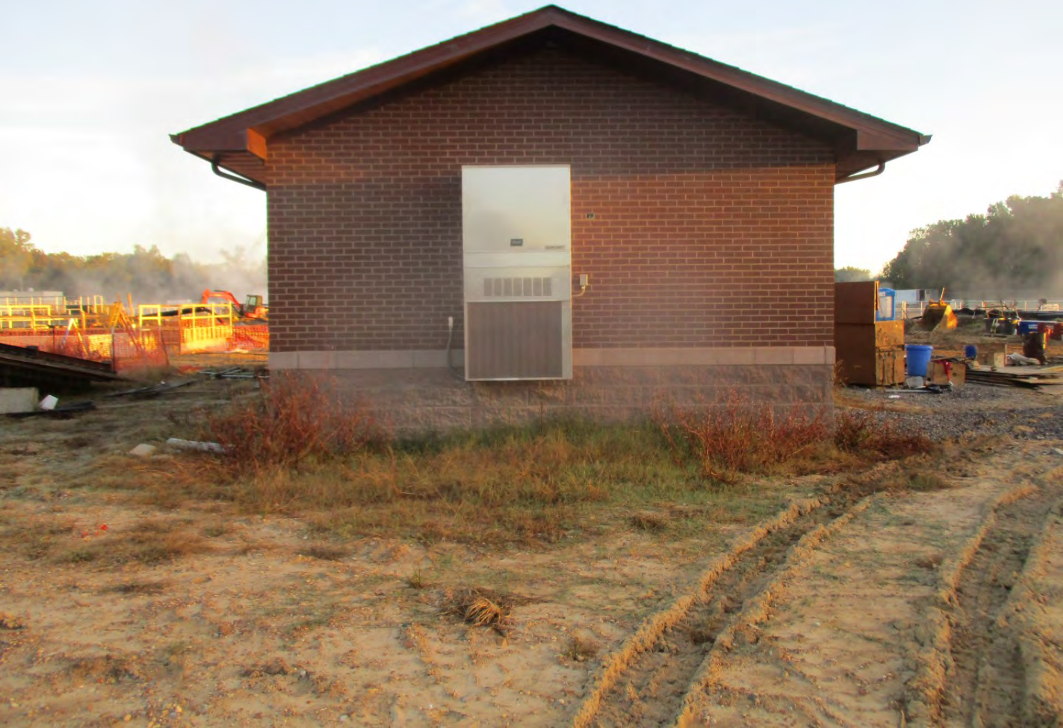
Electrical Building No. 2 - Photo 2
