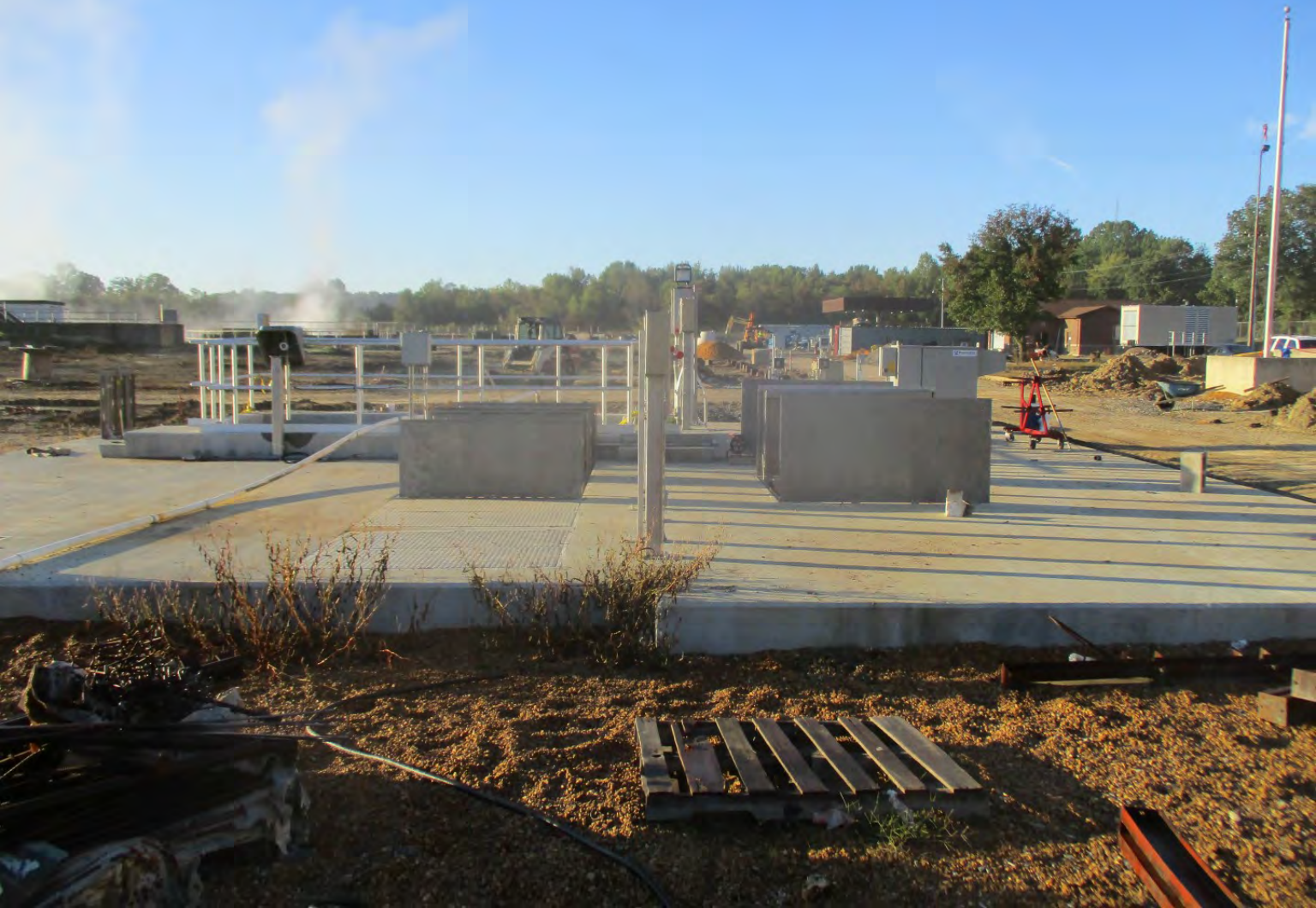
RAS Pump Station - Photo 3
