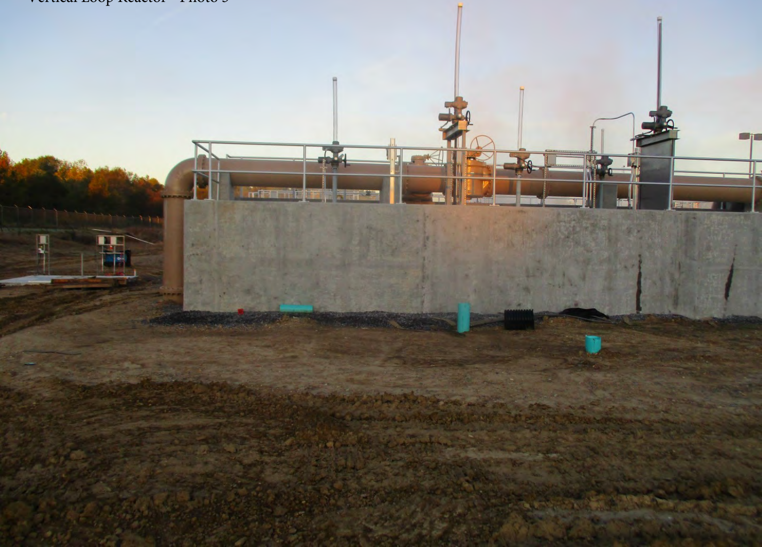
Vertical Loop Reactor - Photo 5
