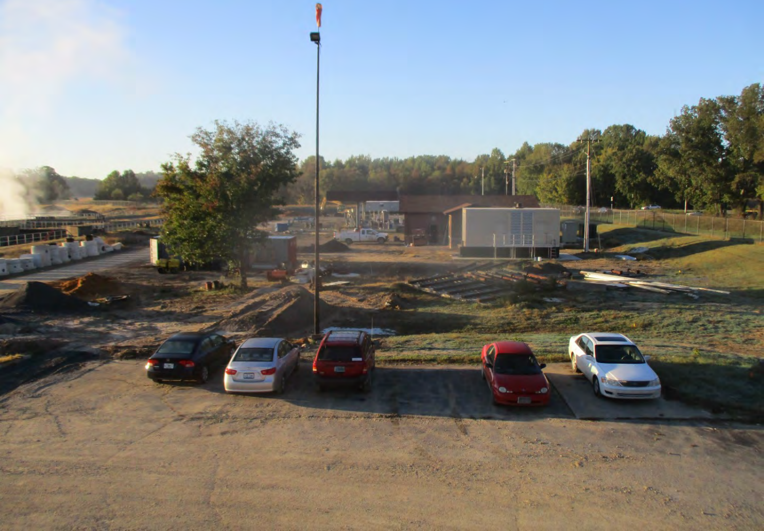
Pretreatment Facilities - Photo 7
