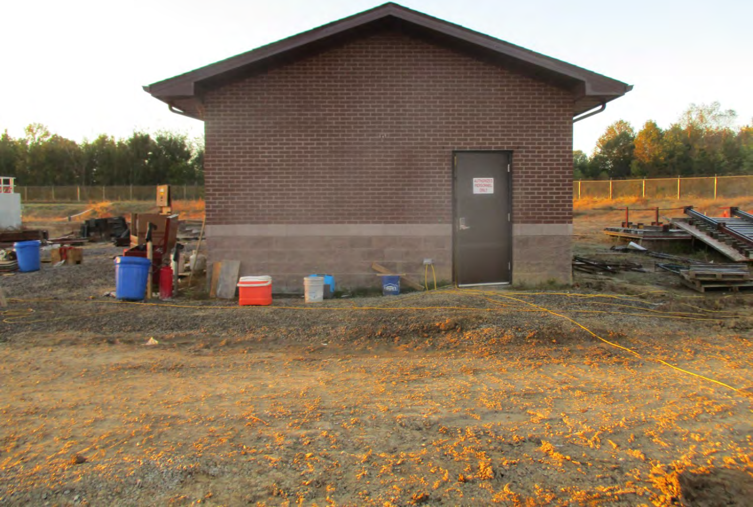
Electrical Building No. 2 - Photo 1
