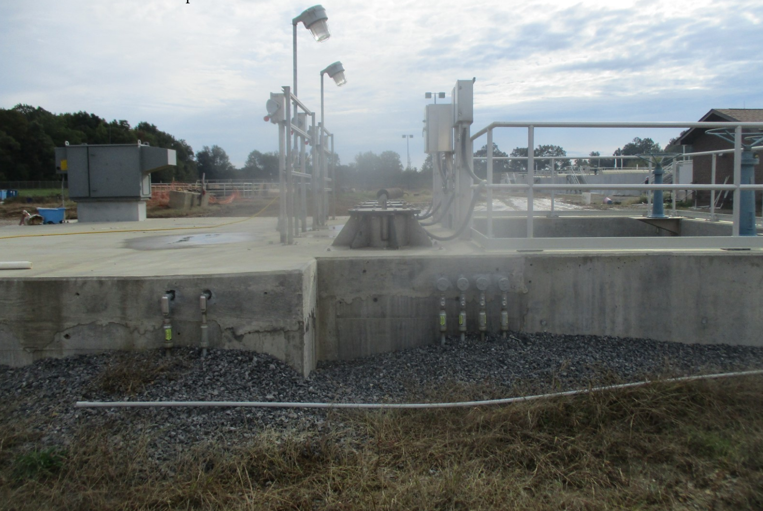
Nitrate Pump Station - Photo 3
