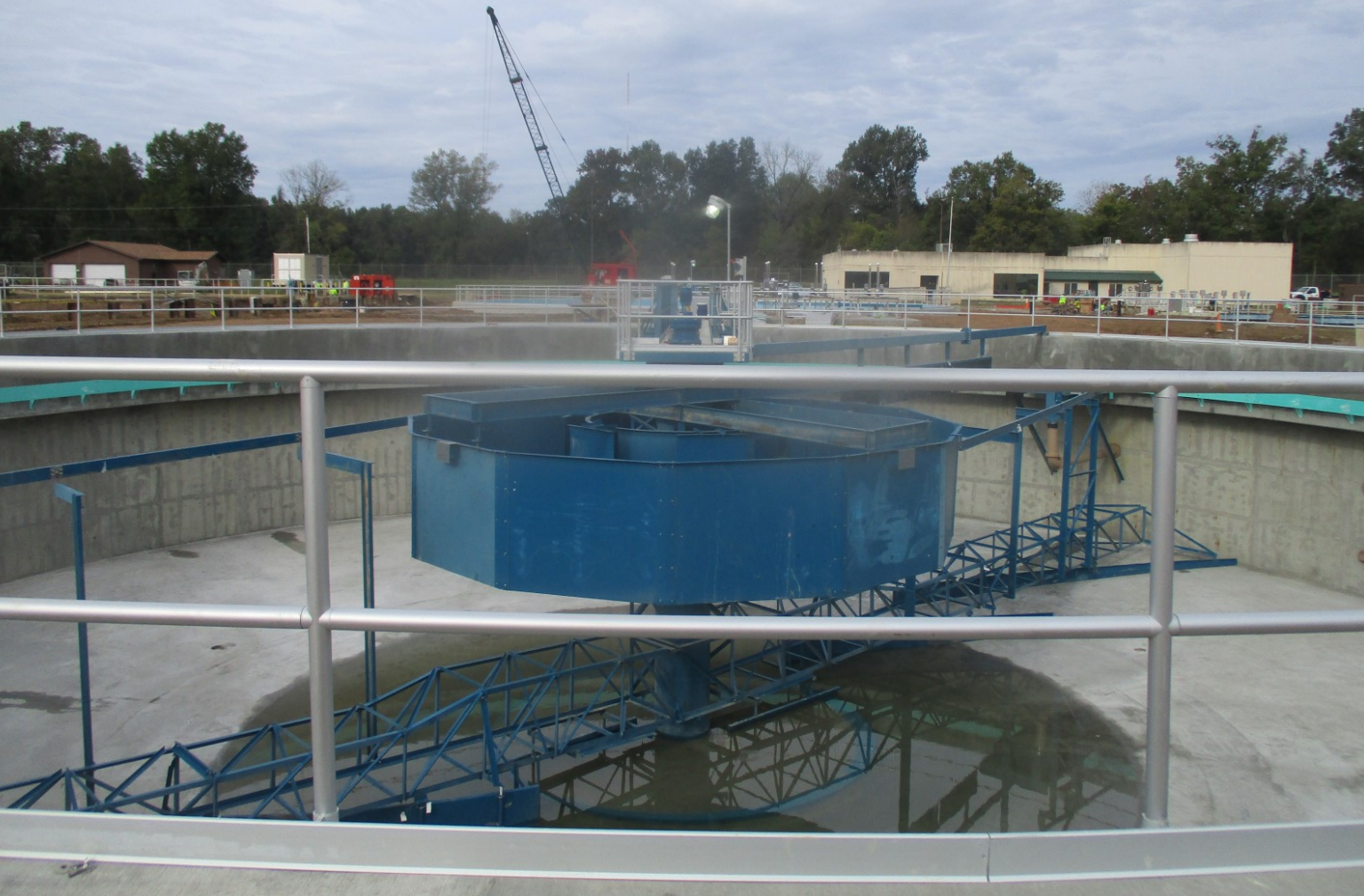
Clarifier No. 7 - Photo 2
