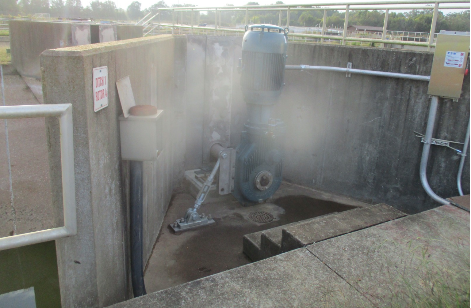
Oxidation Ditch No. 1 - Photo 4
