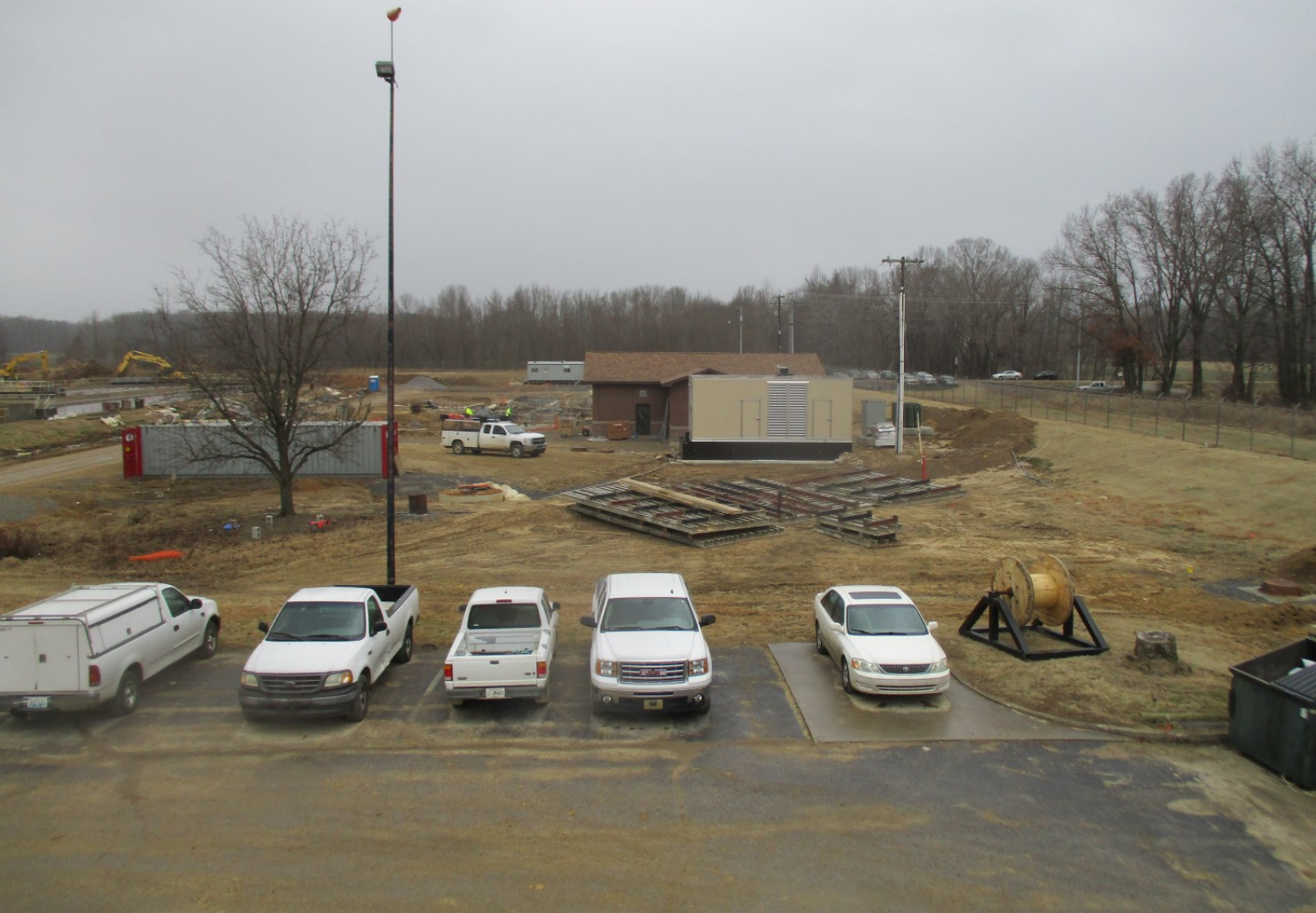
Pretreatment Facilities - Photo 7
