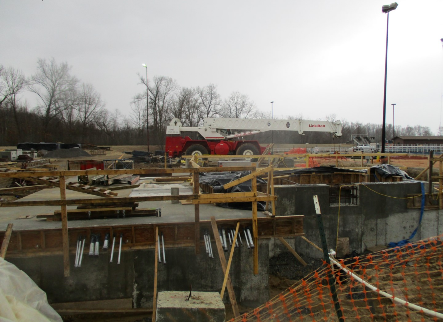
RAS Pump Station - Photo 2
