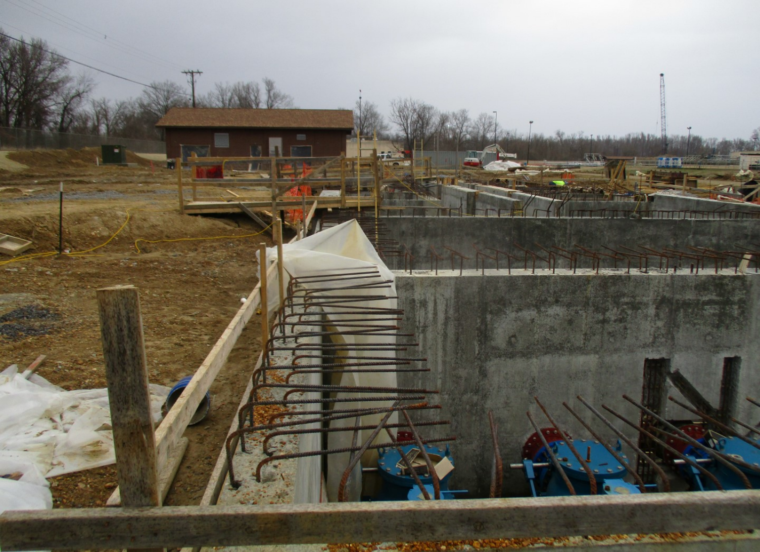
Pretreatment Facilities - Photo 1
