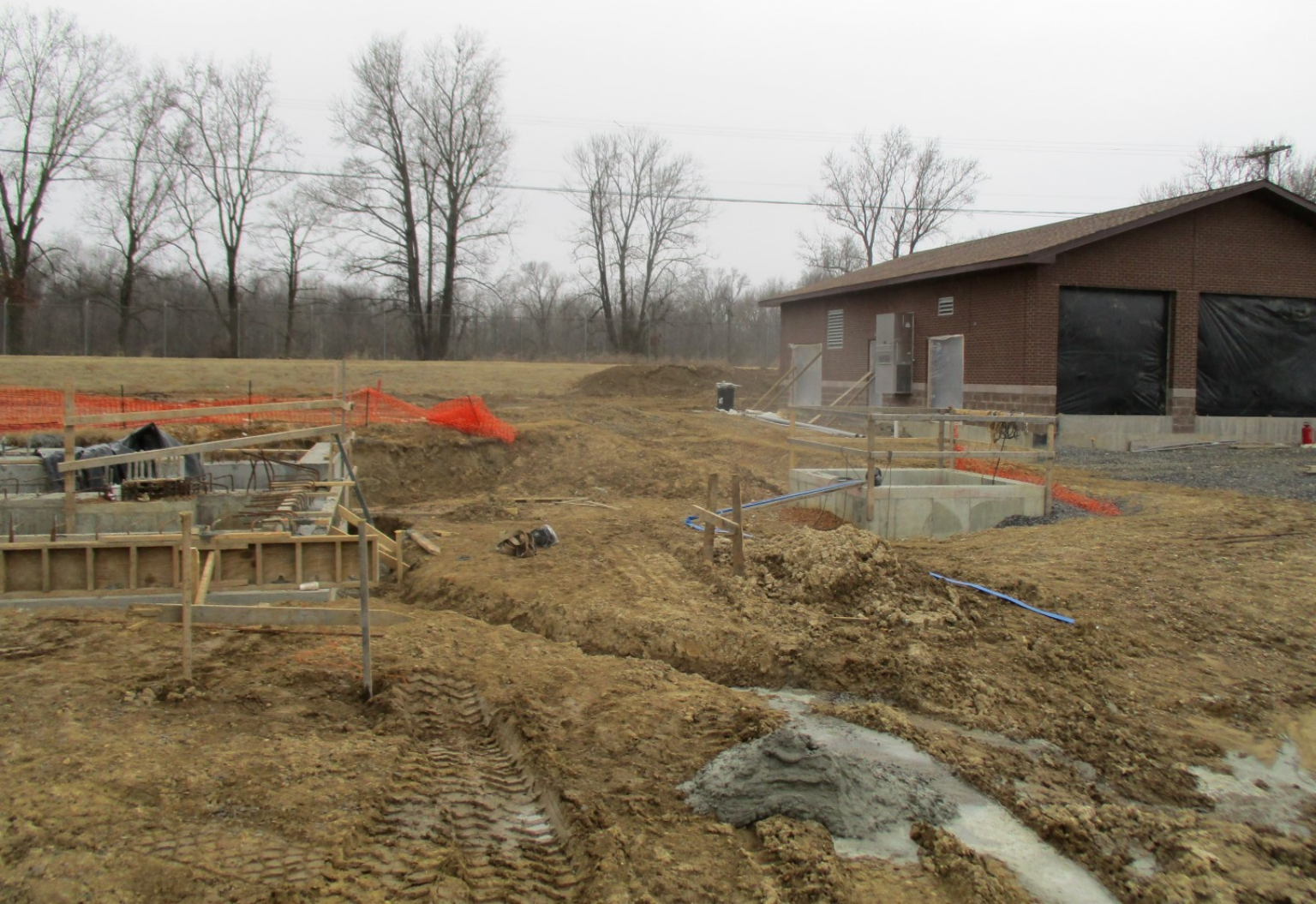
Pretreatment Facilities - Photo 6
