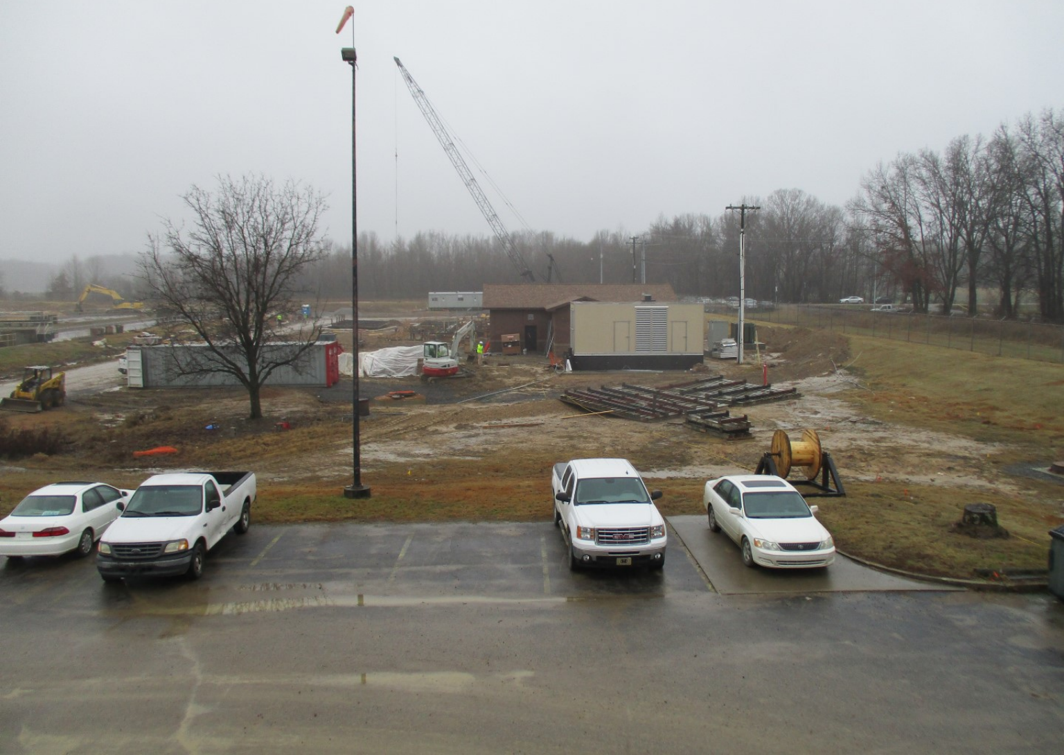
Pretreatment Facilities - Photo 7
