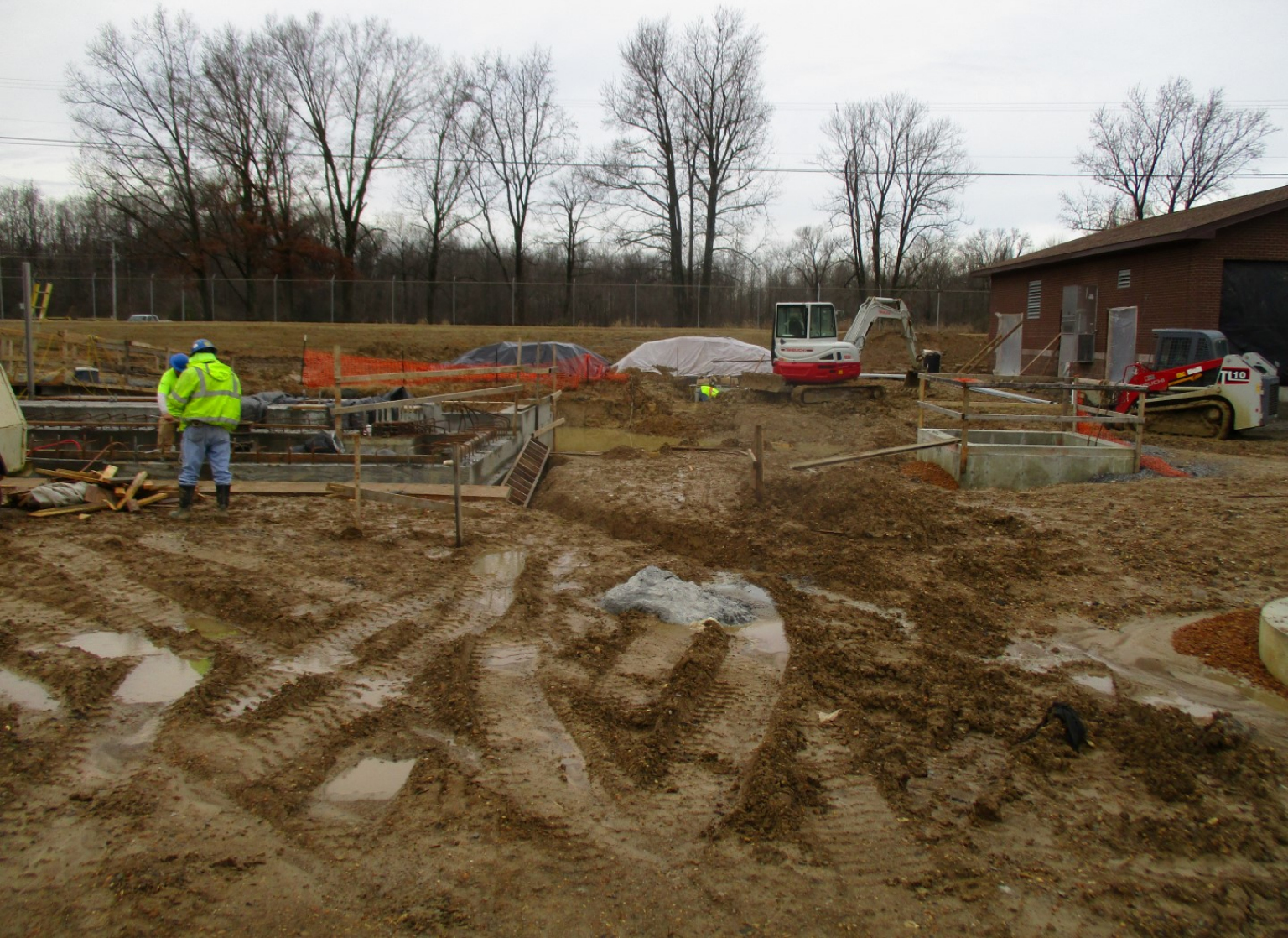
Pretreatment Facilities - Photo 6
