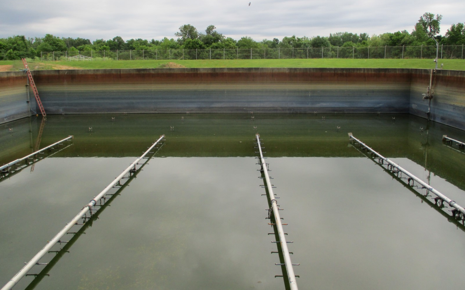
Interchange Tank - Photo 2
