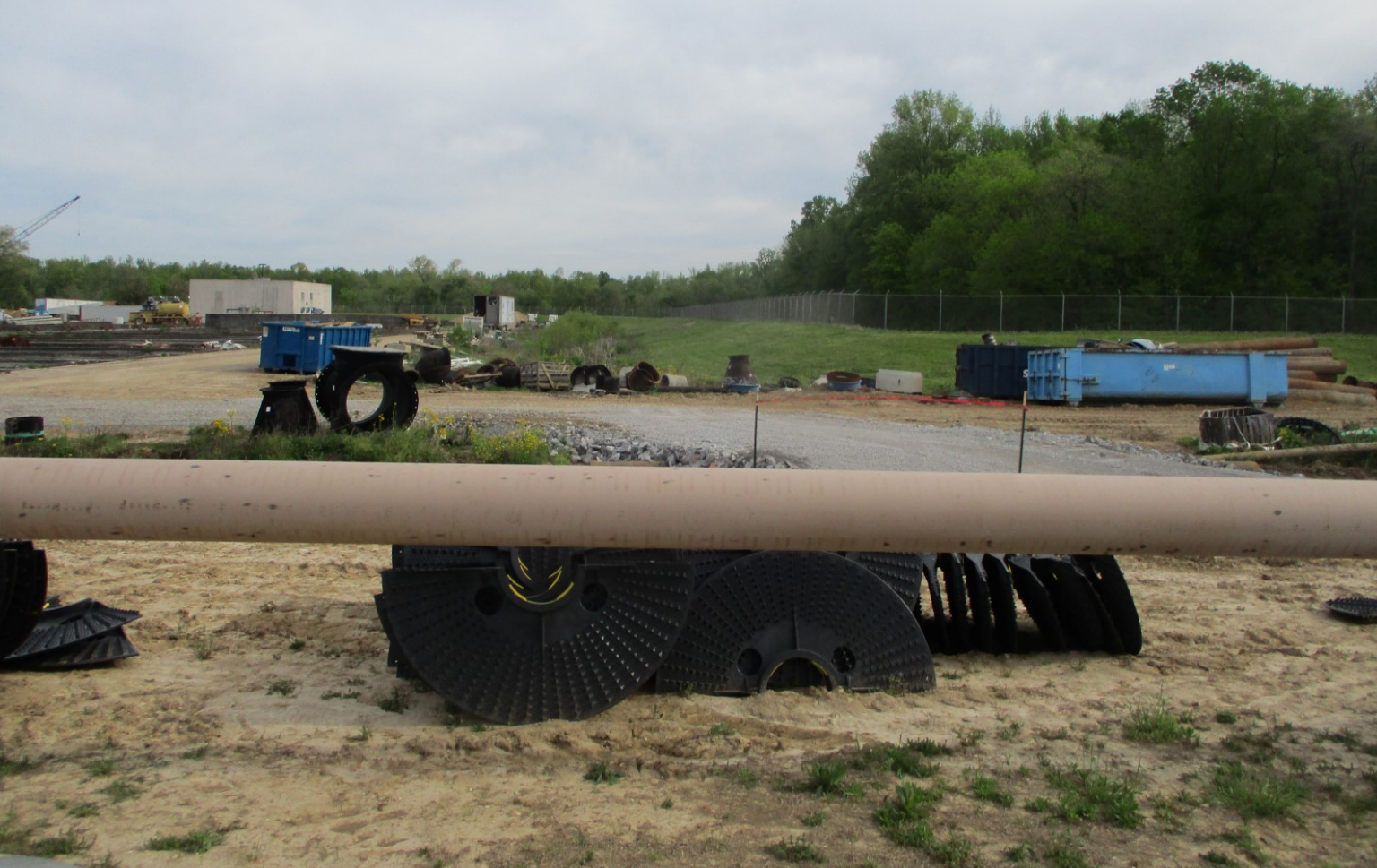
Oxidation Ditch No. 3 - Photo 2
