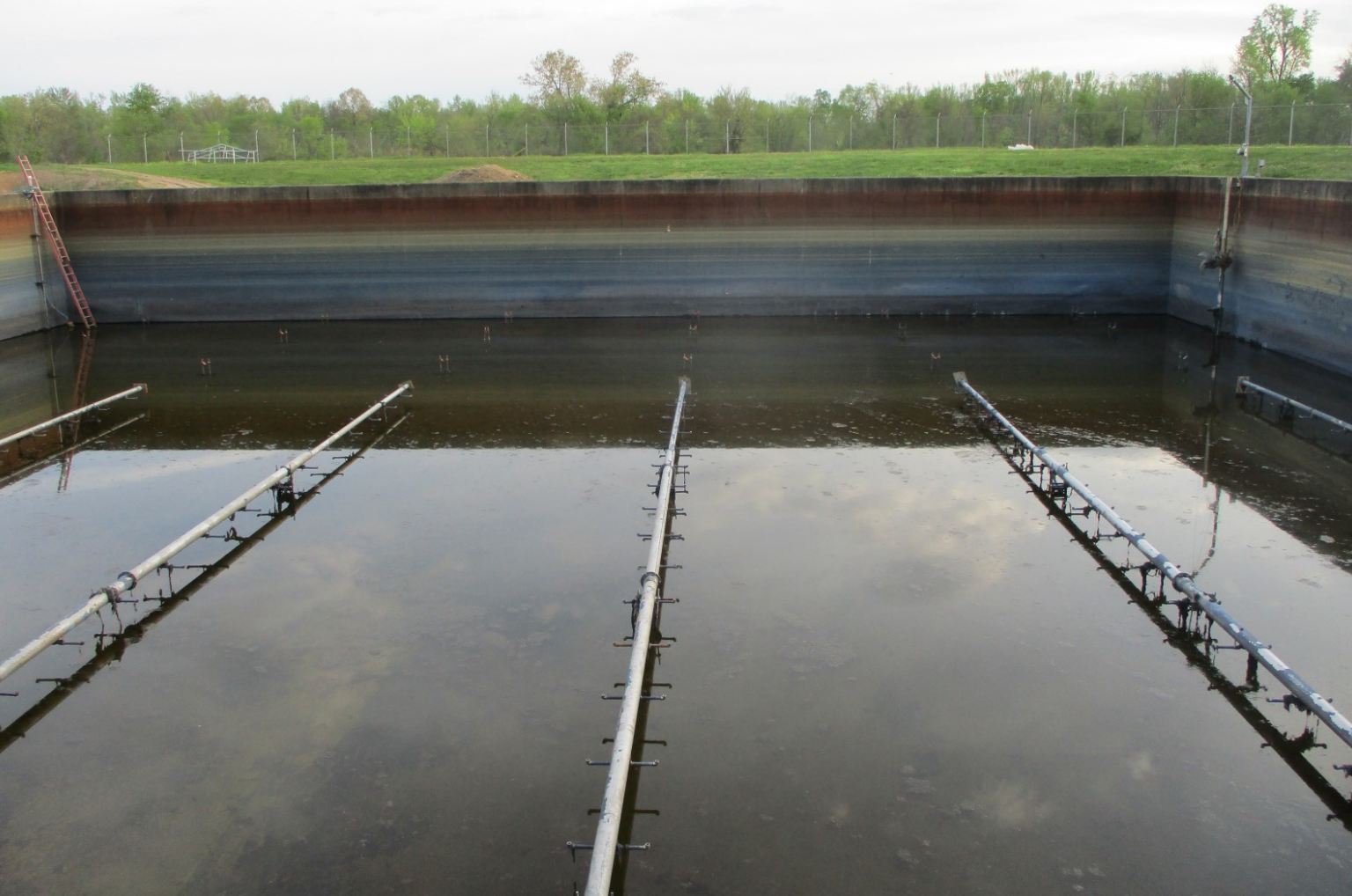
Sludge Holding Tank No. 2 - Photo 2
