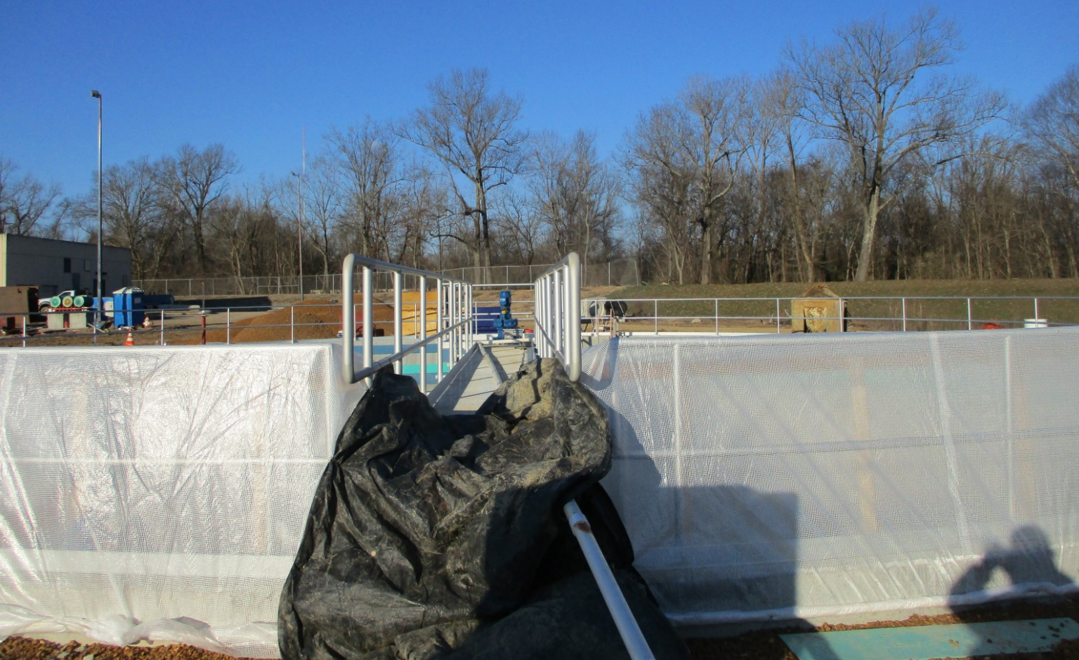
Clarifier No. 6 - Photo 1
