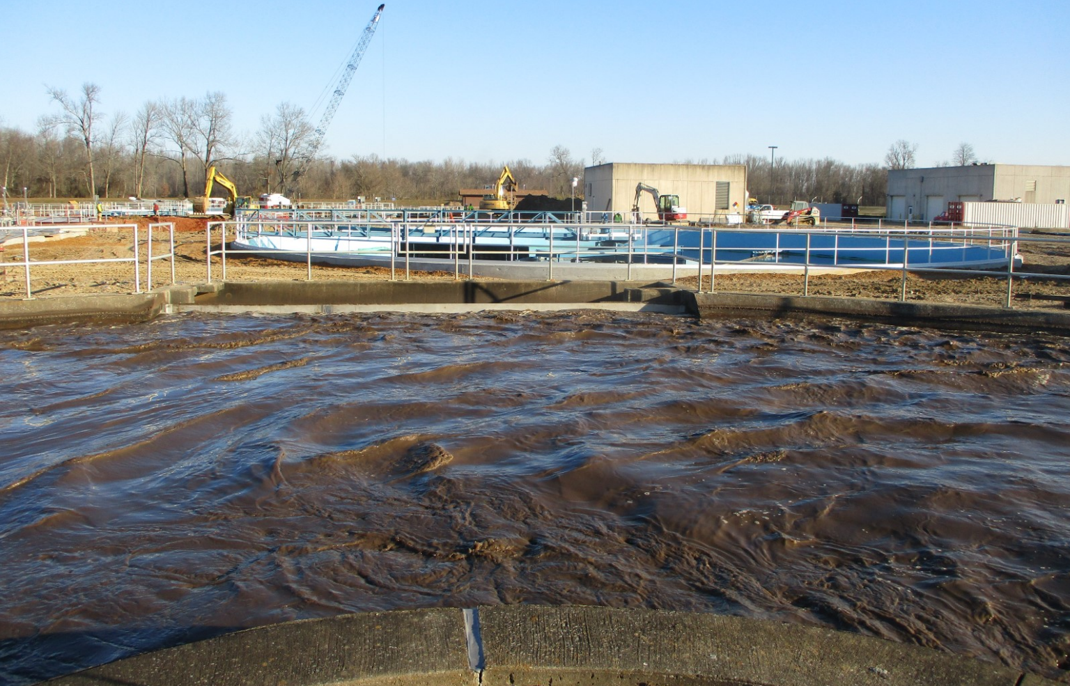
Oxidation Ditch No. 2 - Photo 4
