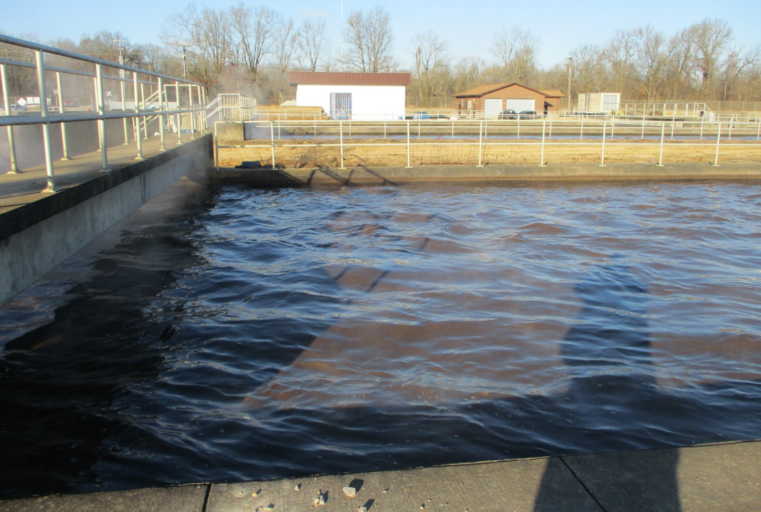
Oxidation Ditch No. 2 - Photo 2
