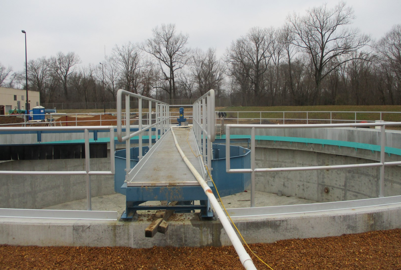
Clarifier No. 6 - Photo 1
